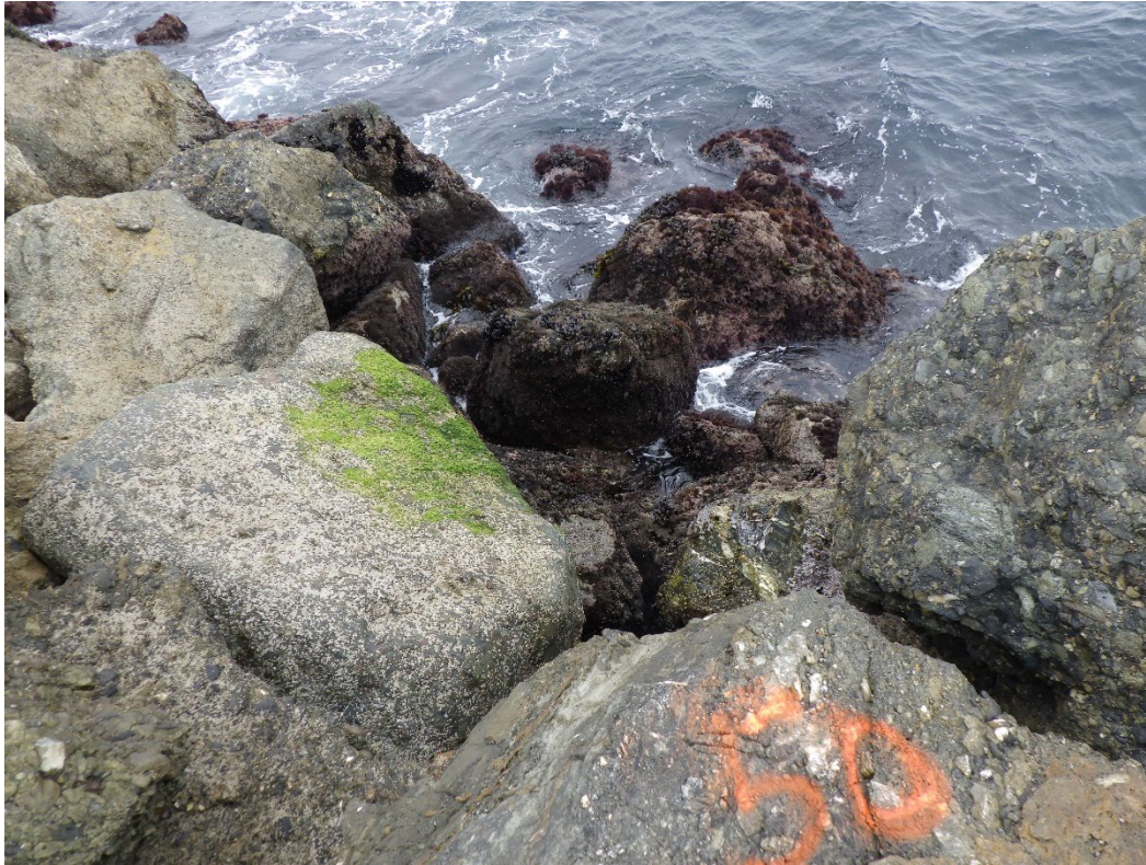
Figure 35: Near breach, failure of seaward slope at Station 50+00.
