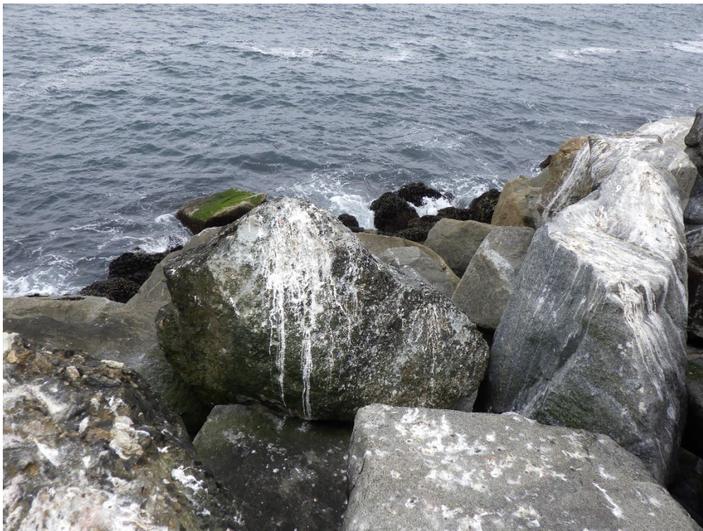
Figure 18: Loss of interlock and separation from seaward shoulder, Station 29+75.
