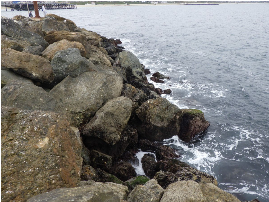
Figure 36: Failure of seaward slope, underlayer visible and several perched stones, Station 50+85.
