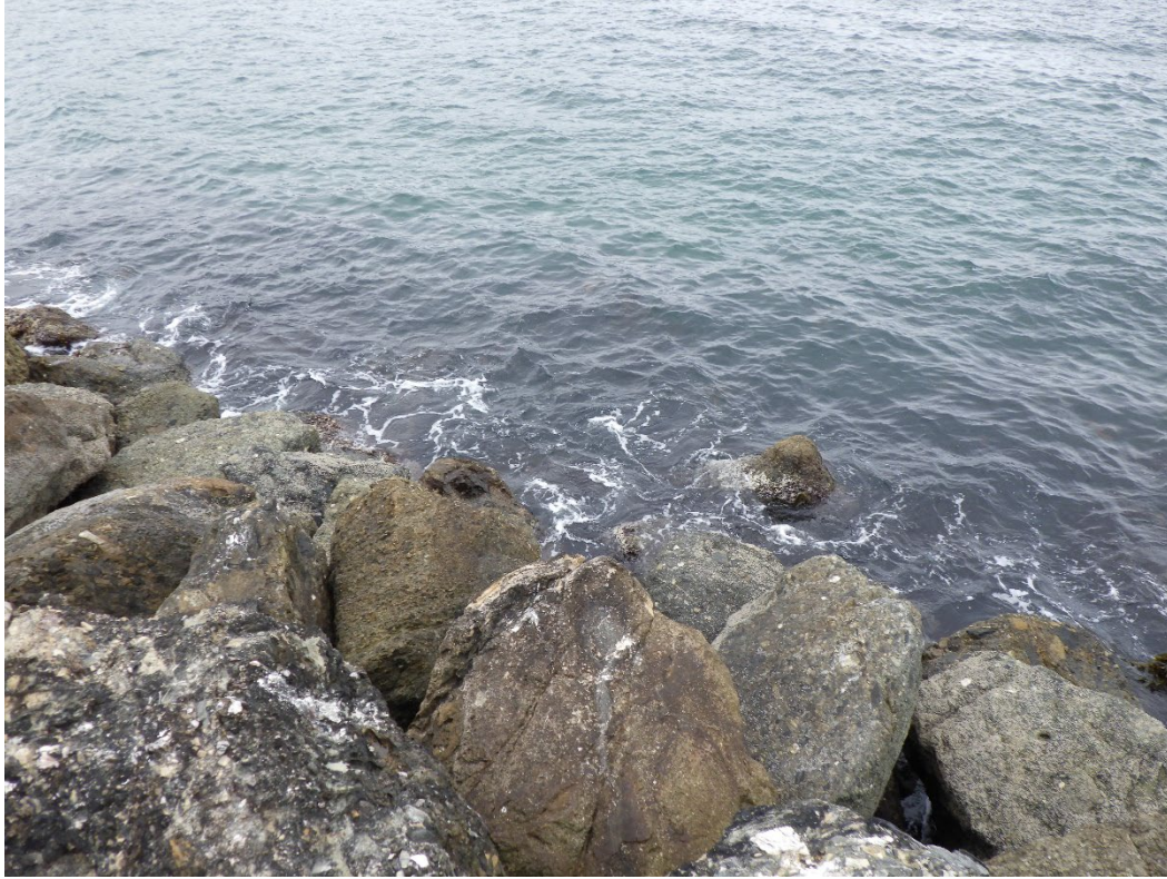
Figure 43: Displaced stone at waterline, loss of interlock on seaward slope, station 3+60
