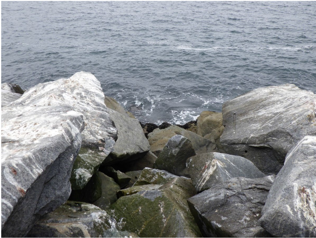
Figure 20: Loss of armor stone on seaward slope, upturned stone on seaward shoulder, Station 30+25.
