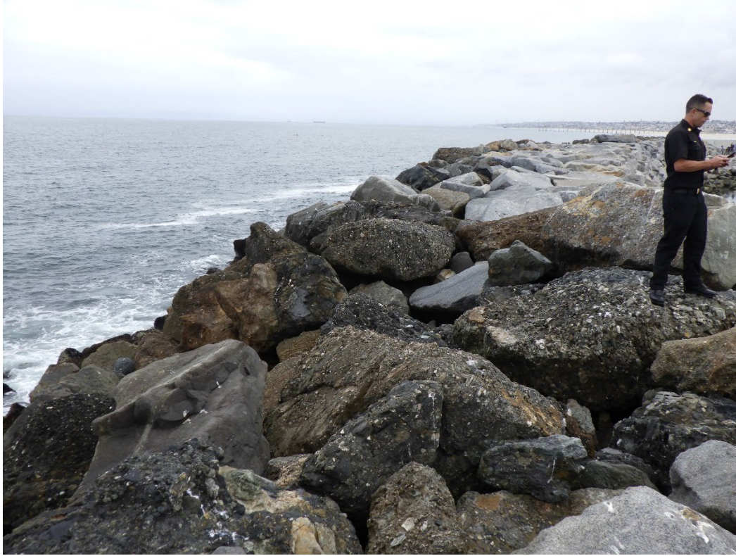
Figure 9: Loss of crest elevation and oversteepened slope along seaward shoulder from 20+00.
