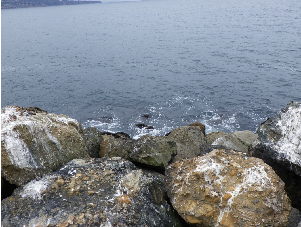
Figure 25: Oversteepened seaward slope at Station 36+20.
