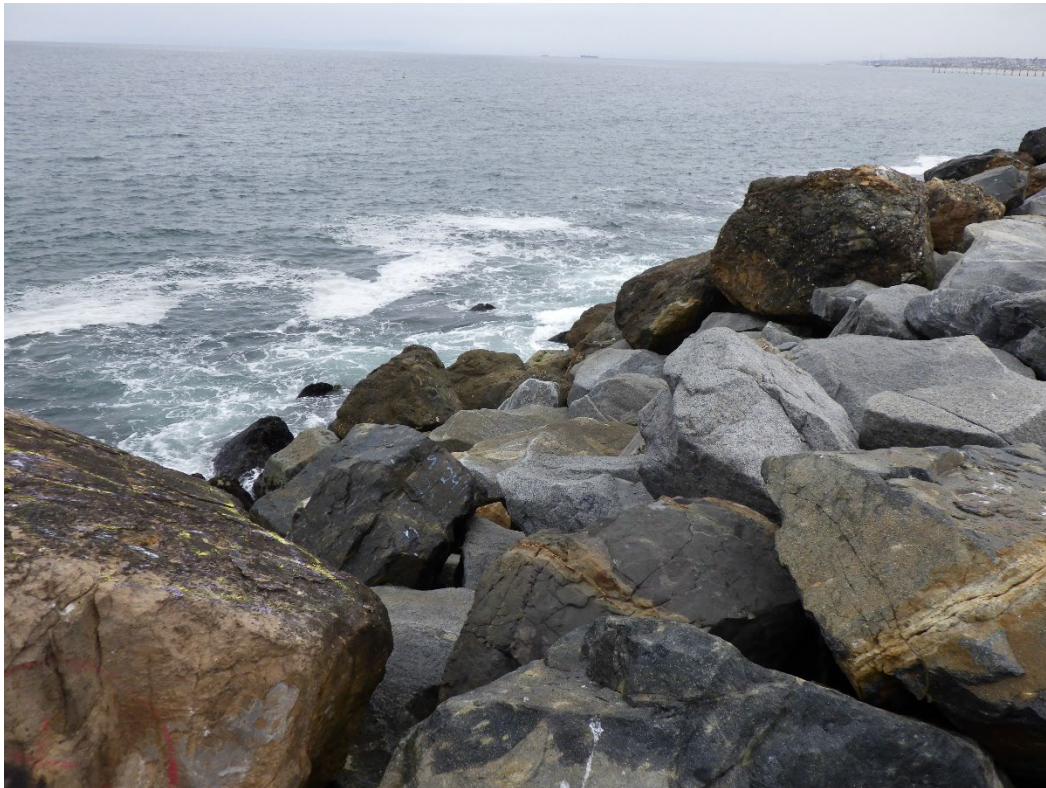
Figure 6: Missing stones on seaward slope, Station 18+20.
