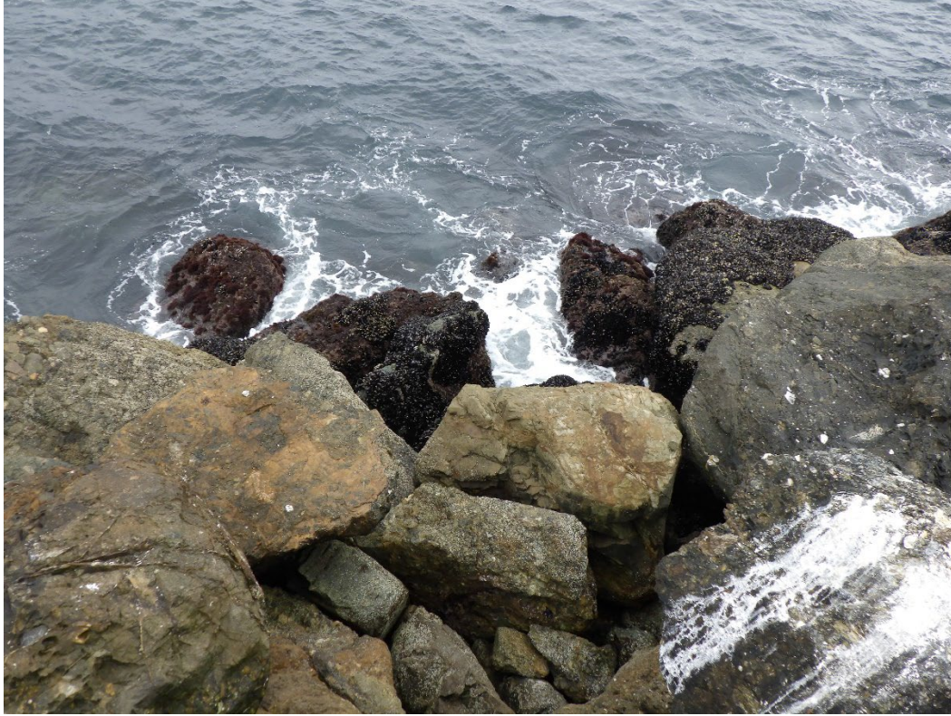
Figure 33: Missing armor stone at waterline and on seaward slope, loss of interlock, Station 48+00.0.
