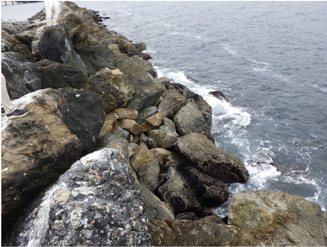
Figure 34: Failure of seaward slope between stations 48+50 and 49+00.
