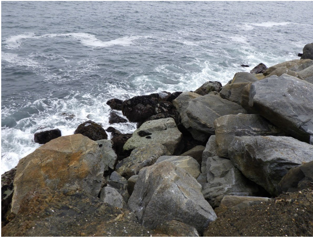
Figure 10: Missing stones at waterline causing instability and loss of interlock up slope, Station 20+60.
