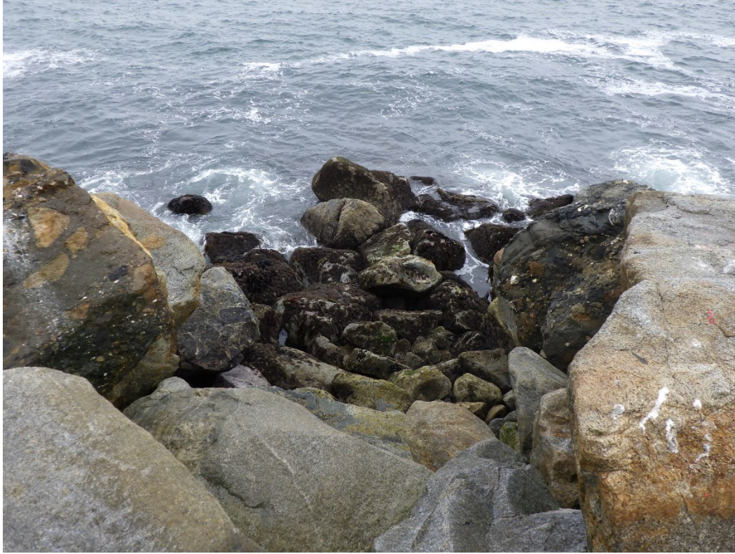
Figure 11: Loss of armor stone from seaward slope, Station 21+05.
