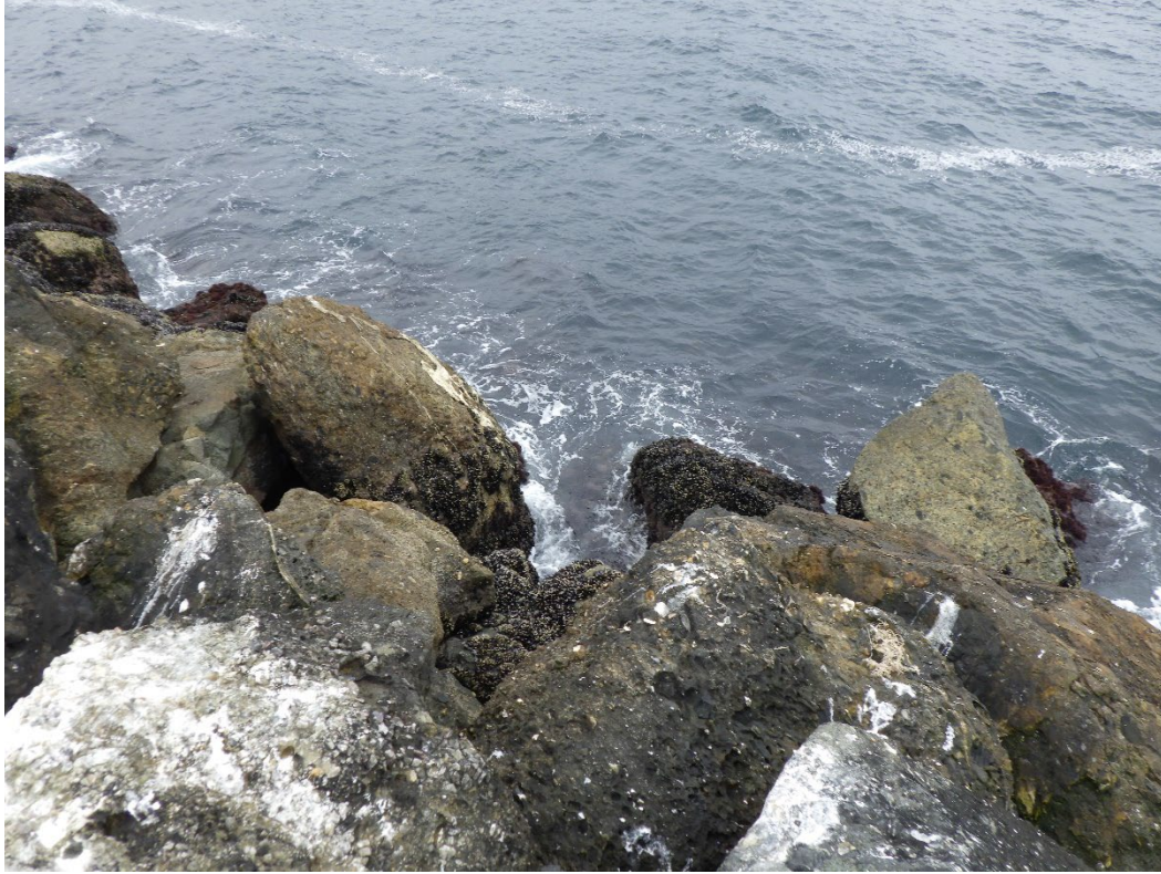
Figure 31: Upturned armor stones and loss of interlock, loss of armor stone on seaward slope, Station 47+00.
