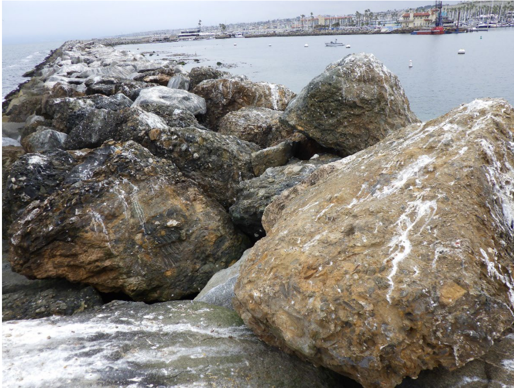
Figure 23: Two upturned stones on structure crest, Station 33+30.
