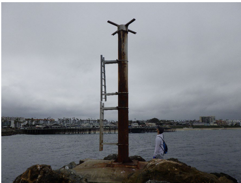
Figure 38: North breakwater navigation aid missing.
