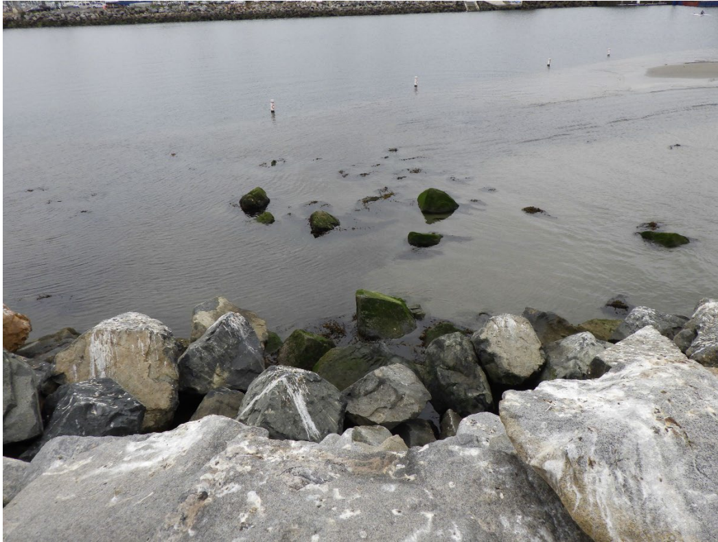
Figure 13: Ejected stones and damage to harbor side bench, Station 23+15.
