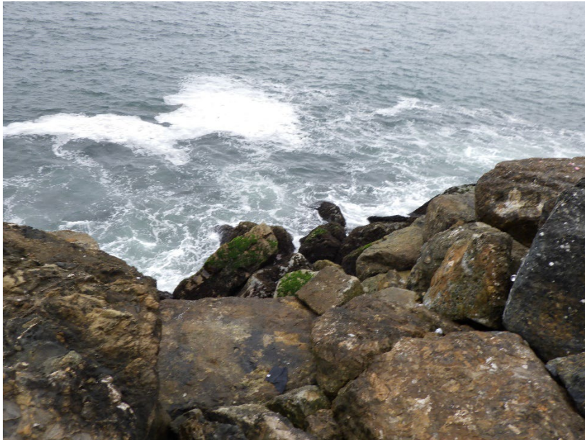
Figure 2: Condition 3 damage area, loss of armor stone on seaward slope at approx. station 15+75.
