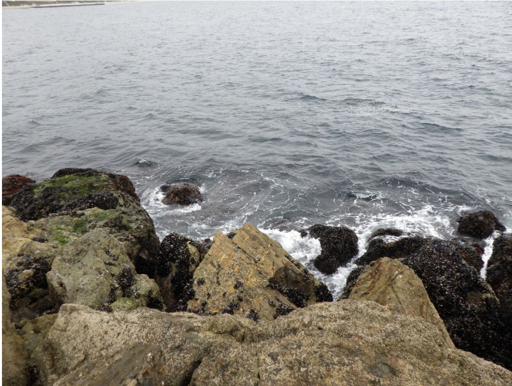
Figure 37: Separated armor stone at waterline, seaward radial of head section.
