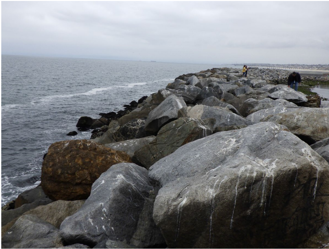
Figure 12: Loss of interlock on seaward slope, Station 22+00 looking north.
