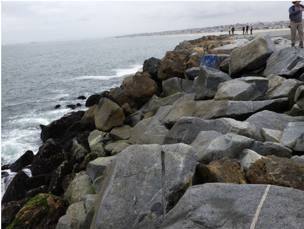
Figure 4: Loss of interlock and armor stone on seaward slope 17+50
