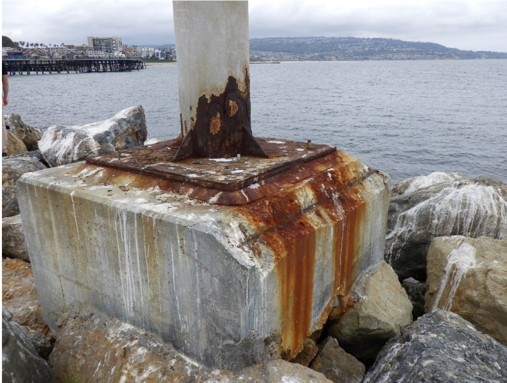
Figure 47: Rust at bottom of navigation aid pedestal and spalling on concrete base.
