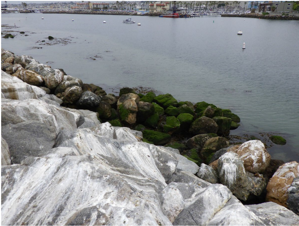
Figure 22: Separation of stones on harbor side bench at Station 32+00.
