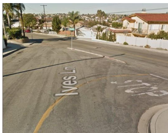
Photo 2 – Street view of existing configuration
