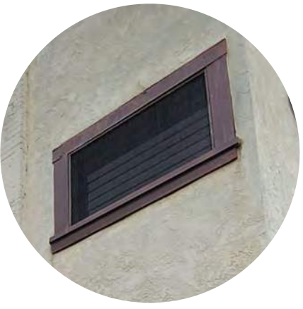
D: Replace non-original windows with custom wood windows to match original windows & existing opening size.
