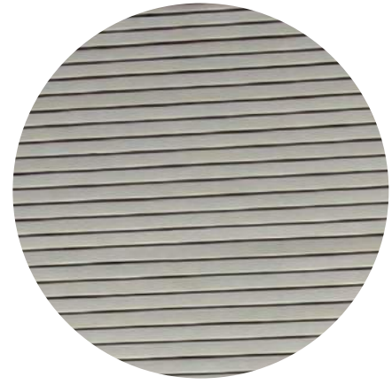
B: Clean & paint horizontal siding & parapet cap
