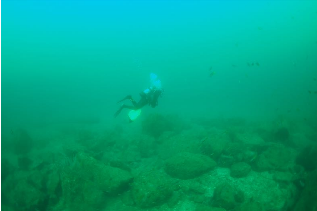
Figure 3. Current photo of the Redondo Beach Artificial Reef. Levelled pile of quarry rock.
