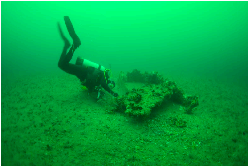
Figure 8. Current photo of the Redondo Beach Artificial Reef. Concrete dock floats were turned into habitat by cutting windows into the cement cube. Floats have broken up into flat plates, this float is in above average condition.
