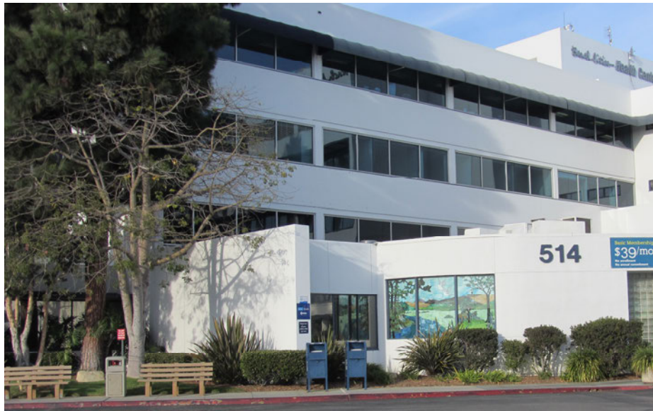
Figure 2 - View of South Side of North Tower
