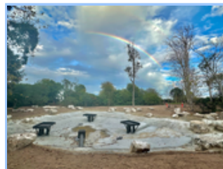
Wilderness Park Pond Construction
