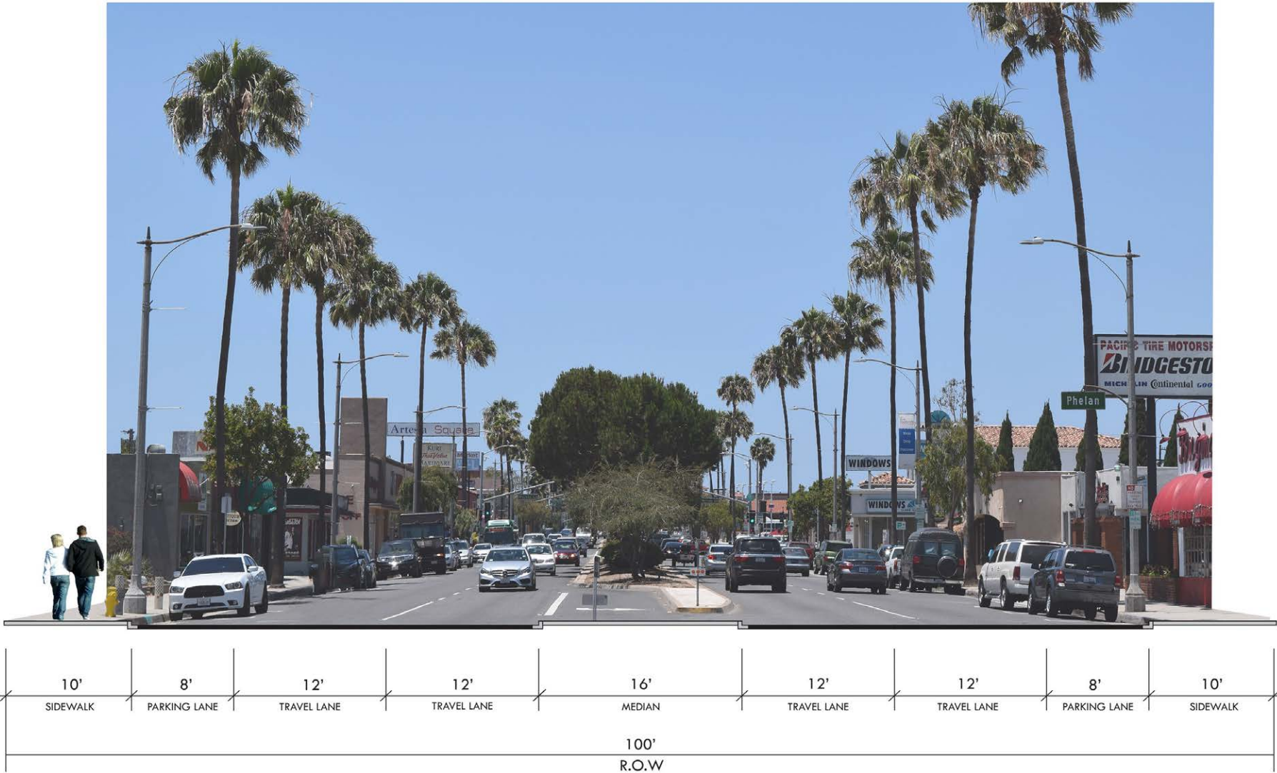
Figure 4.4: Artesia Boulevard Existing Configuration
