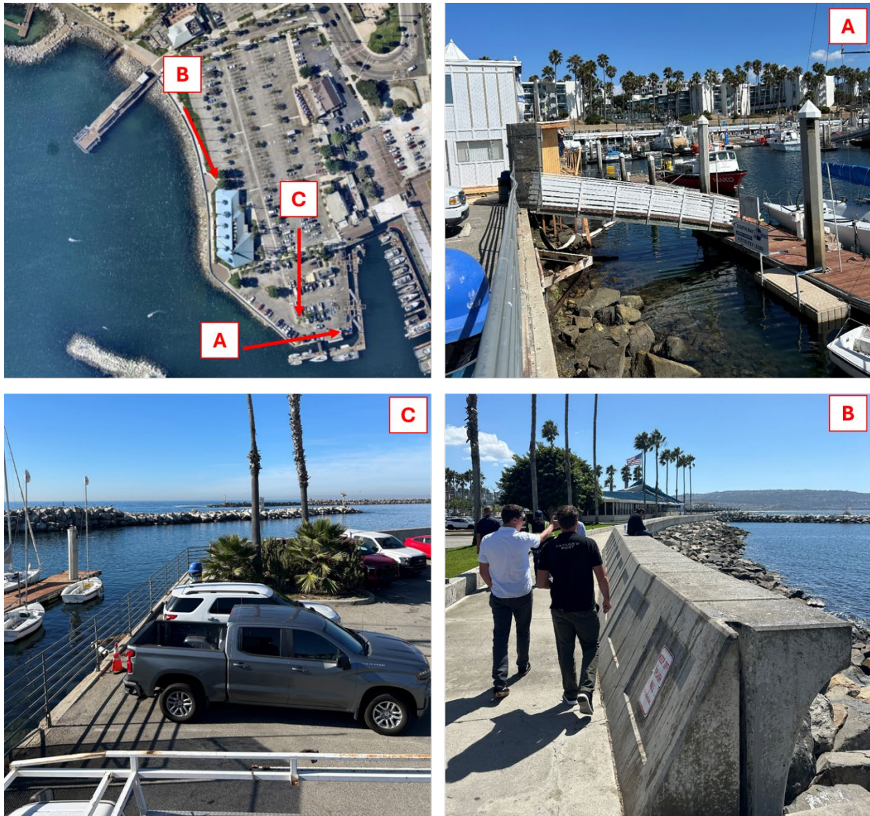
Figure 21. Project site seawall (A and B) and bulkhead (C) from different views (photos taken in fall of 2024)
