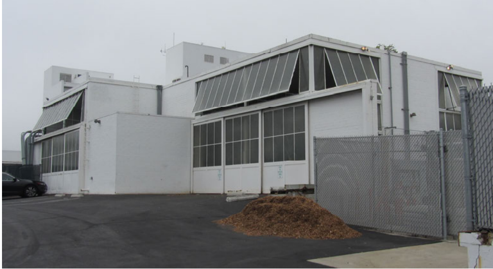
Figure 3 -View of Central Plant
