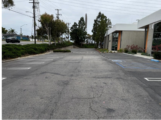
Photo 2. Side (south) parking area near 2601 Manhattan Beach Blvd.
