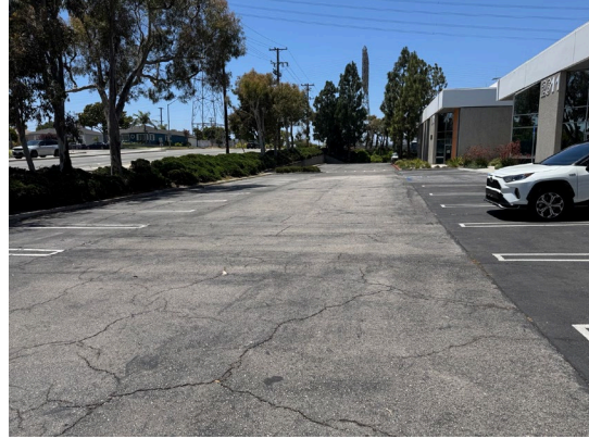
Photo 2. Parking along the side (south) frontage area near 2601 Manhattan Beach Blvd.
