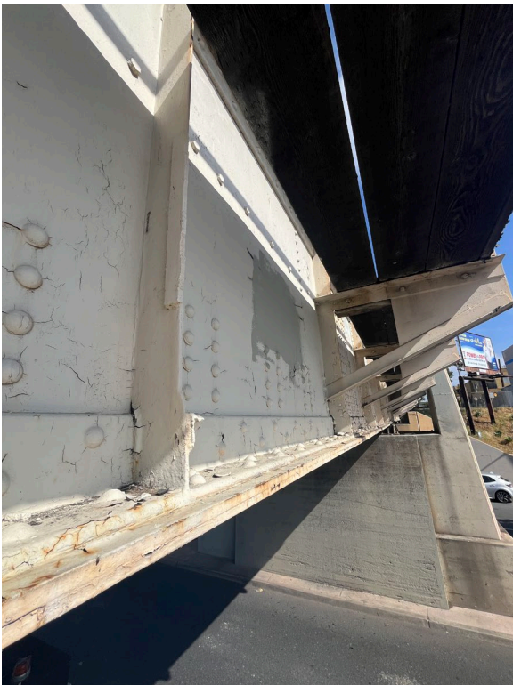
(above) Lead-based white wood paint, beige handrail paint, multicolor metal support paint, beam paint, and lead-containing concrete paint.
