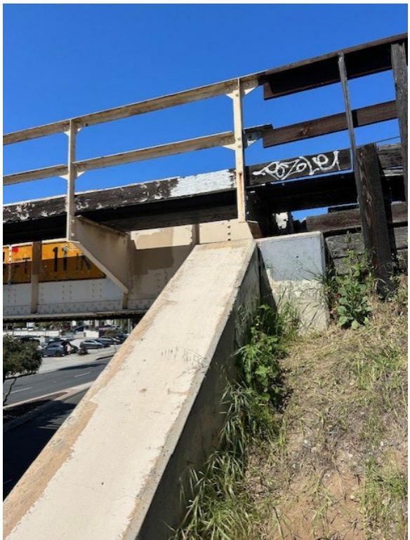
(above) Lead-based white wood paint, beige handrail paint, multicolor metal support paint, beam paint, and lead-containing concrete paint.
