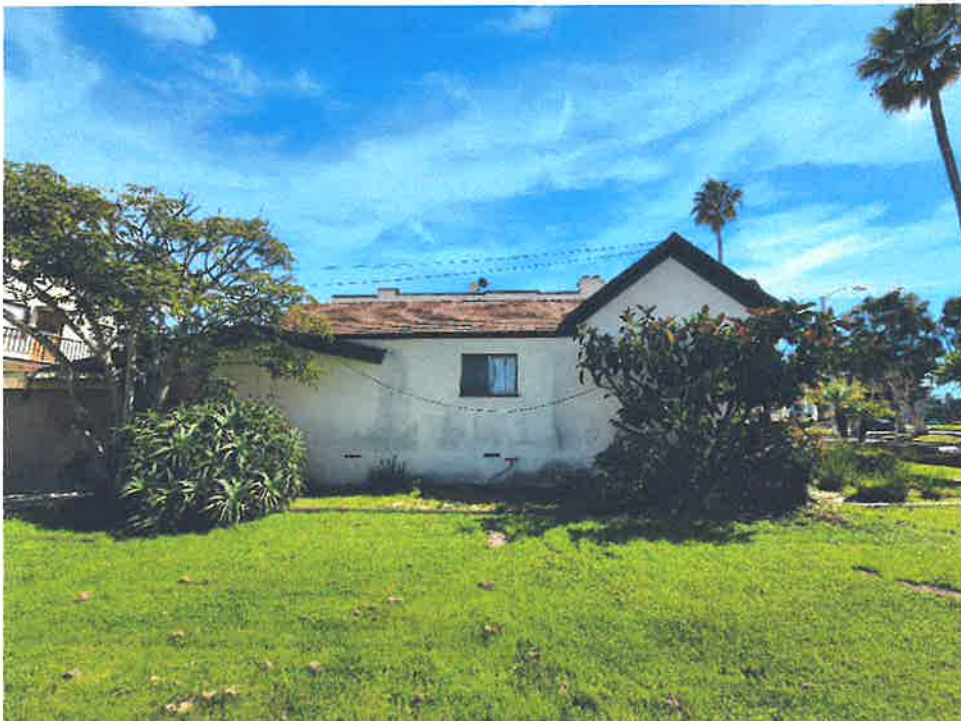
North elevation (from adjacent vacant lot)
