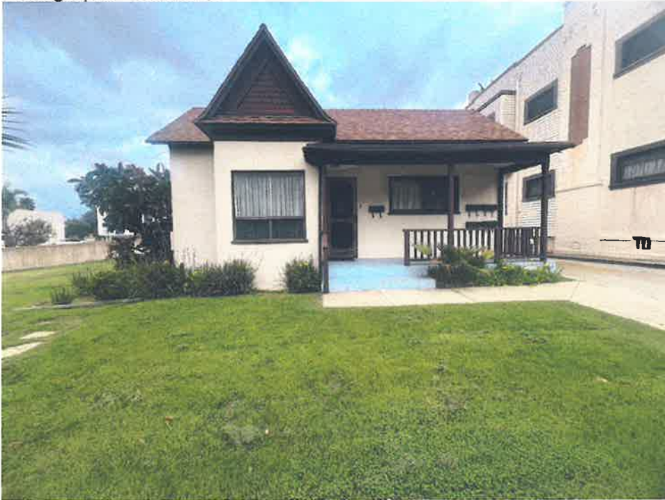
West elevation front façade)
