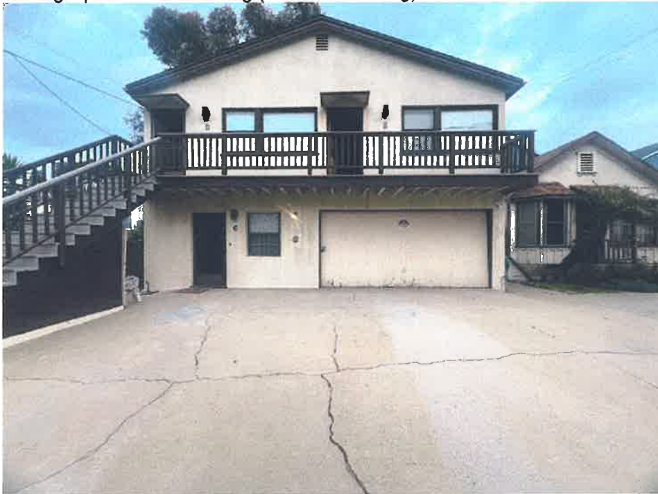
West elevation (front façade)
