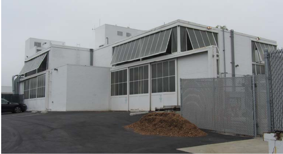
Figure 3 -View of Central Plant
