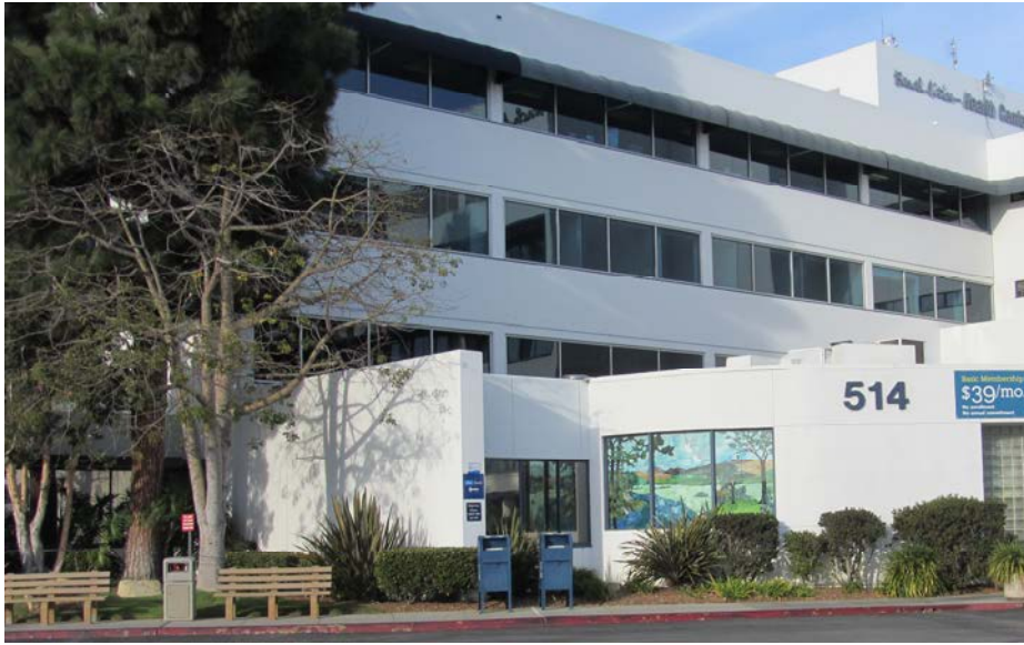
Figure 2 - View of South Side of North Tower
