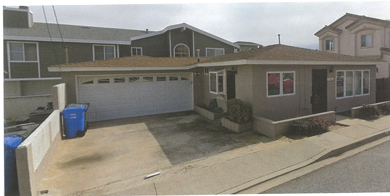
EXISTING FRONT VIEW/GREEN LANE
