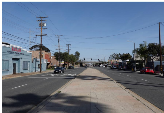
Looking East on Manhattan Beach Blvd.
