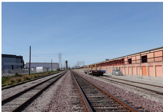
Looking North from the ROW north of Inglewood.
