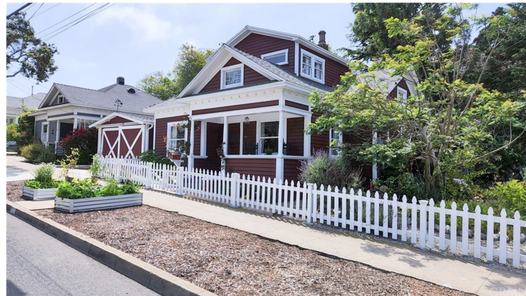
EXISTING NORTHWEST VIEW
