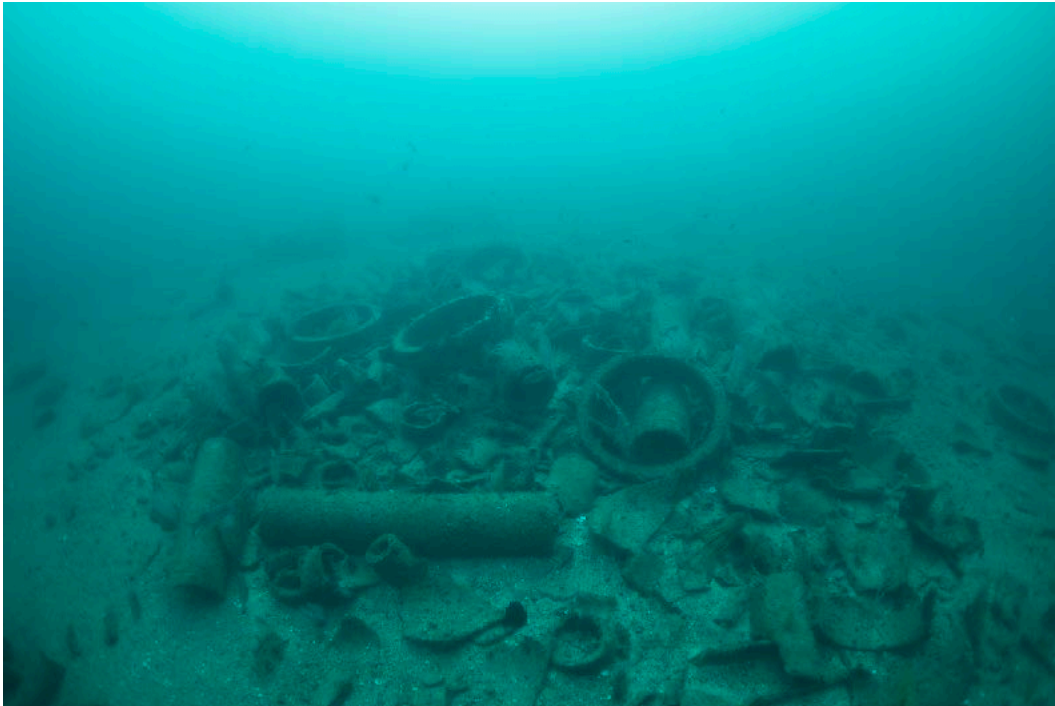
Figure 5. Current photo of the Redondo Beach Artificial Reef. Crumbled cement pipe.
