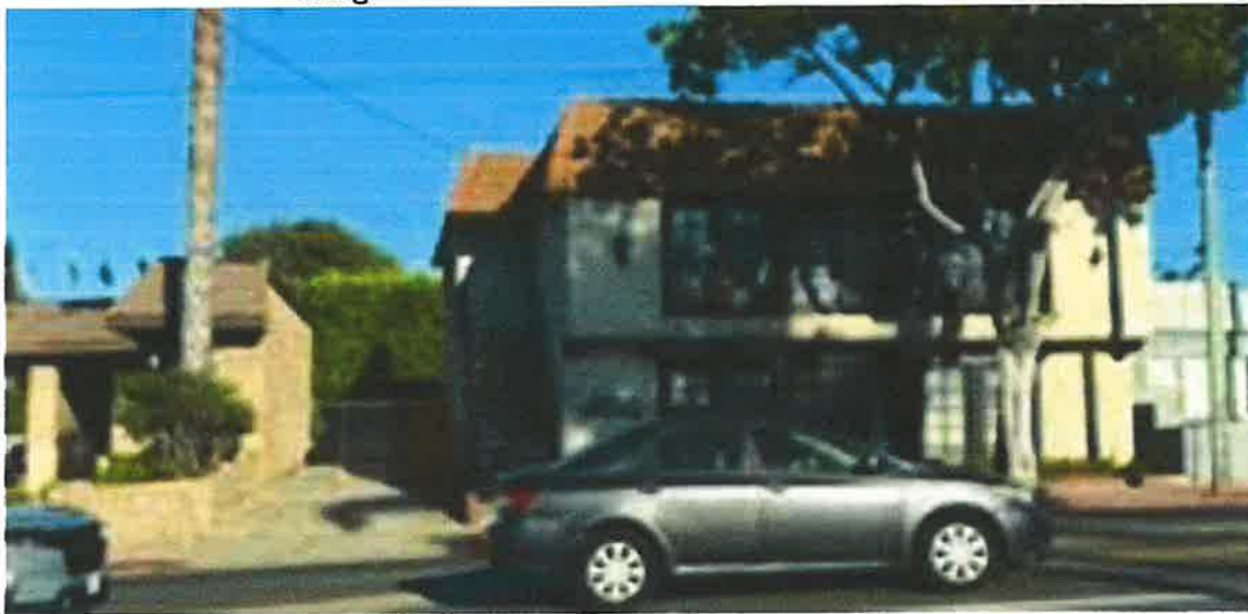
12' Driveway to Rear Parking Lot Commercial Office Building next to car wash.
