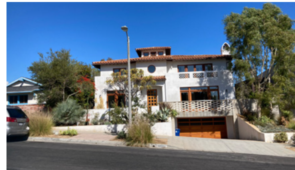
Example of side-sloping lot with a basement garage on the downslope side.
