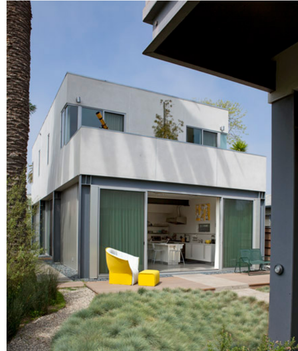
Example of modular construction with second-story setback on a 40-foot wide lot in Venice, CA. (Source: OMD Corp. A Jennifer Siegal company)
