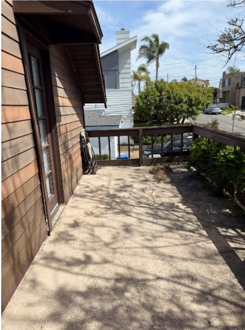
Figure 6. Second-story deck, facing southeast.
