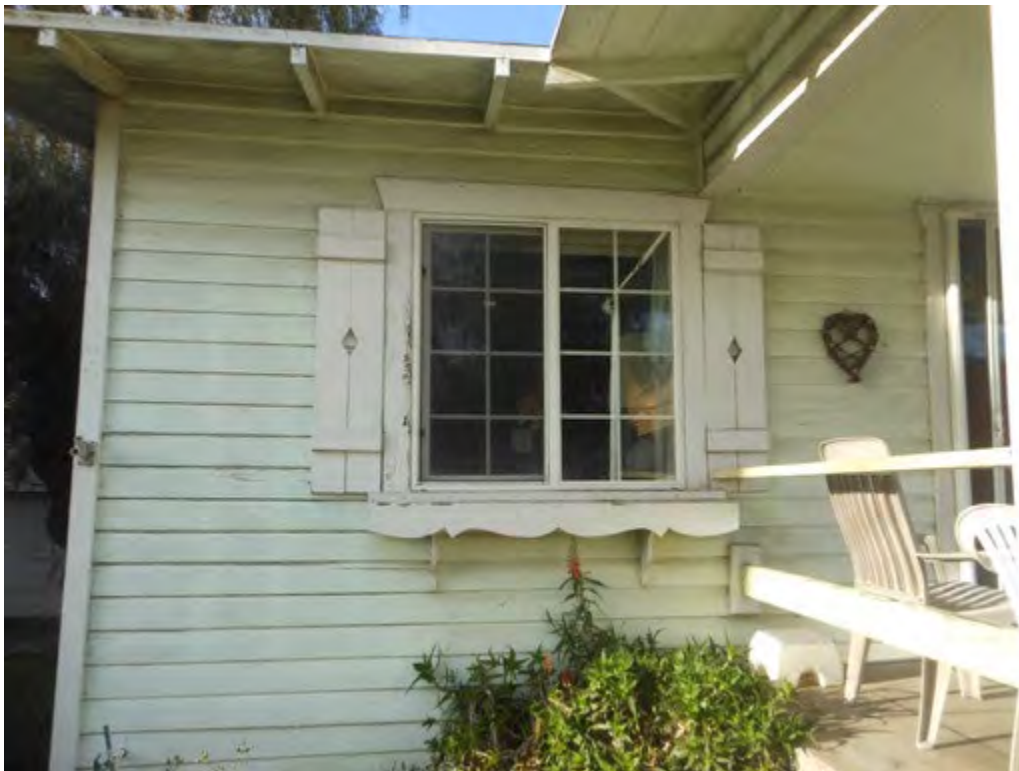
44. Window detail on south (front) elevation
