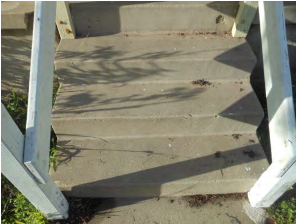
47. Stair and porch railing detail on south (front) elevation
