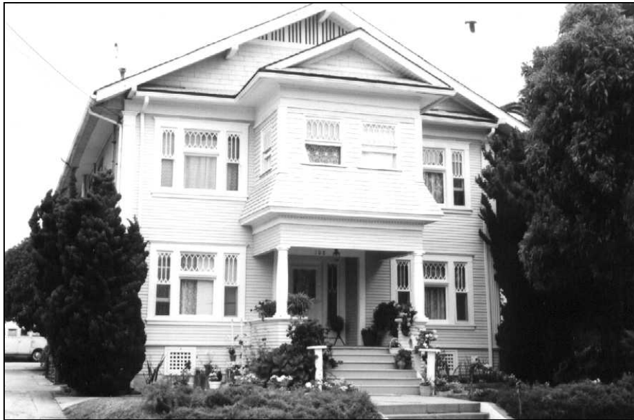
Dorrington Apartments, Local Landmark No. 18 108 North Broadway
