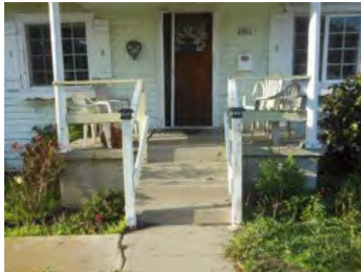
Stair to porch and entry door on south elevation
