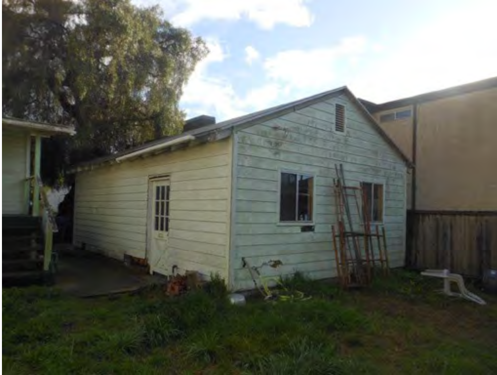
39. East (side) and north (rear) elevation of garage
