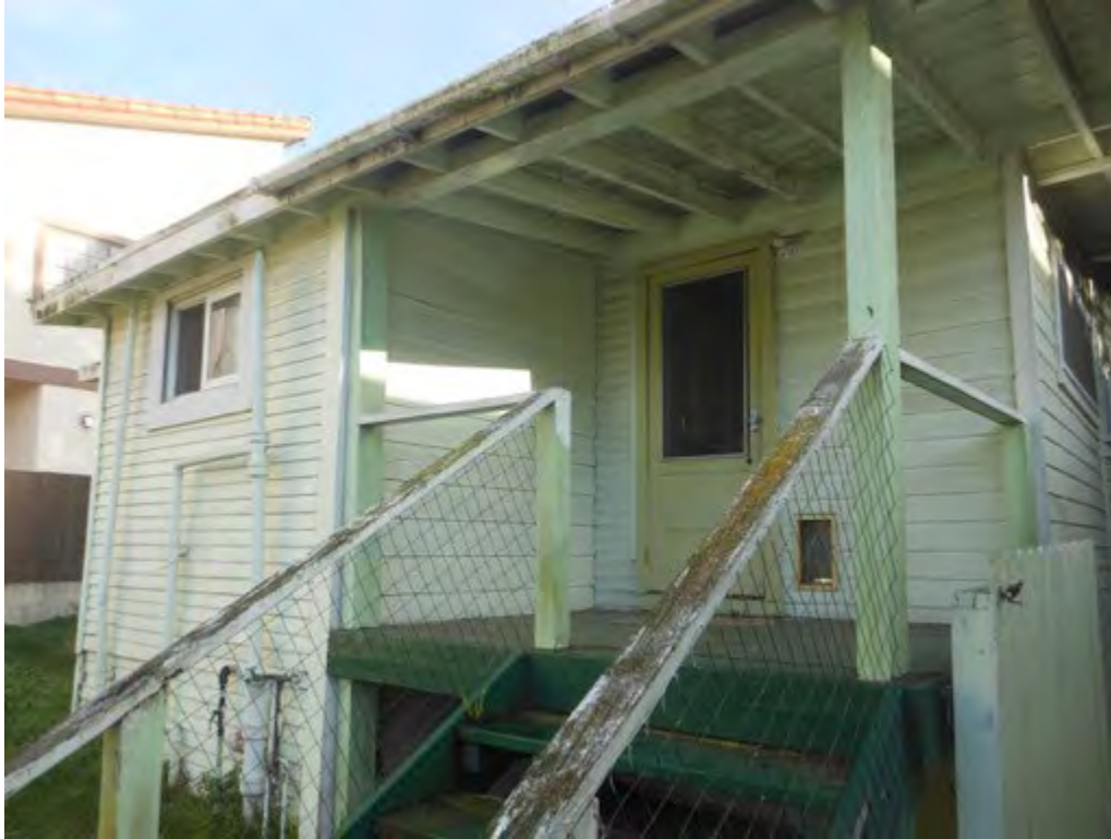
37. Stair and entrance on north (rear) elevation
