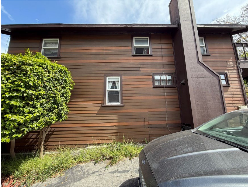
Figure 7. Northwestern elevation, facing southeast.
