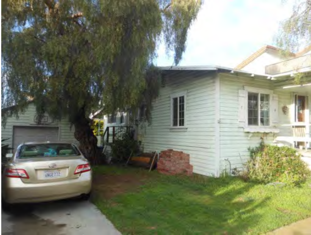
31. Part of south (front) elevation and west (side) elevation
