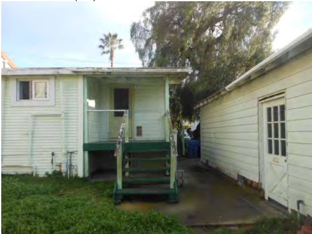
38. West half of north (rear) elevation and east elevation of garage
