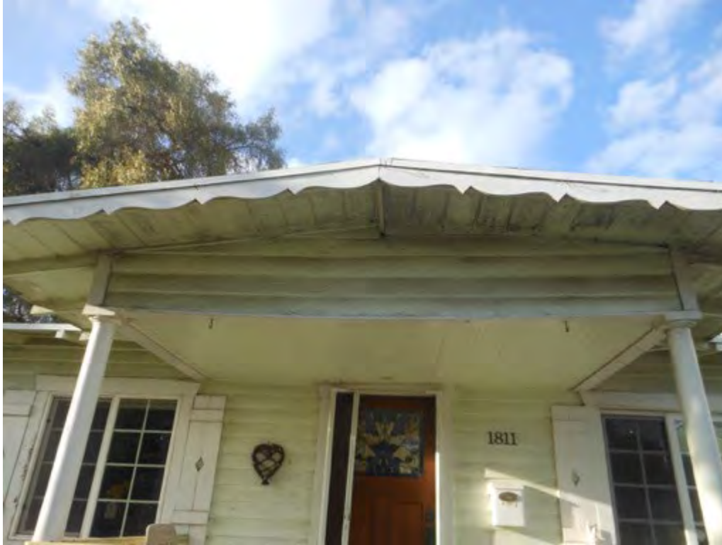
43. Roof over porch
