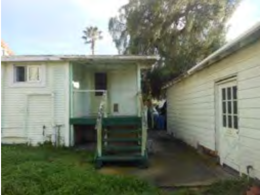
West half of north (rear) elevation and east elevation of garage
