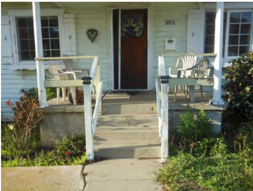
46. Stair to porch and entry door on south (front) elevation
