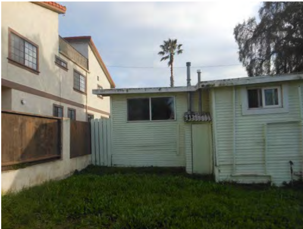
36. East half of north (rear) elevation
