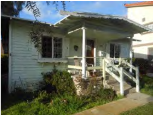
Stair and porch on south (front) elevation
