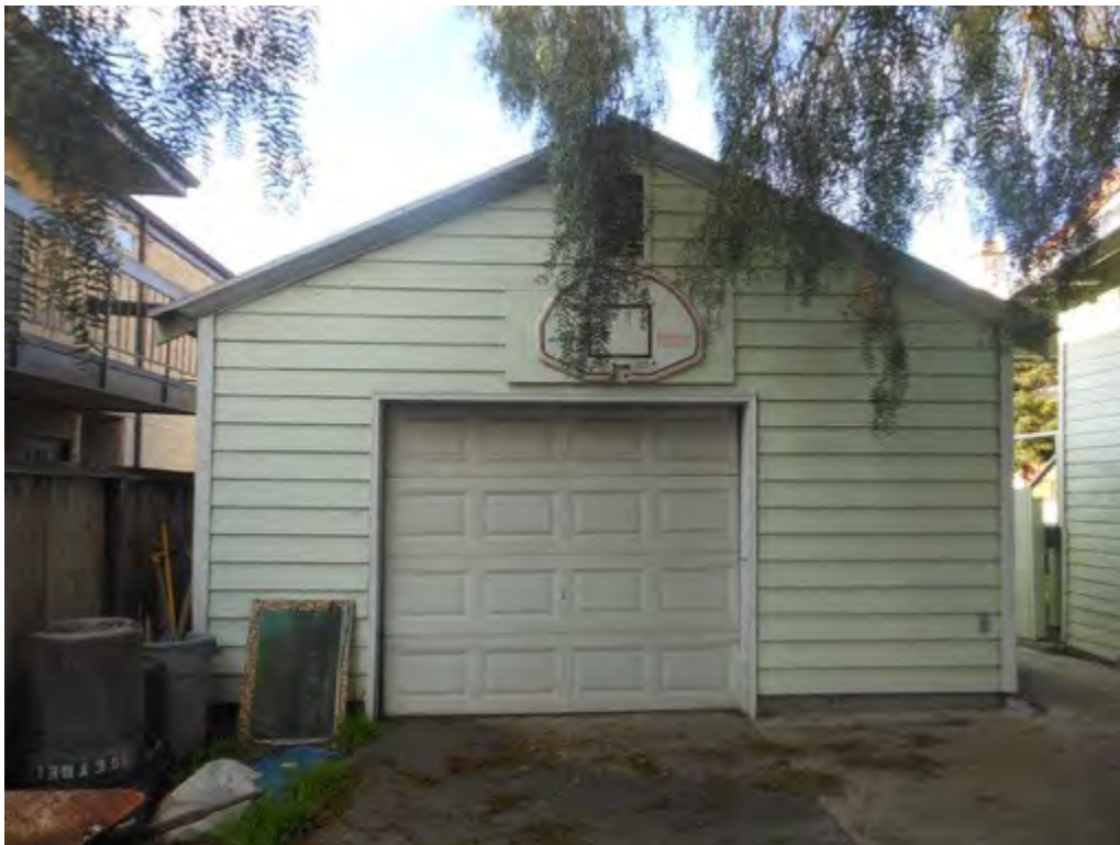
40. South (front) elevation of garage
