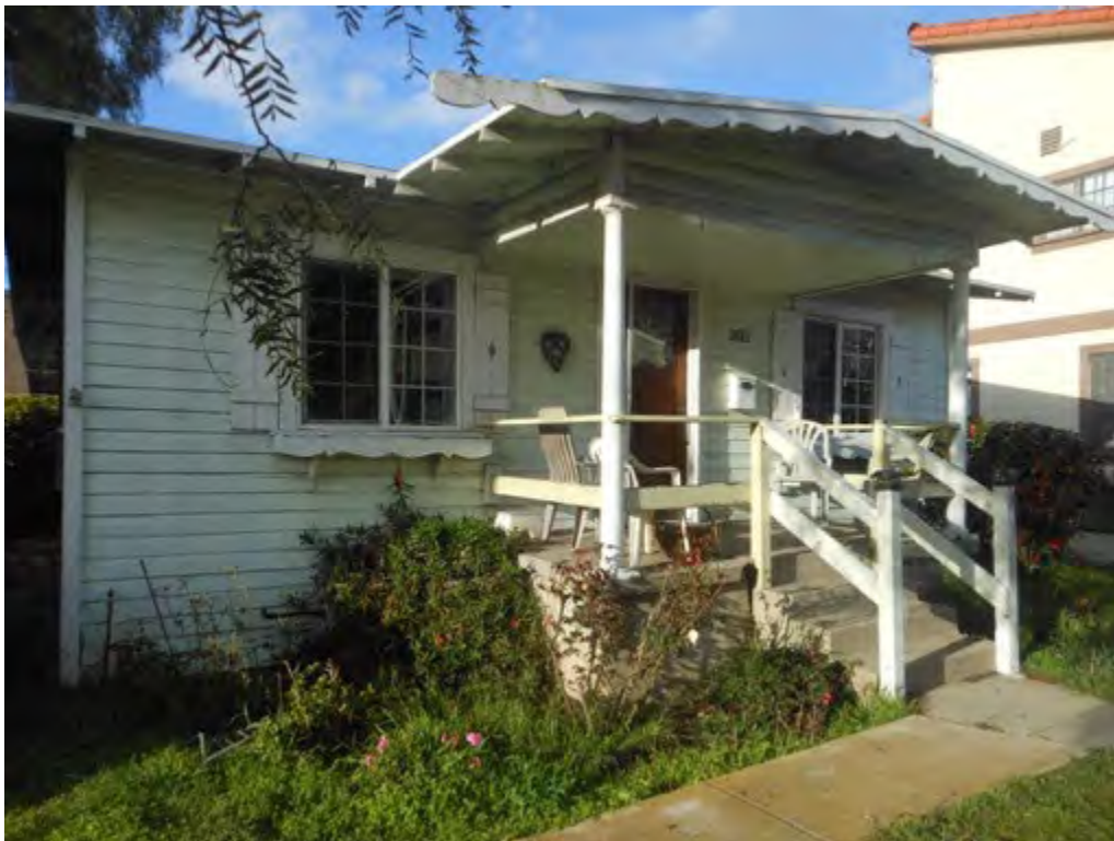
42. Stair and porch on south (front) elevation
