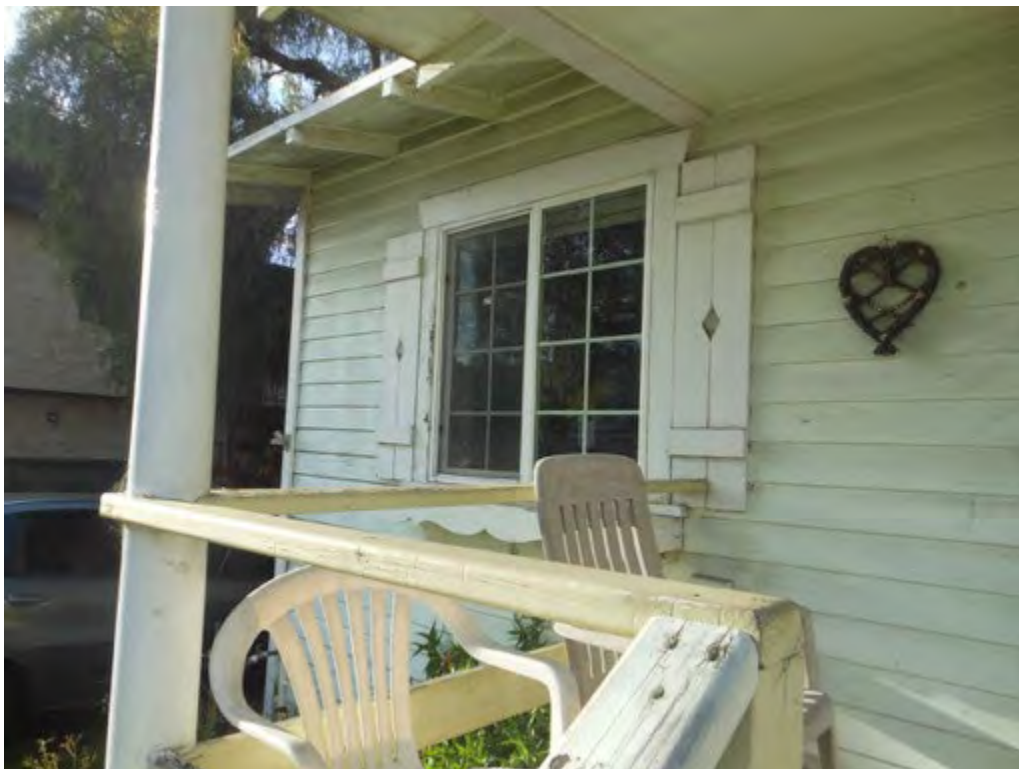
48. Porch and railing and window detail on south (front) elevation
