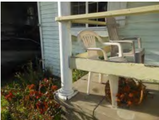
Porch detail on south (front) elevation
