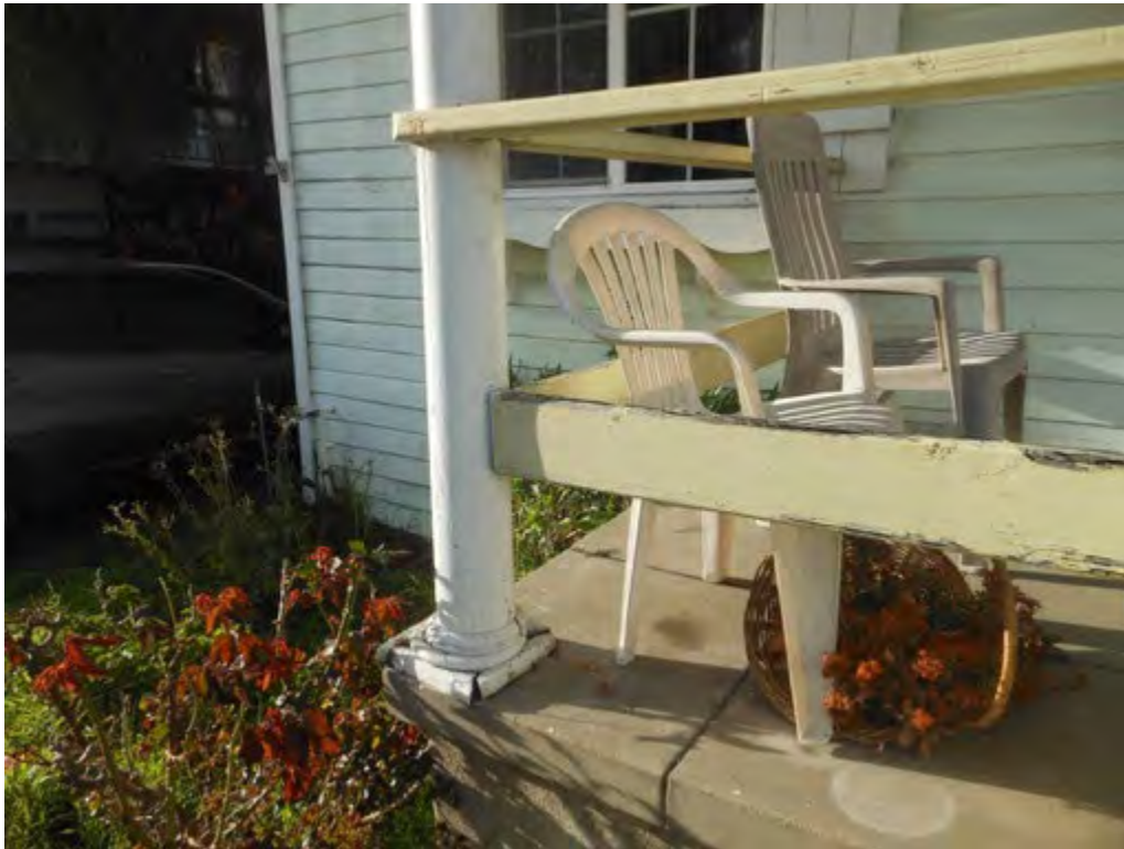
49. Porch detail on south (front) elevation
