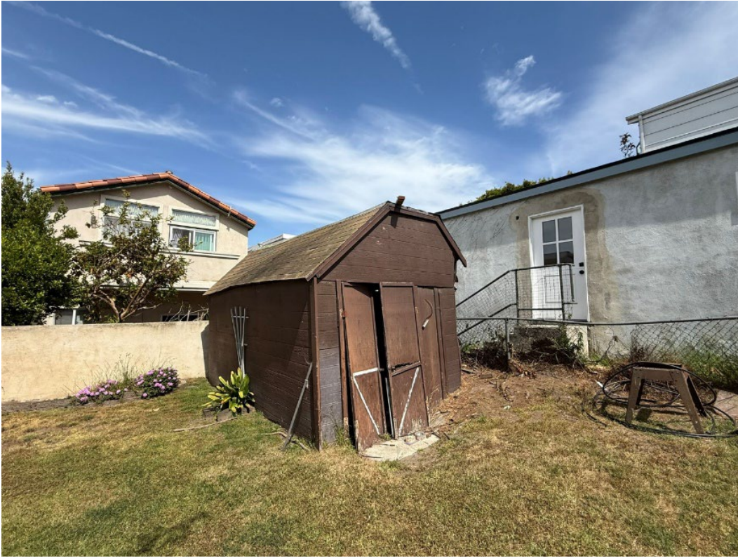
Figure 12. Detached shed, facing east.
