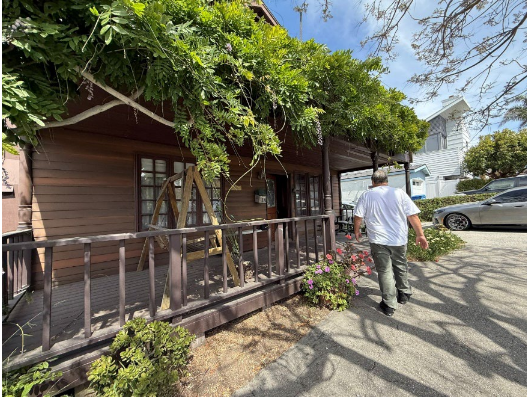
Figure 5. Porch on primary (southwestern) elevation, facing east.
