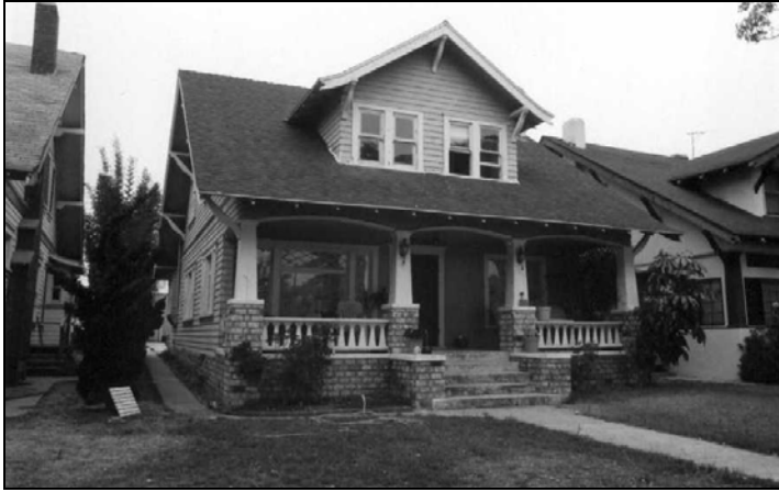
Gephart House, City Landmark No. 19 519 South Catalina Avenue
