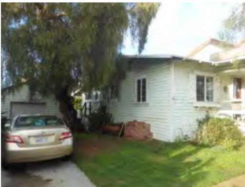
Part of south (front) elevation and west (side) elevation
