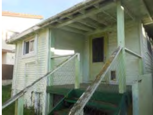
Stair and entrance on north (rear) elevation
