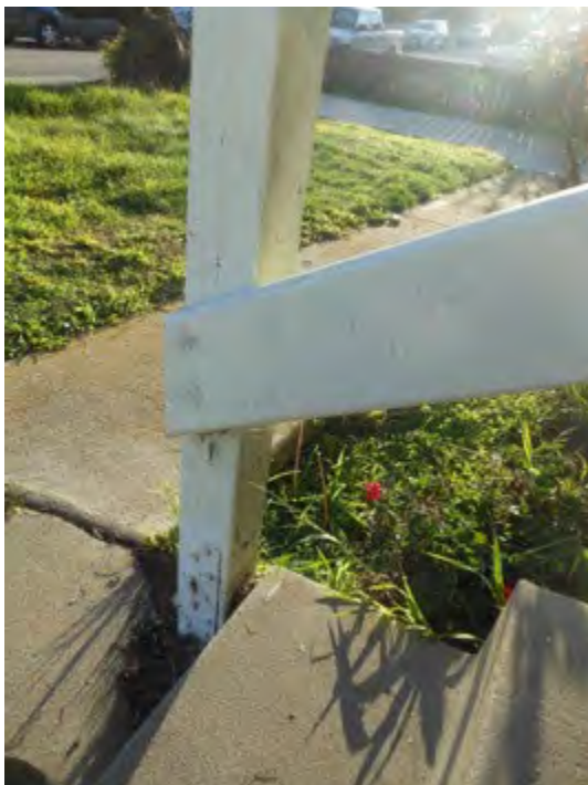
50. Railing detail on south (front) porch entry
