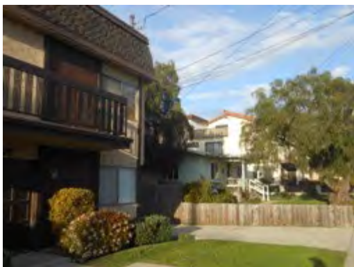
1809 Clark Lane, building to west of subject building
