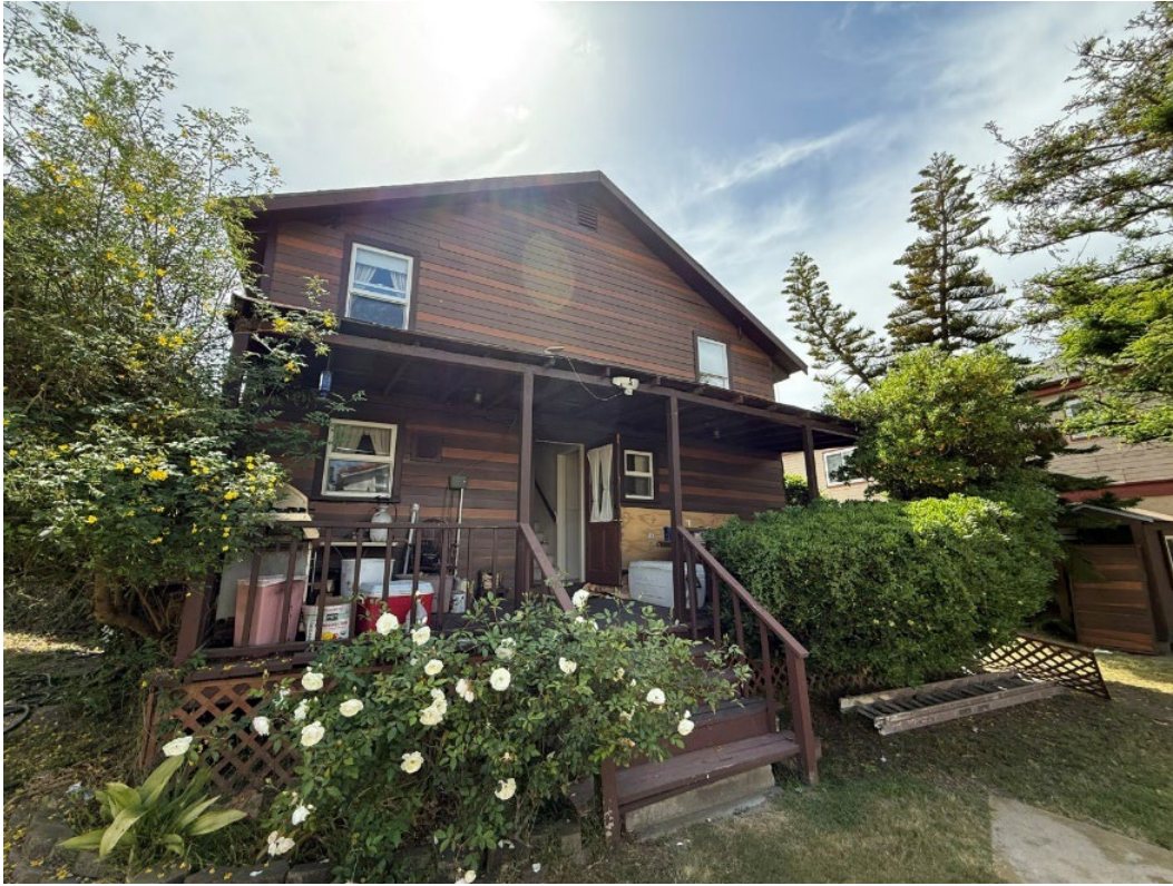
Figure 10. Rear elevation, exhibiting entrance and windows.
