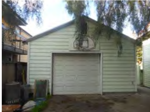
South (front) elevation of garage
