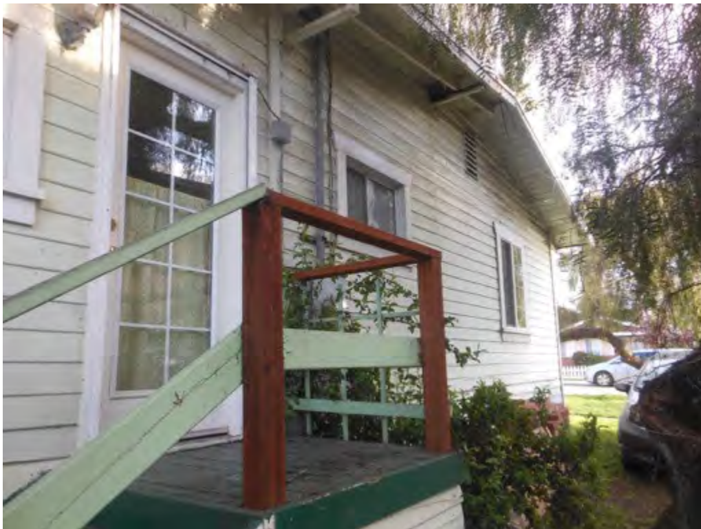
32. South half of west (side) elevation
