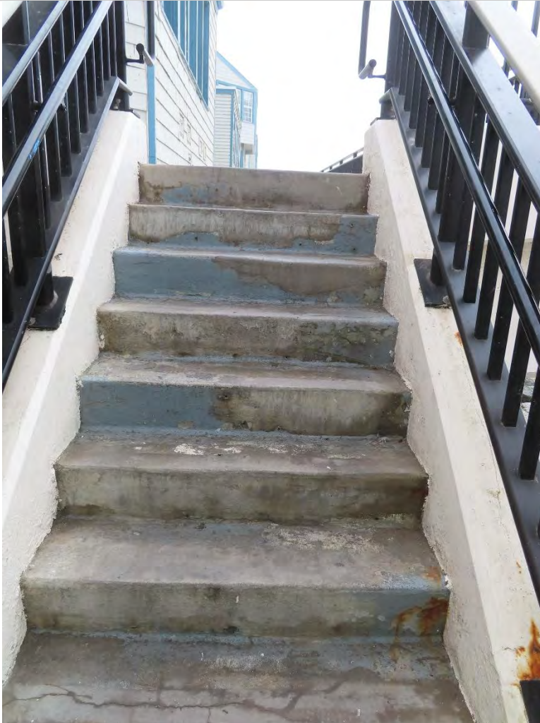
Photo 1.40- Typical stair coating worn off, (SH2-118)
