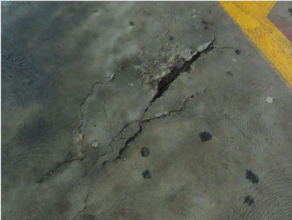
Photo 1.21- Concrete spalling at slabs, Pier level (SH2-10)
