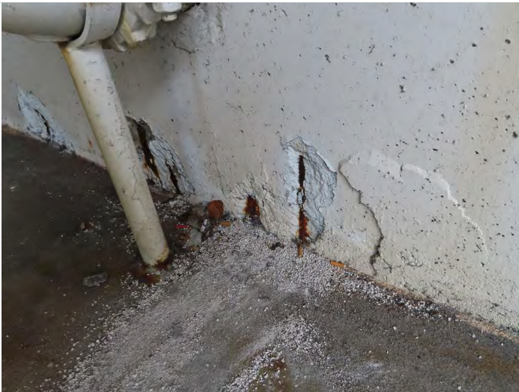
Photo 1.24- Exposed rebar on wall, Pier level (SH1-117)
