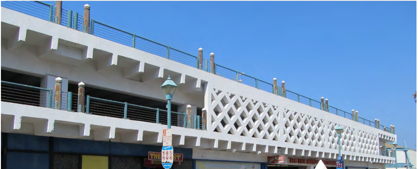
Photo 3.14- Truss chords at waffle shear wall at line Z.1 at the Village and Pier Level
