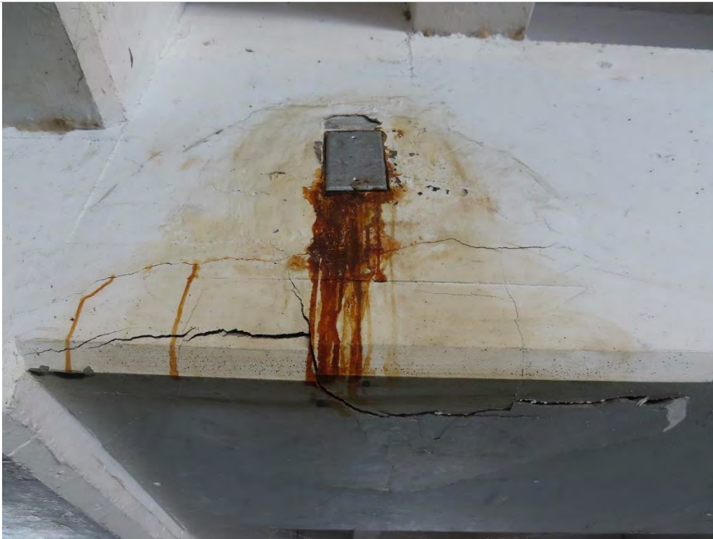
Photo 1.10- Concrete beam spall, Pier Level (SH3-201)
