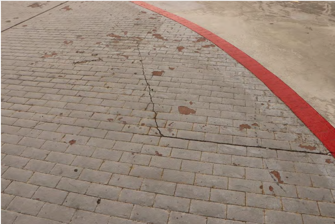
Photo 1.10- Typical spalled and cracked pavers, Village level (BA1-113)
