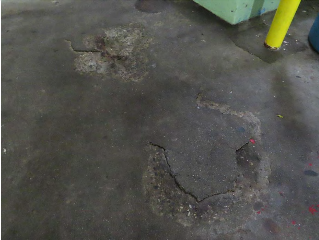
Photo 1.38- Isolated concrete column spalls, Basin level (SH1-241)
