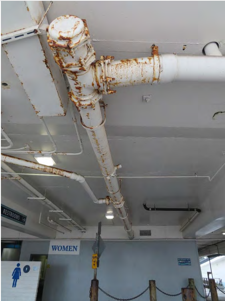
Photo 1.34- Corroded drainpipe, Pier level (MM1-33)
