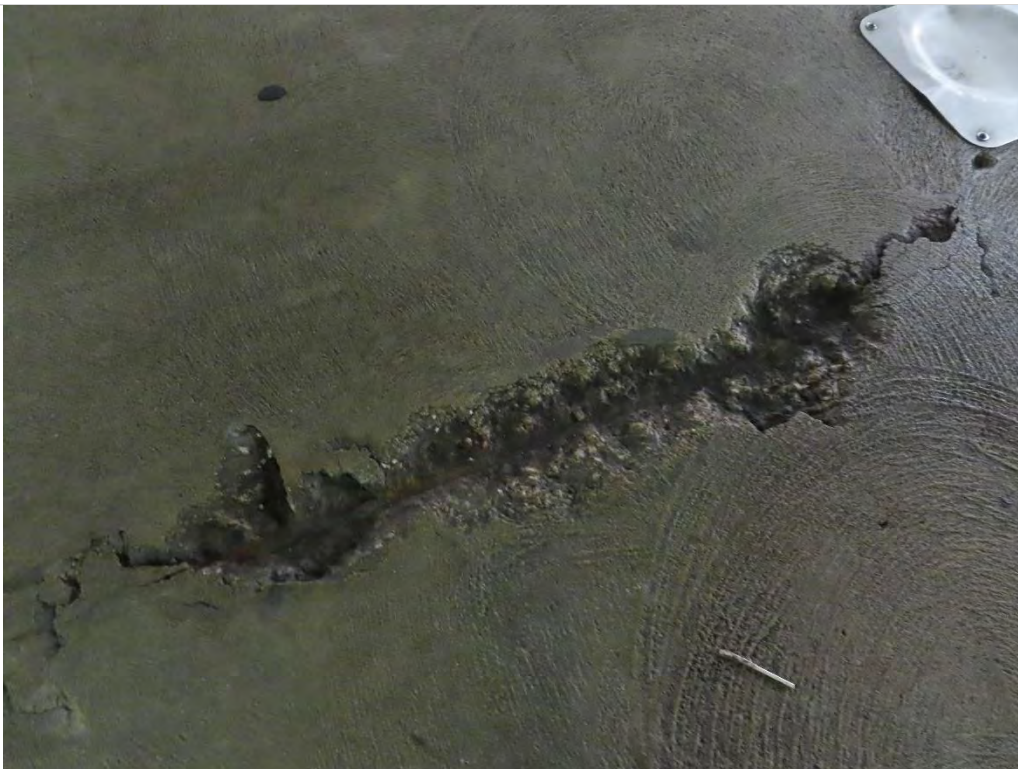
Photo 1.36- Deteriorated slab on grade, Basin level (SH2-44)
