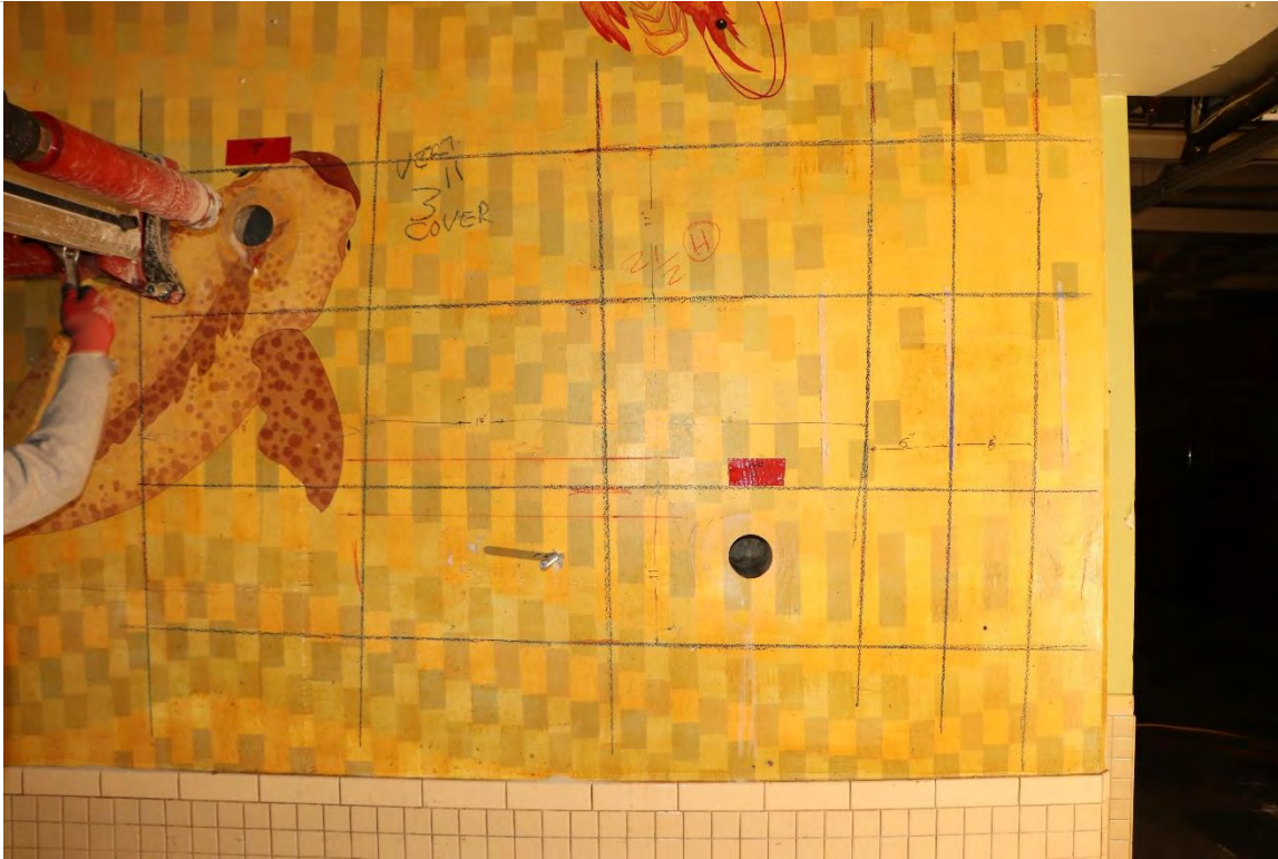
Photo 2.7- Concrete coring, Kitchen wall at gridline 3, 1962 Construction - Basement (BA2-102)
