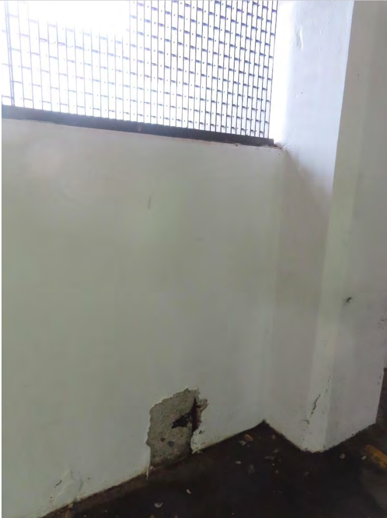
Photo 2.12- Exposed rebar on wall, Basin level (SH2-198)
