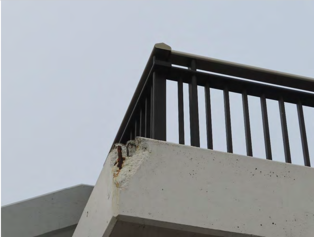
Photo 3.1- Exposed and corroded rebar, Exterior - South elevation (SH2-252)
