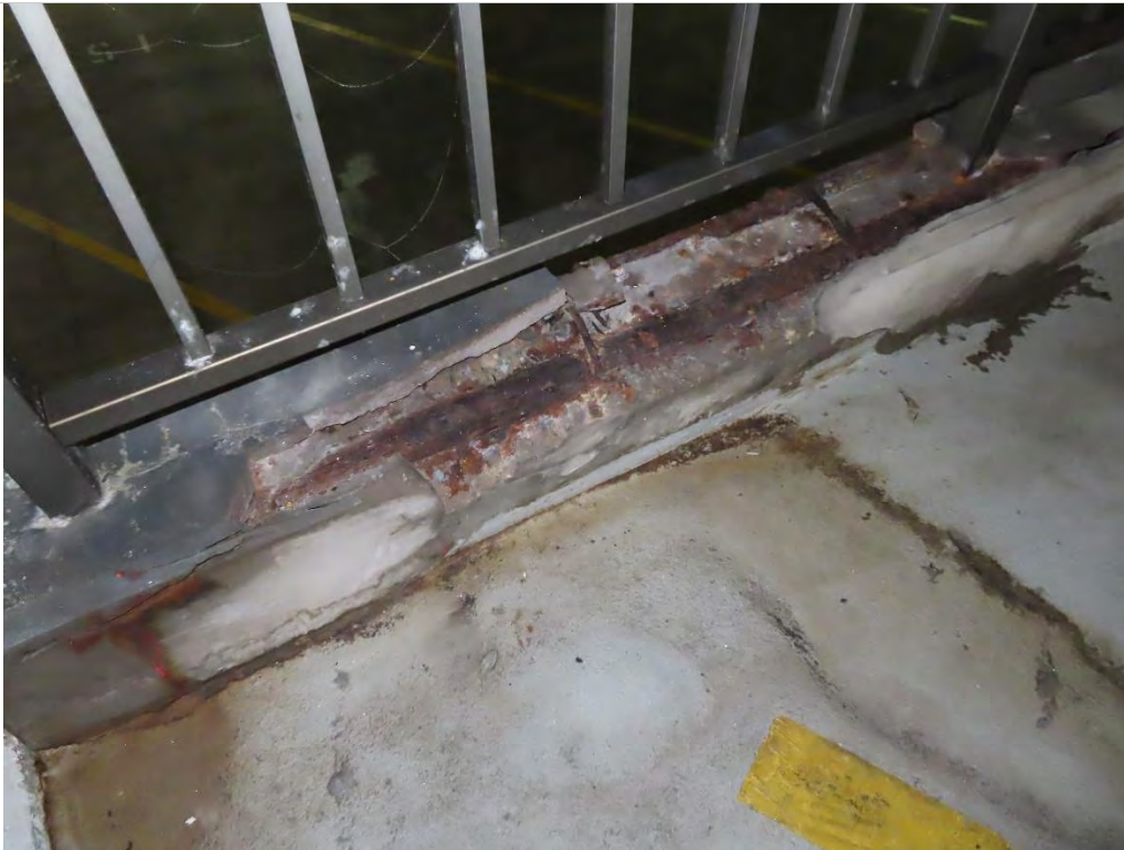
Photo 1.23- Isolated slab edge spall, Pier level (SH1-198)
