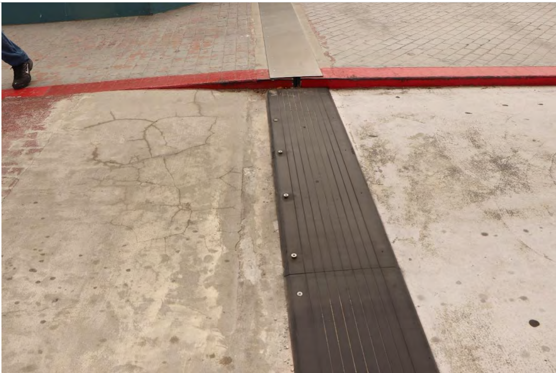
Photo 1.12- Expansion joint cover plate bolts projecting out, Village level (BA1-139)
