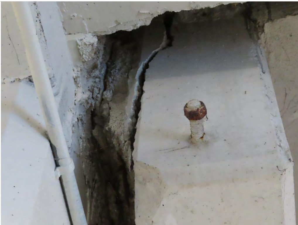
Photo 1.11- Concrete beam spall, Pier Level (SH3-197)
