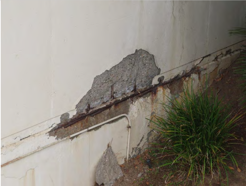
Photo 3.3- Concrete delamination, Exterior - South elevation (SH2-262)
