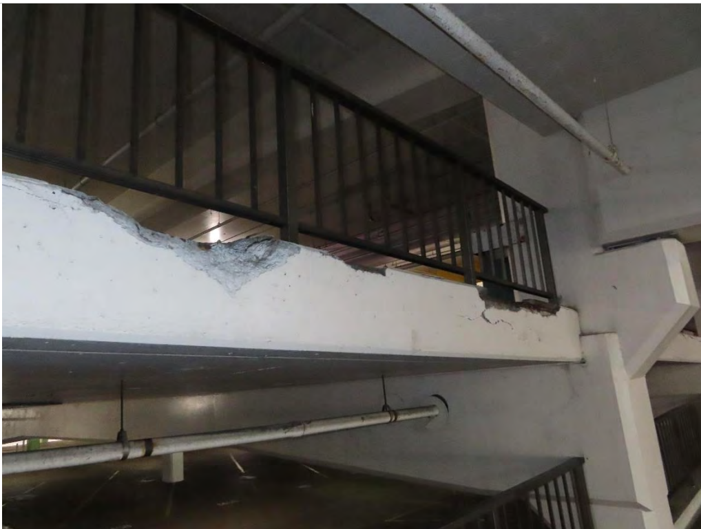
Photo 1.22- Isolated slab edge spall, Pier level (MM1-129)
