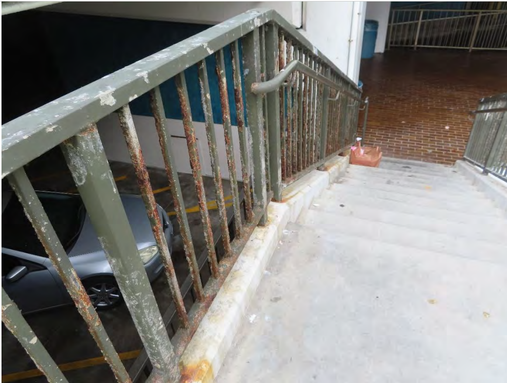
Photo 1.42- Corroded stair railing, (SH2-104)
