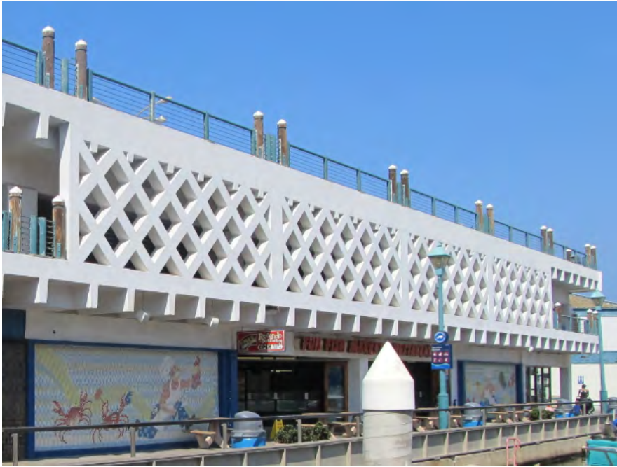
Photo 3.7- 12-inch-thick waffle shear wall at line Z.1 at Pier Level
