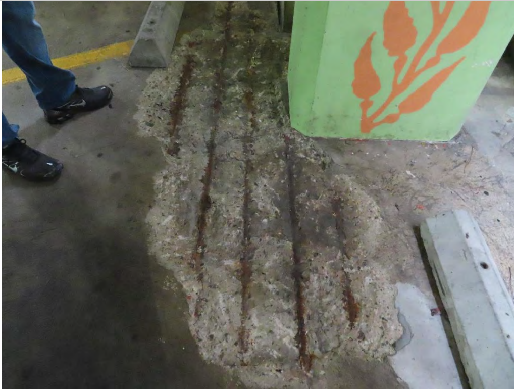
Photo 1.19- Exposed rebar on floor, Pier level (SH2-8)
