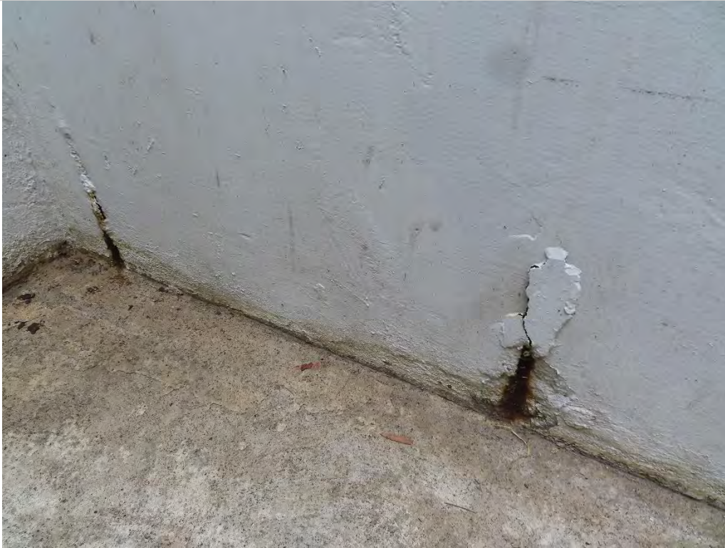
Photo 2.11- Exposed rebar on wall, Basin level (SH2-166)
