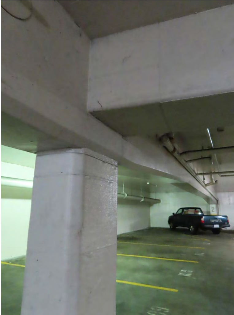
Photo 1.33- Fiber reinforcing wraps with added concrete cover, Basin level (SH1-271)
