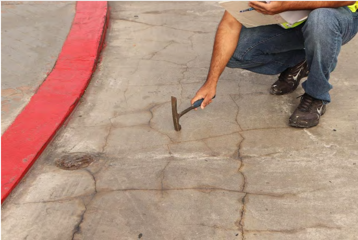
Photo 1.1- Concrete delamination, Village level (BA1-50)
