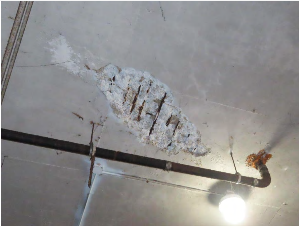
Photo 1.35- Corroded drainpipe, Pier level (MM1-82)
