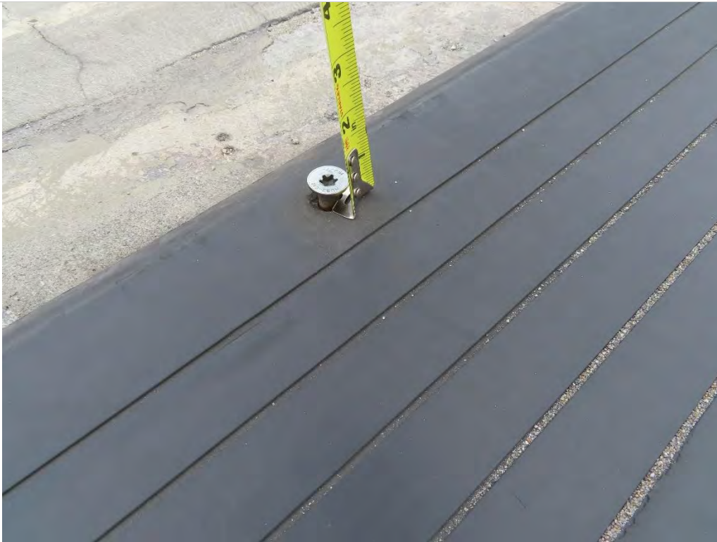
Photo 1.13- Expansion joint cover plate bolts projecting out, Village level (SH1-185)
