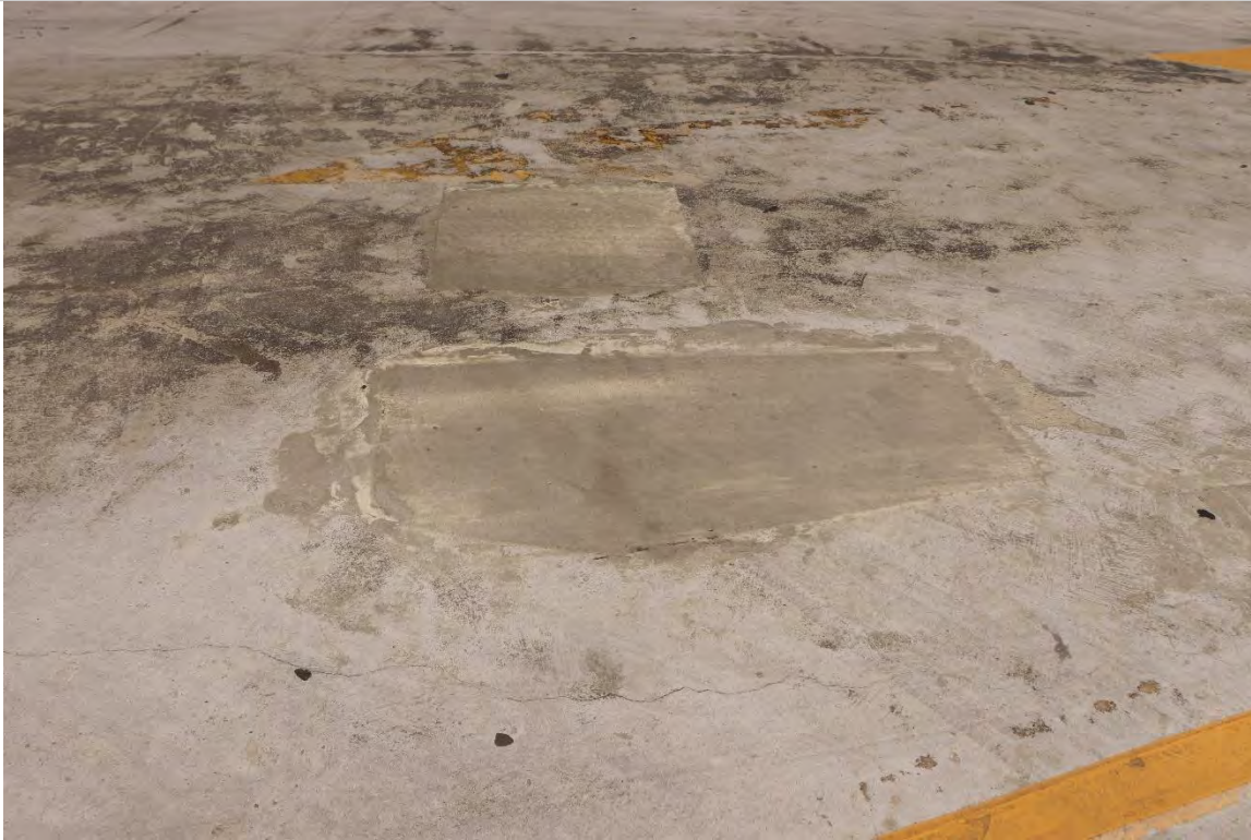
Photo 1.3- Delaminated previous repair, Village level (BA1-111)
