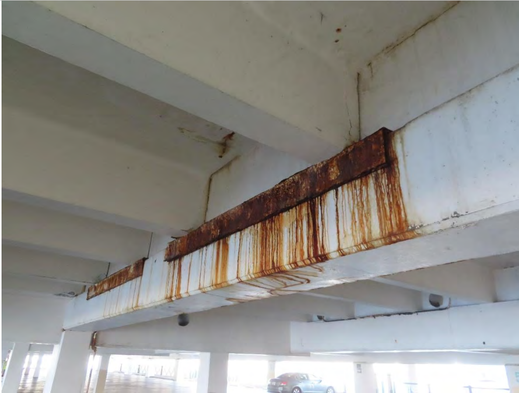
Photo 1.17- Exposed rebar on wall, Basement Level (SH3-308)
