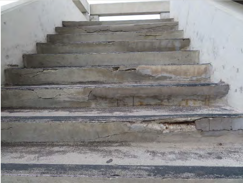
Photo 2.14- Damaged concrete stair treads and risers, (SH2-209)
