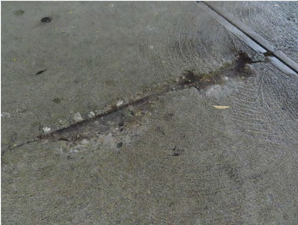
Photo 1.20- Exposed rebar on floor, Pier level (SH2-17)
