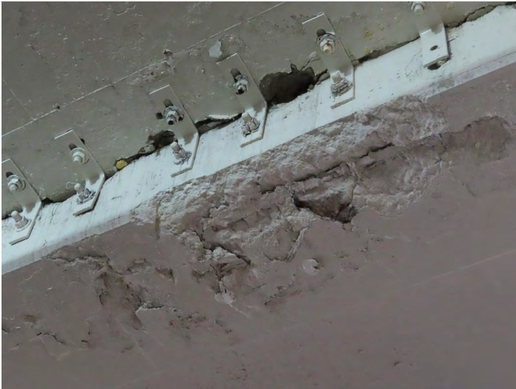
Photo 1.30- Concrete beam spalling below the expansion joint, Pier level (MM1-46)
