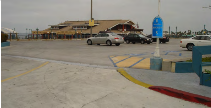
Photo 3.3- 2 ½-inch-thick overlay of CIP topping slab – Village Level
