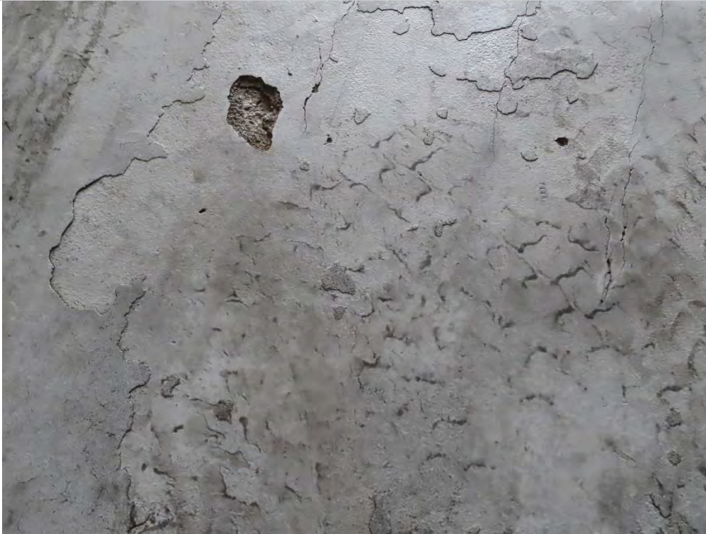
Photo 1.31- Compromised traffic membrane, Pier level (SH1-52)
