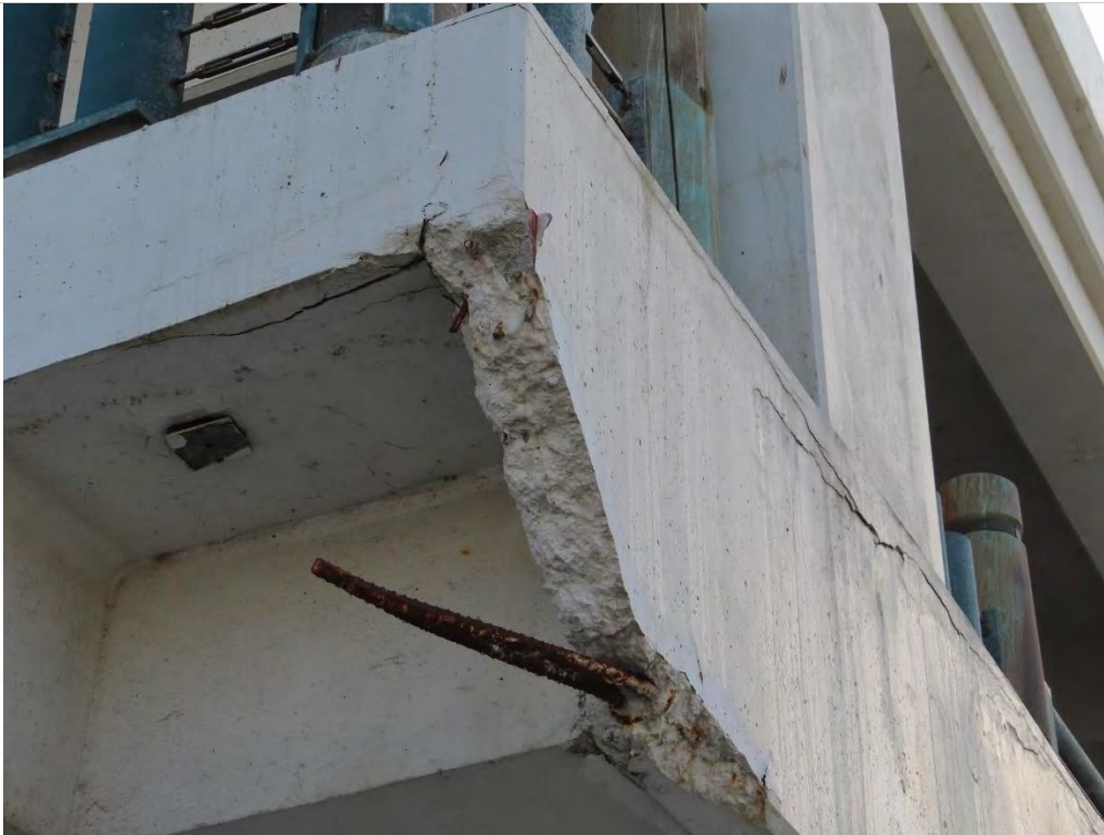
Photo 1.24- Concrete spandrel beam spall with exposed rebar, Exterior – North-east elevation (SH2-362)
