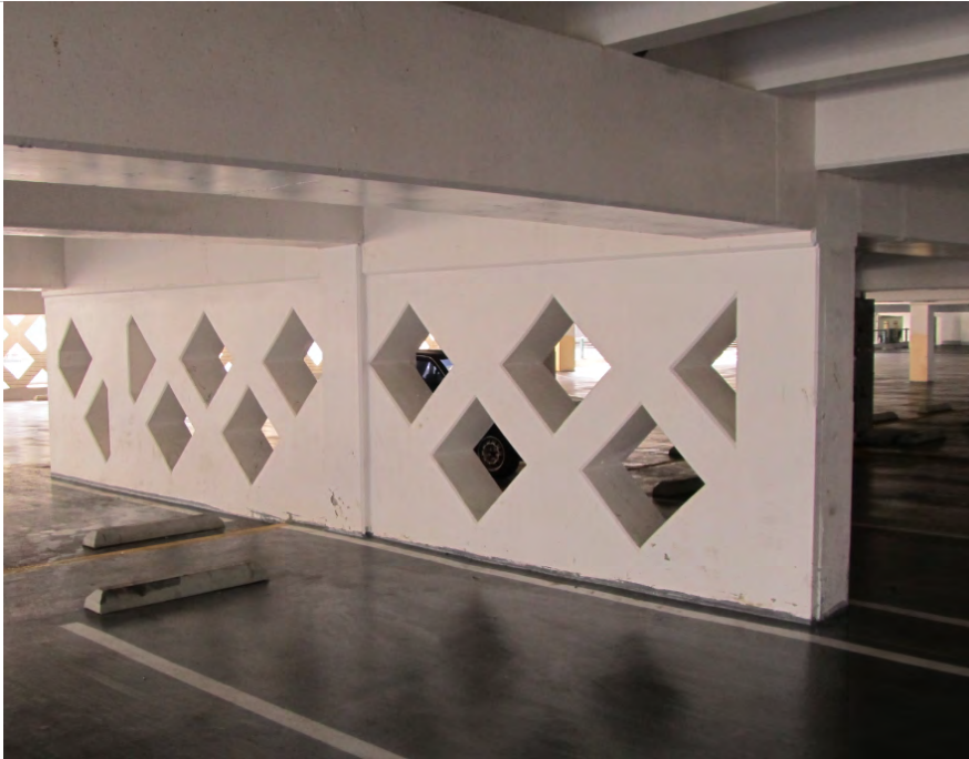
Photo 3.5- 12-inch-thick waffle shear wall at line 3 and Y at Pier Level
