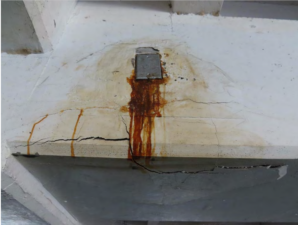
Photo 1.11- Concrete beam spall, Pier Level (SH3-197)
