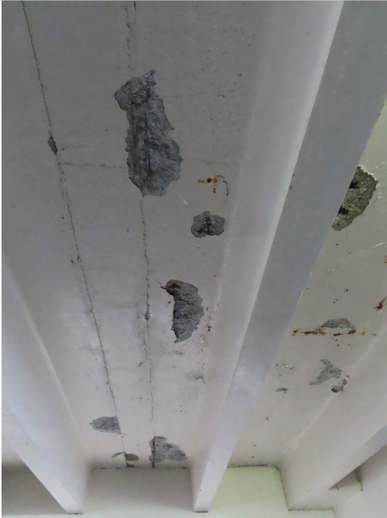
Photo 1.3- Soffit slab deterioration and spall with exposed reinforcement, Village Level (SH3-96)
