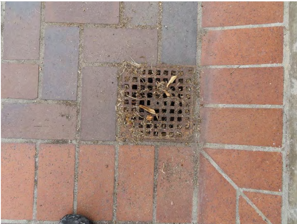
Photo 2.4- Clogged drains, Plaza level (SH2-267)
