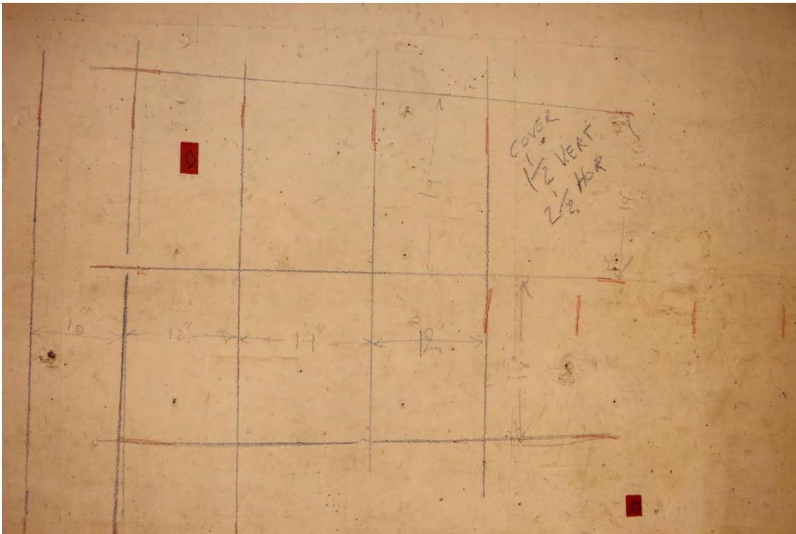
Photo 2.4- Wall steel reinforcement detected by GPR, South Wall Gridline 11, 1962 Construction - Basement (BA2-128)
