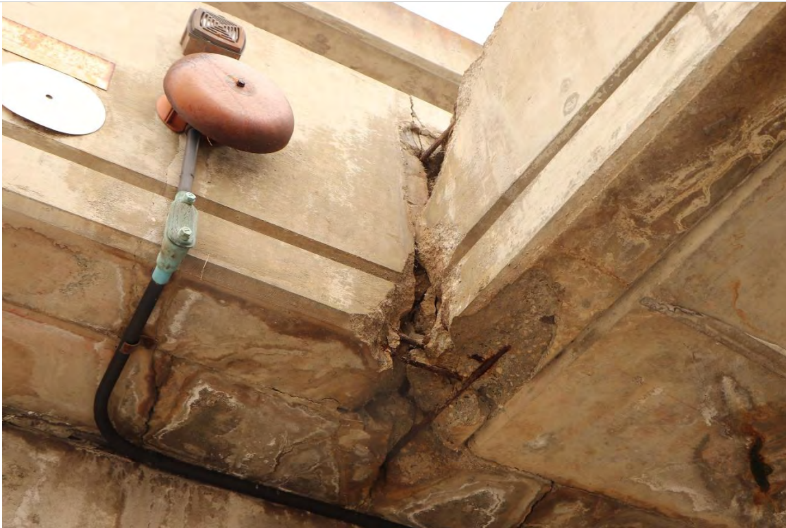
Photo 2.7- Soffit slab deterioration and spalls with exposed reinforcement, Pier level (BA1-327)
