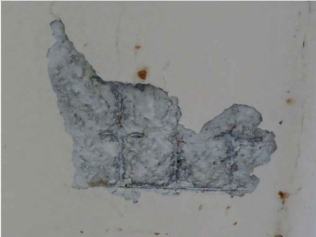
Photo 1.2- Soffit slab deterioration and spall with exposed reinforcement, Village Level (SH3-87)
