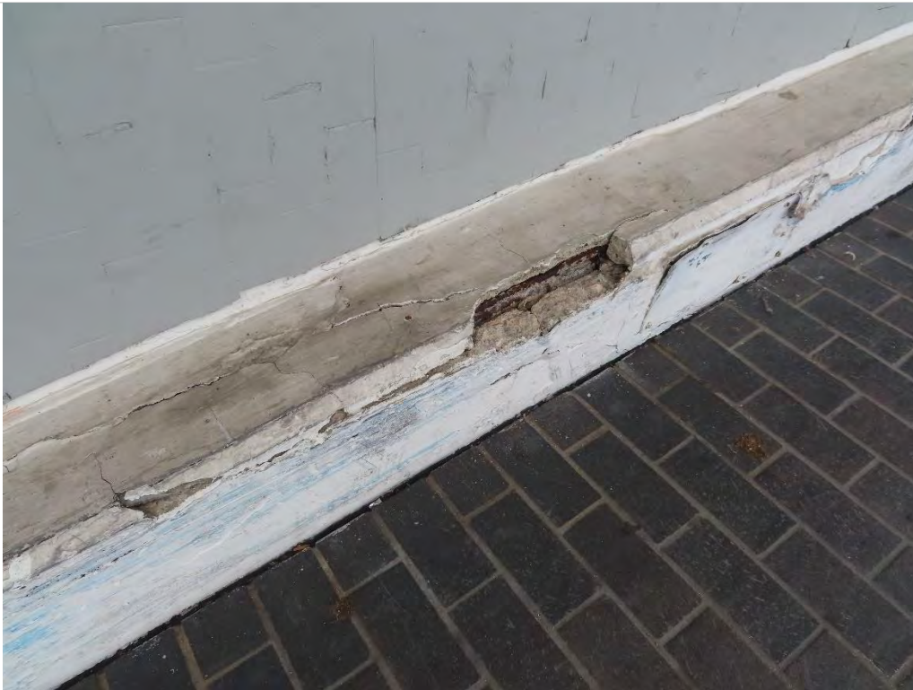
Photo 3.2- Exposed and corroded rebar, Exterior - South elevation (SH2-257)
