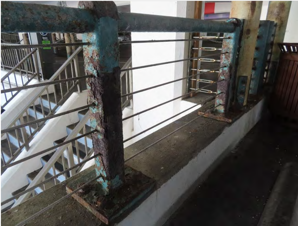
Photo 1.14- Corroded barrier post, Pier Level (SH3-192)
