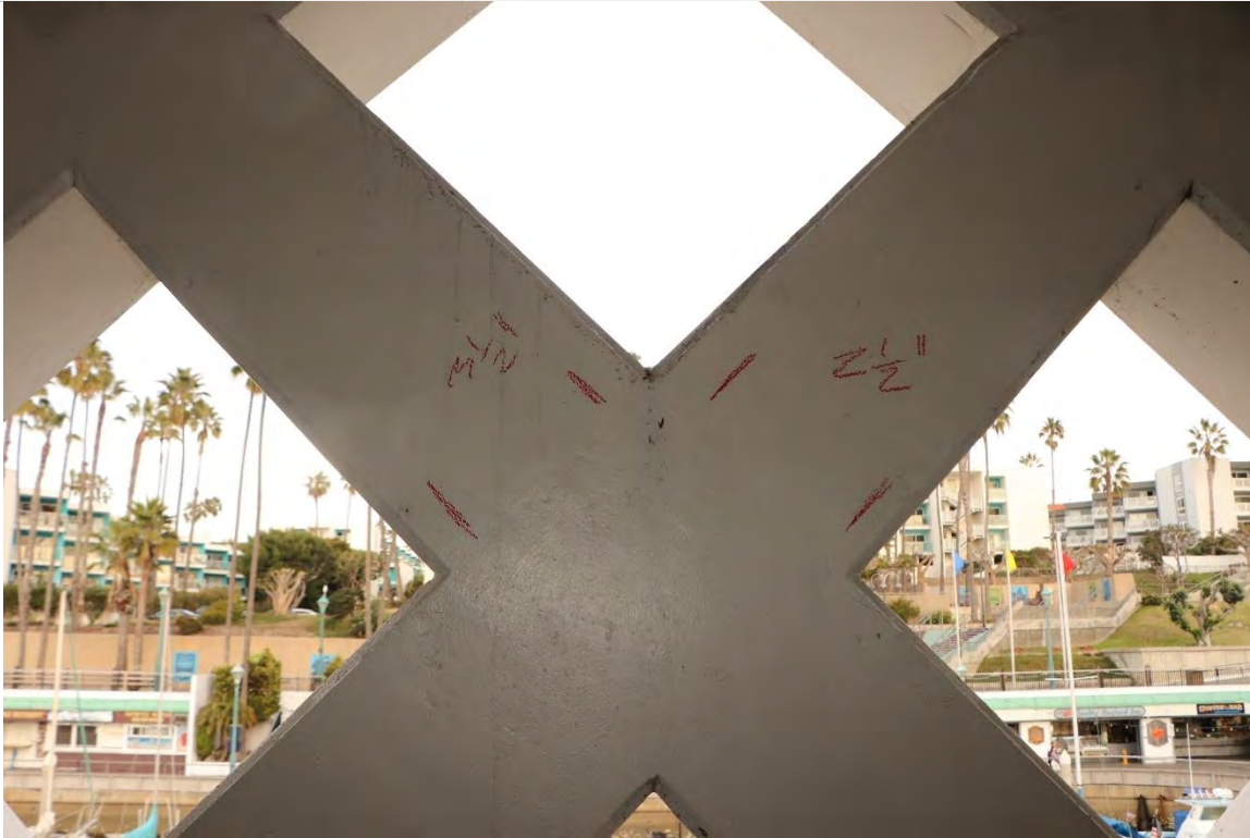
Photo 2.3- Wall steel reinforcement detected using GPR, only longitudinal bar was found, No confinement bar was present, East Wall, 1992 Retrofit – Pier Level (BA2-197)
