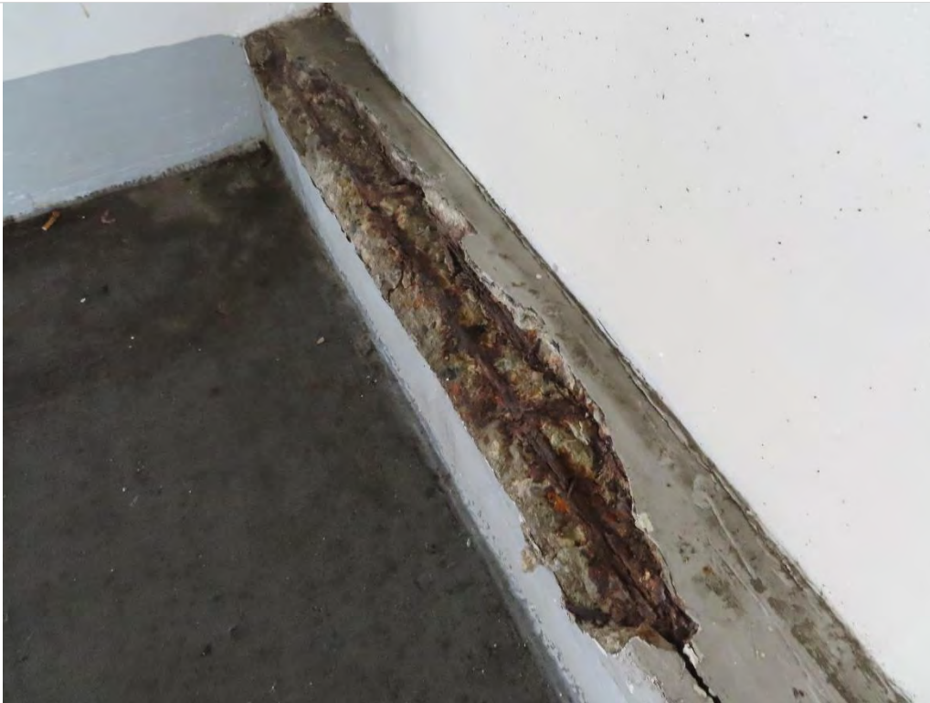
Photo 1.13- Concrete curb spall, Pier Level (SH3-189)
