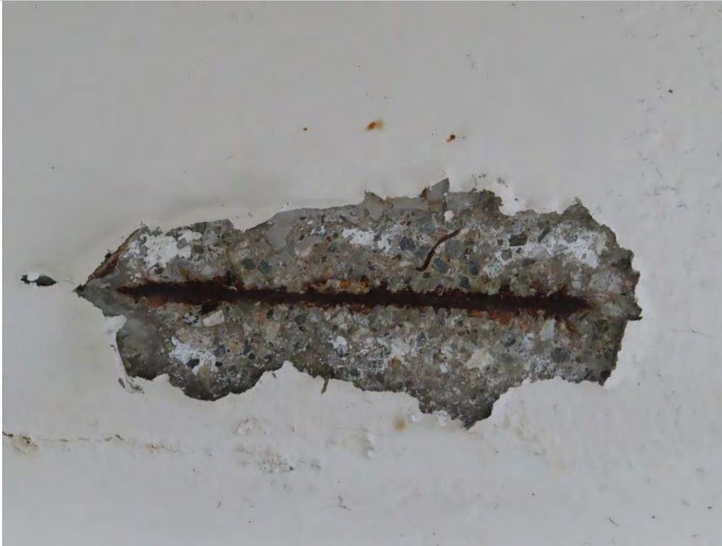
Photo 1.1- Soffit slab deterioration and spall with exposed reinforcement, Village Level (SH3-79)
