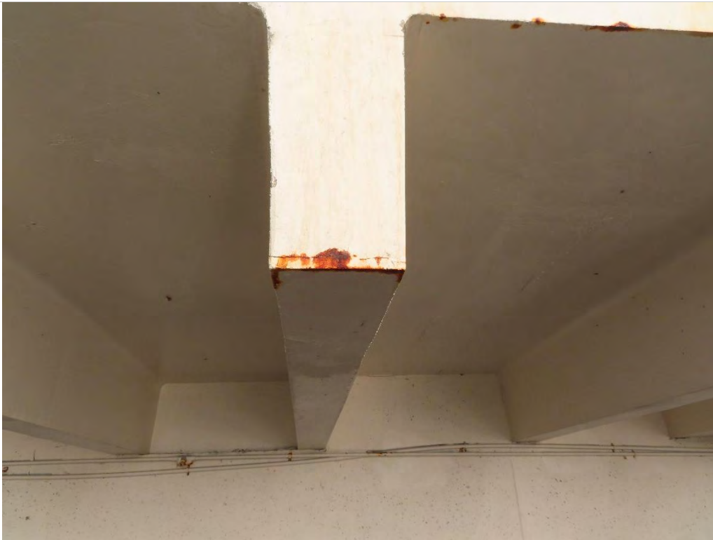
Photo 1.22 - Visual signs of rebar corrosion, Exterior - West elevation (SH2-343)
