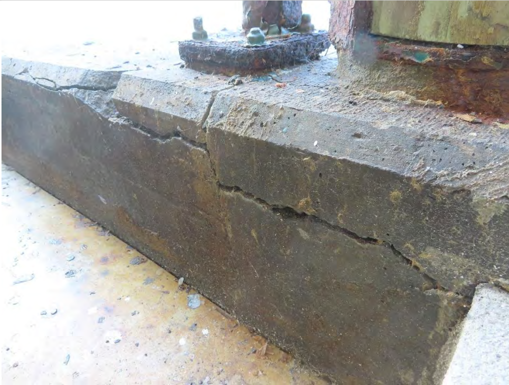
Photo 1.13- Concrete curb spall, Pier Level (SH3-189)
