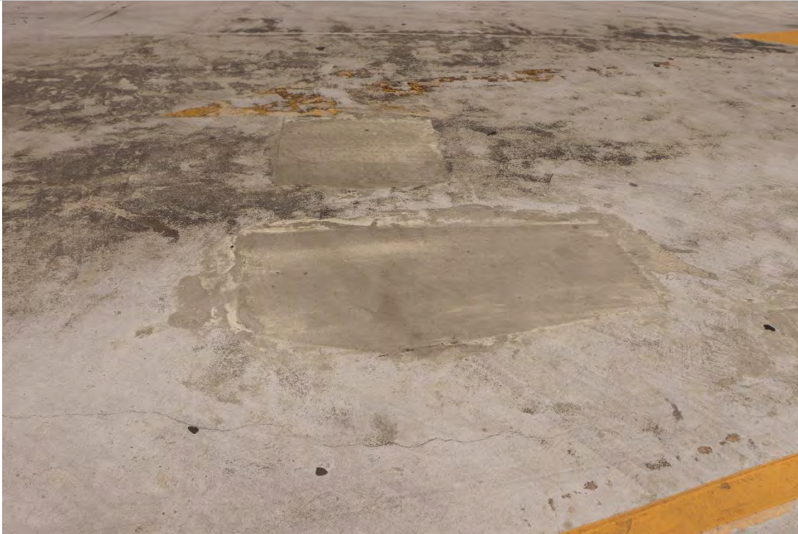
Photo 1.3- Delaminated previous repair, Village level (BA1-111)
