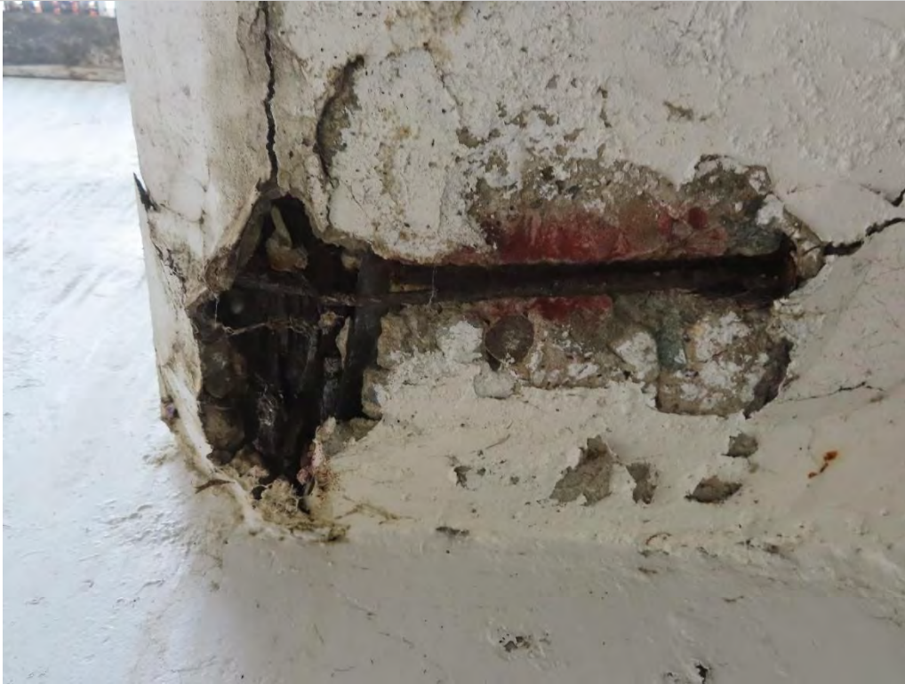
Photo 2.15- Damaged beam P/T rebar, Basin level (SH2-174)
