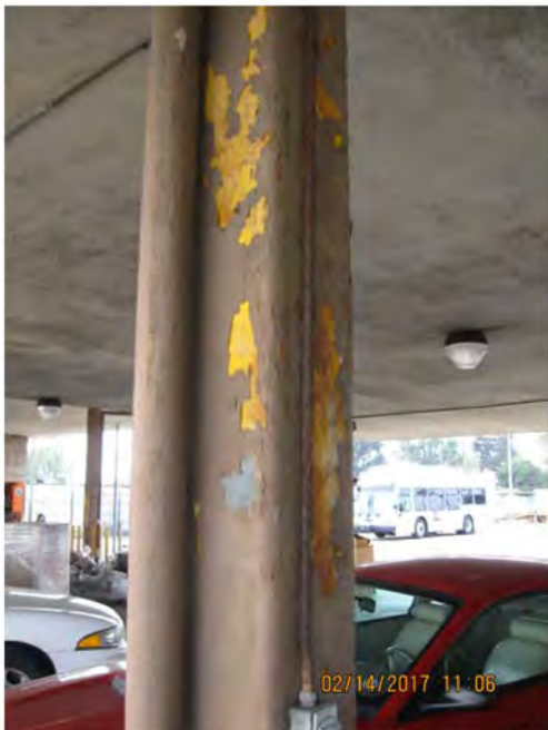
4A. Damaged yellow and brown paint on columns
