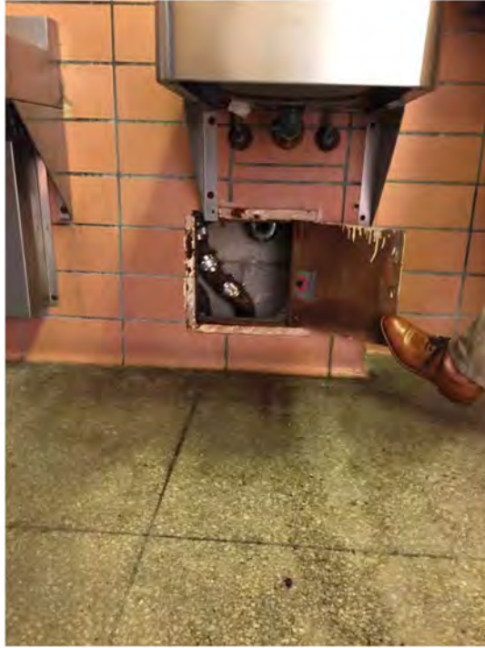
5. Exterior ceramic tile (non-lead) and pipe insulation (non-asbestos)
