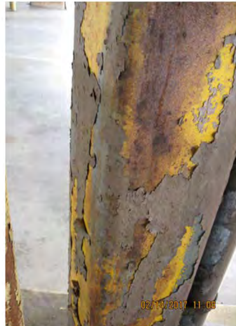
4B. Damaged yellow and brown paint on columns
