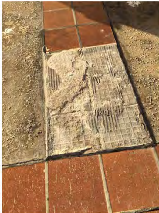
10. Exterior concrete, terrazzo tile, level coat and concrete substrate. No asbestos or lead.
