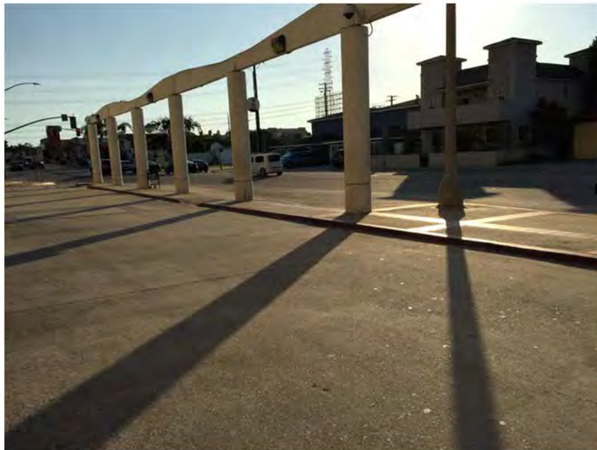
2. Existing RB Transit Center bus parking. Round plaster columns. No lead or asbestos in the columns; lead was identified in red-painted, concrete curbs.
