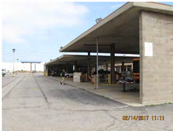
2. Concrete shade structure, looking northeast. The upper, south roof overlaps the lower north roof by approximately 10 feet.
