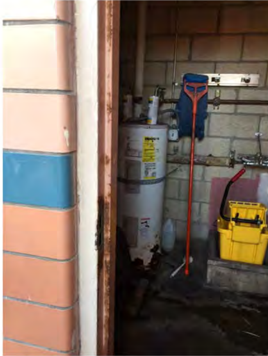
7. Utility closet – fiberglass pipe insulation - no asbestos or lead detected.
