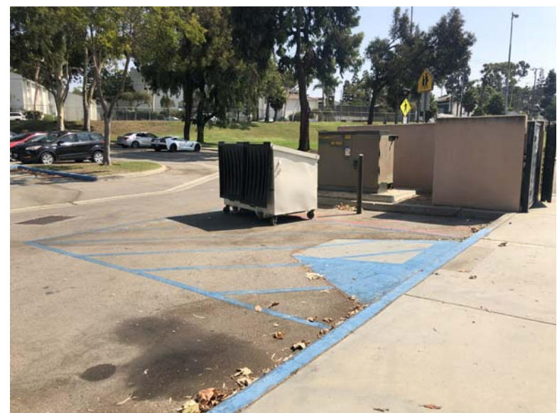
EXISTING A.D.A. RAMP TO BE REPLACED, RE-STRIPE A.D.A. STALLS
