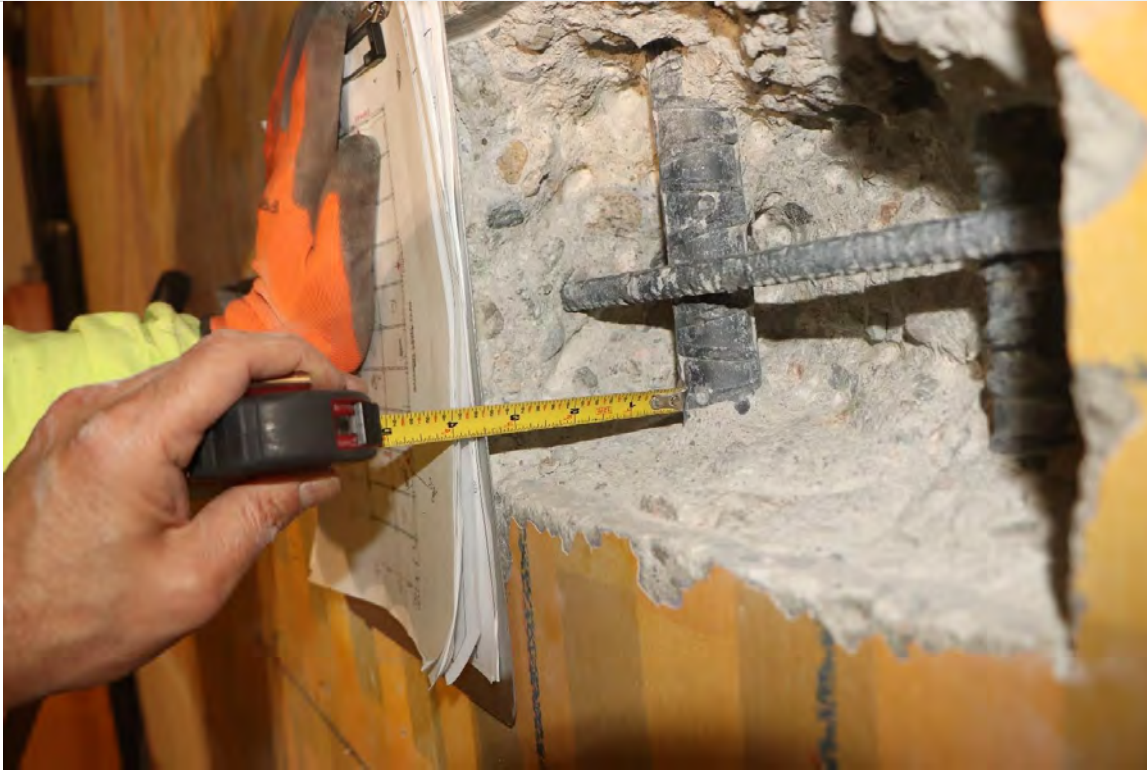
Photo 2.17— Vertical bar concrete cover measurement at wall jamb, destructive opening location DT4, Kitchen wall on gridline 3, 1962 Construction - Basement (BA2-594)
