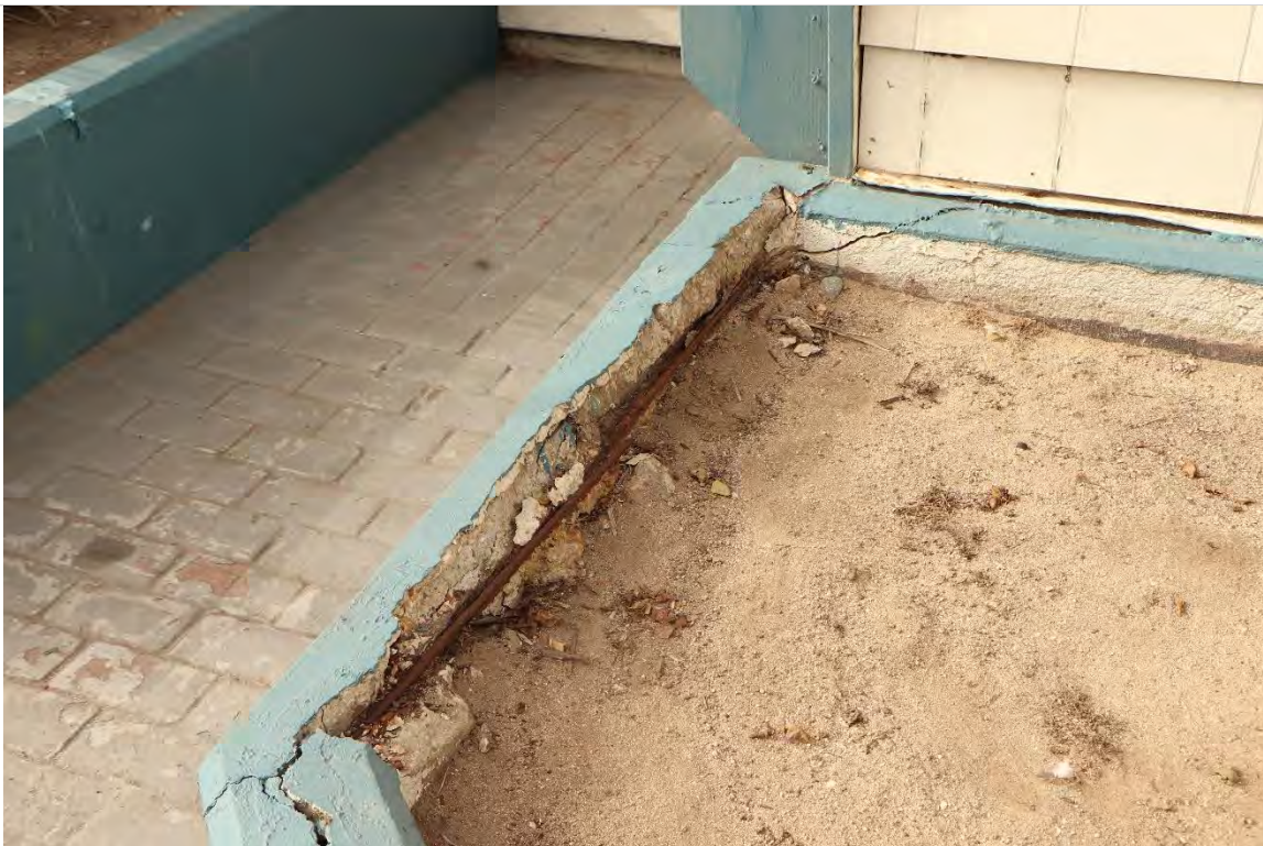
Photo 1.14- Typical spalled concrete planter walls, Village level (BA1-58)
