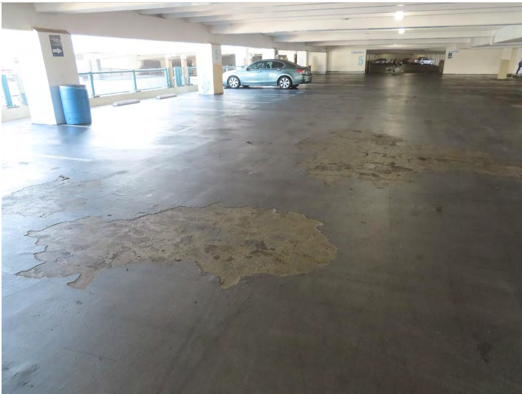
Photo 1.15- Compromised traffic coating, Pier Level (SH3-211)
