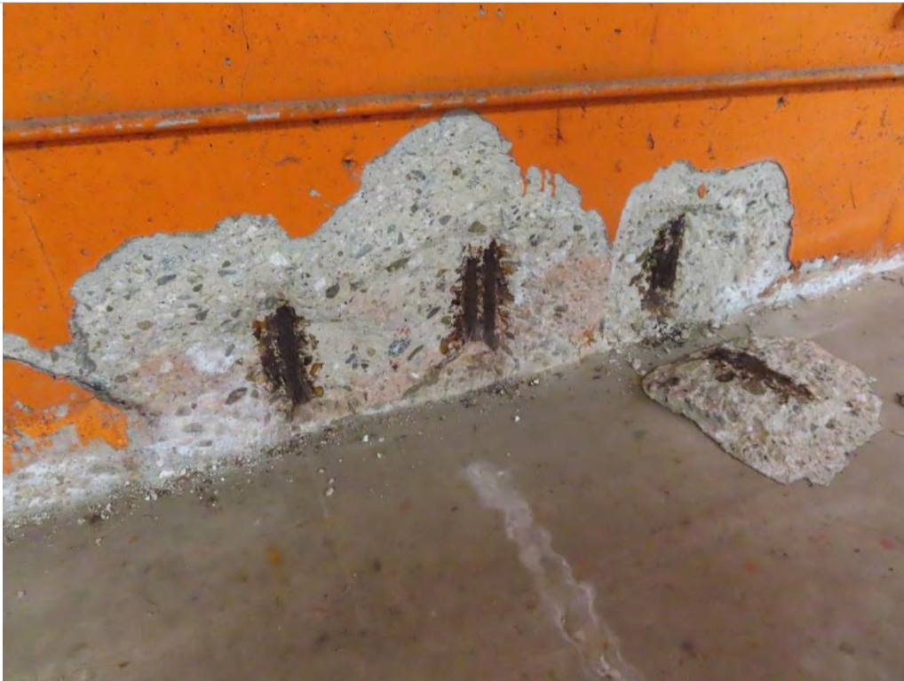
Photo 1.17- Exposed rebar on wall, Basement Level (SH3-308)
