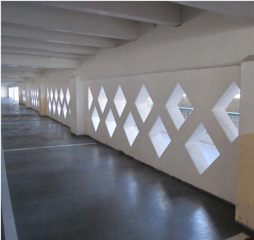
Photo 3.6- 12-inch-thick waffle shear wall along line X at Pier Level
