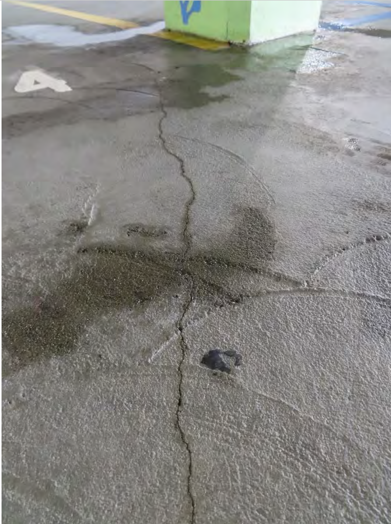
Photo 2.8- Cracks on concrete floor slab, Pier level (SH2-151)
