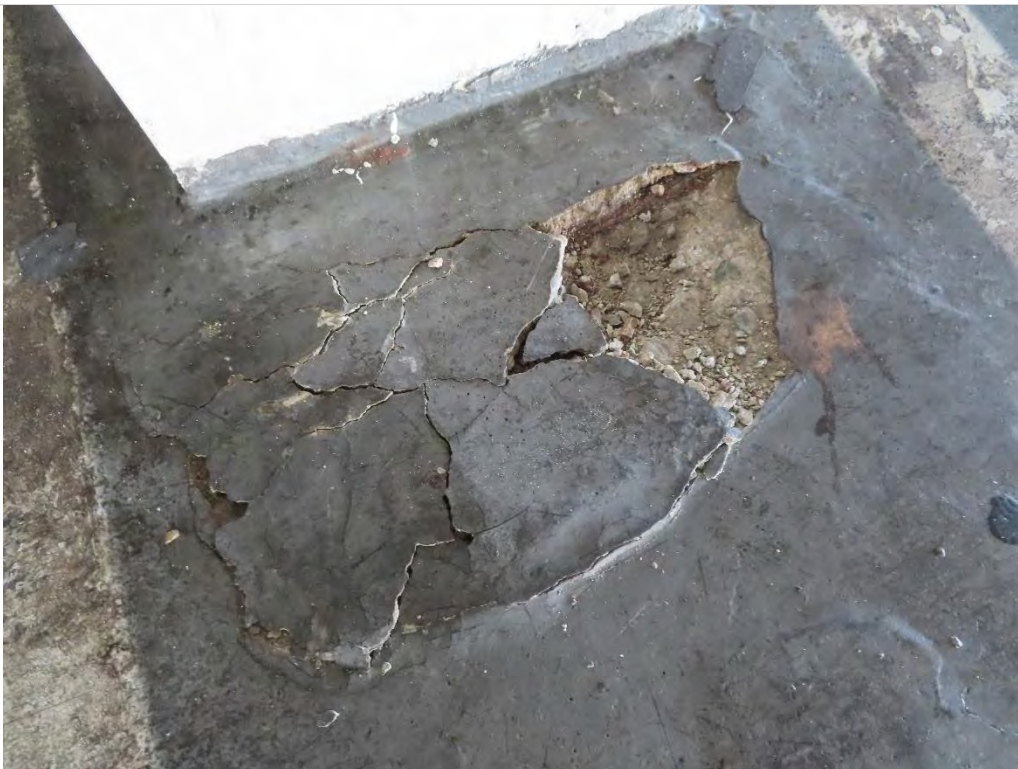
Photo 1.5- Concrete floor delamination, Pier Level (SH3-229)
