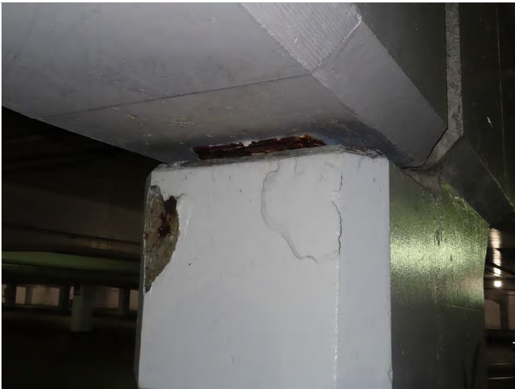
Photo 1.38- Isolated concrete column spalls, Basin level (SH1-241)
