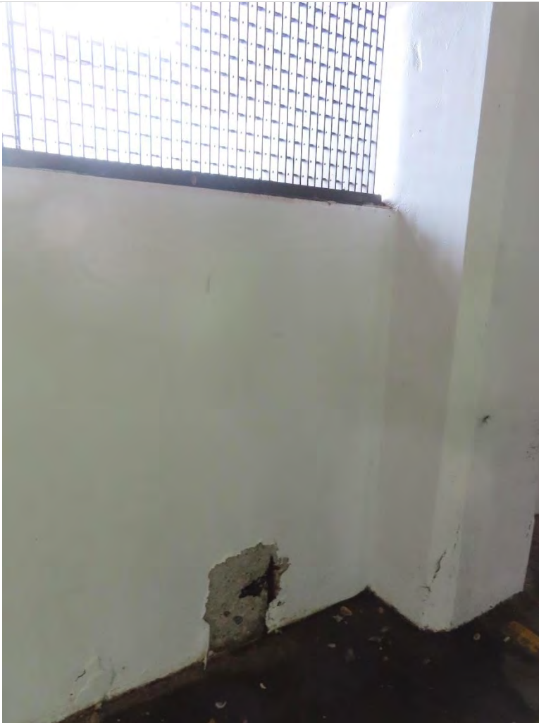
Photo 2.12- Exposed rebar on wall, Basin level (SH2-198)
