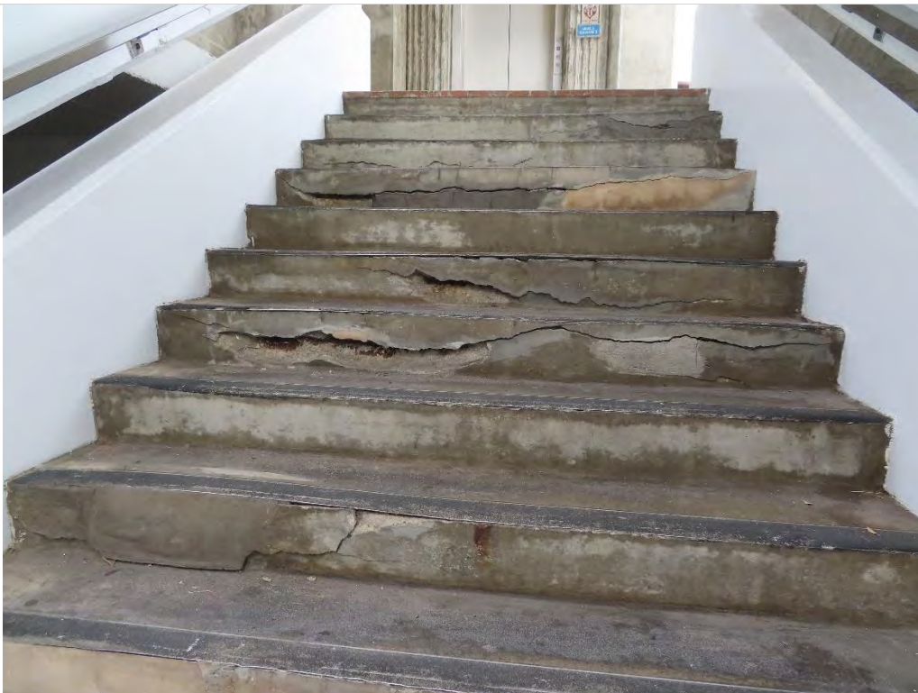
Photo 2.14- Damaged concrete stair treads and risers, (SH2-209)
