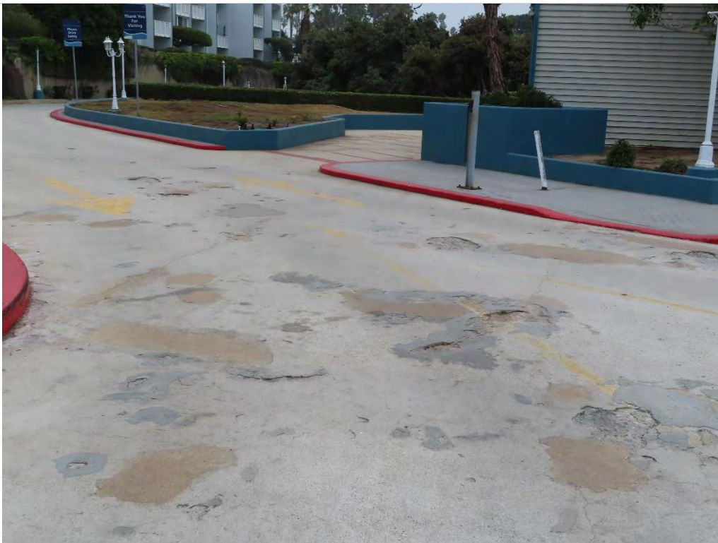
Photo 1.2- Concrete delamination, Village level (SH1-167)
