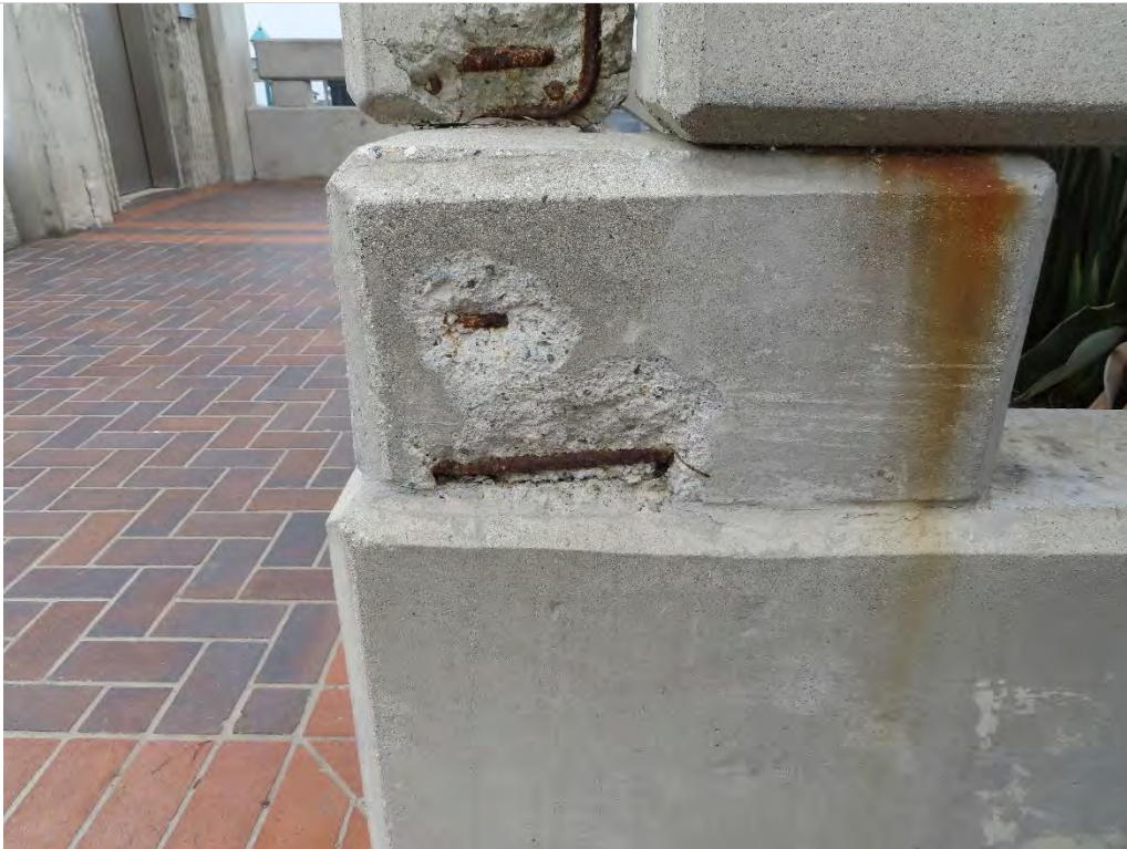
Photo 2.2- Spalled precast concrete spandrel with exposed rebar, Plaza level (SH2-266)
