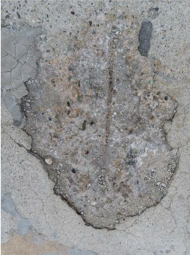
Photo 1.6- Exposed rebar on floor, Village level (SH1-168)
