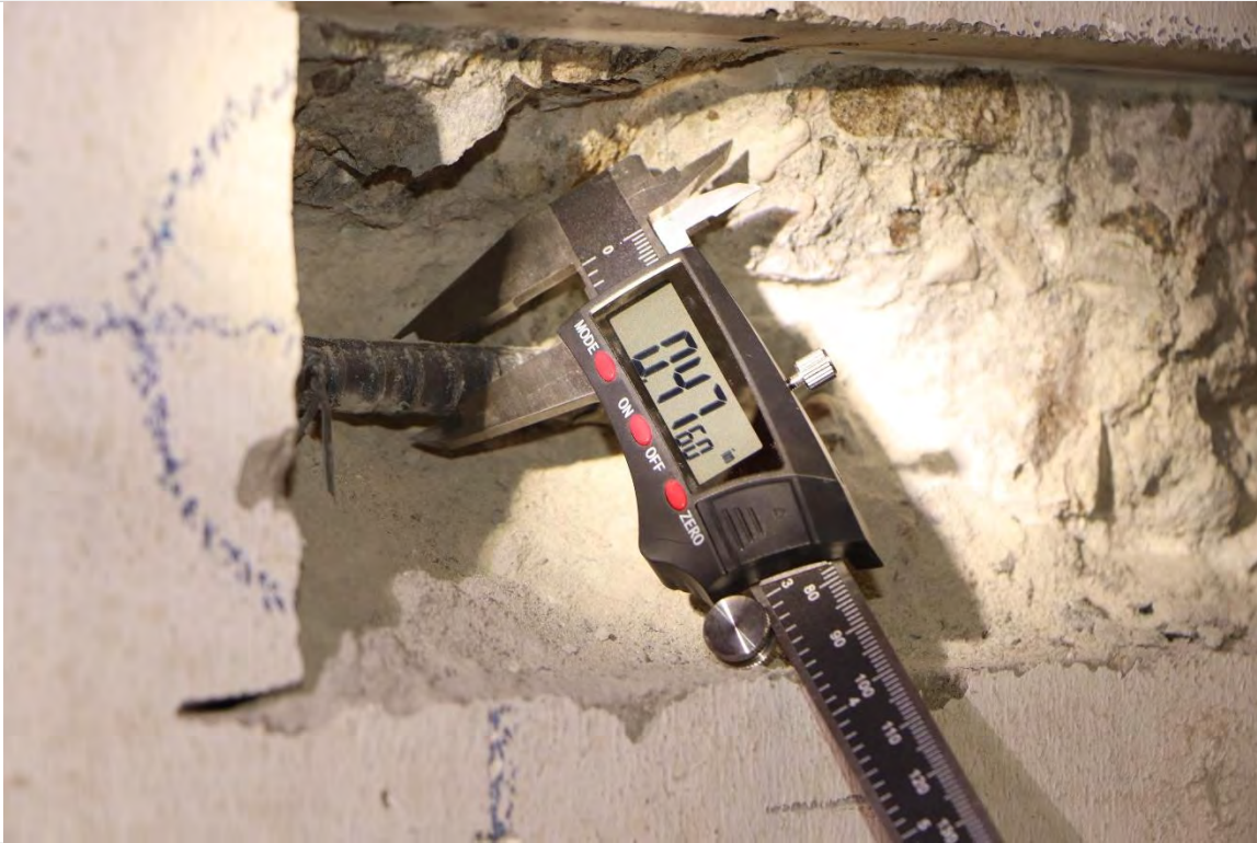
Photo 2.16— Vertical #10 bar found at wall jamb, destructive opening location DT4, Kitchen wall on gridline 3, 1962 Construction - Basement (BA2-580)
