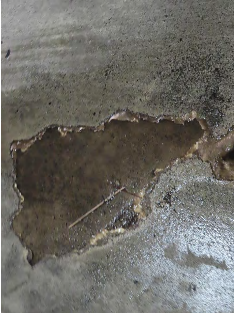
Photo 1.32- Compromised traffic membrane, Pier level (SH1-48)
