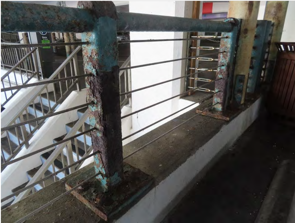
Photo 1.14- Corroded barrier post, Pier Level (SH3-192)
