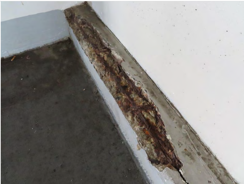
Photo 1.13- Concrete curb spall, Pier Level (SH3-189)
