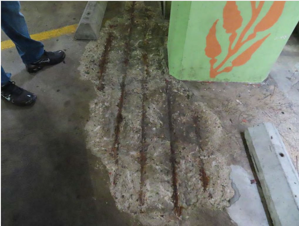
Photo 1.19- Exposed rebar on floor, Pier level (SH2-8)
