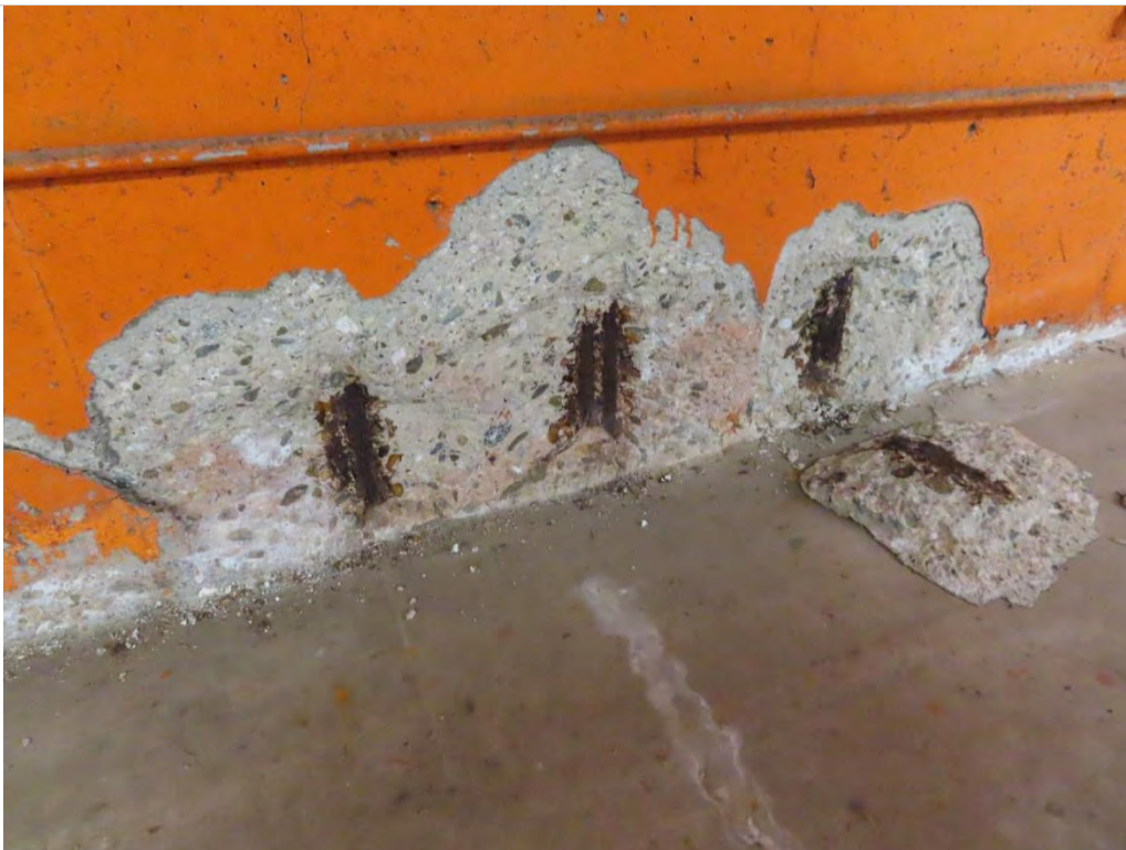
Photo 1.17- Exposed rebar on wall, Basement Level (SH3-308)
