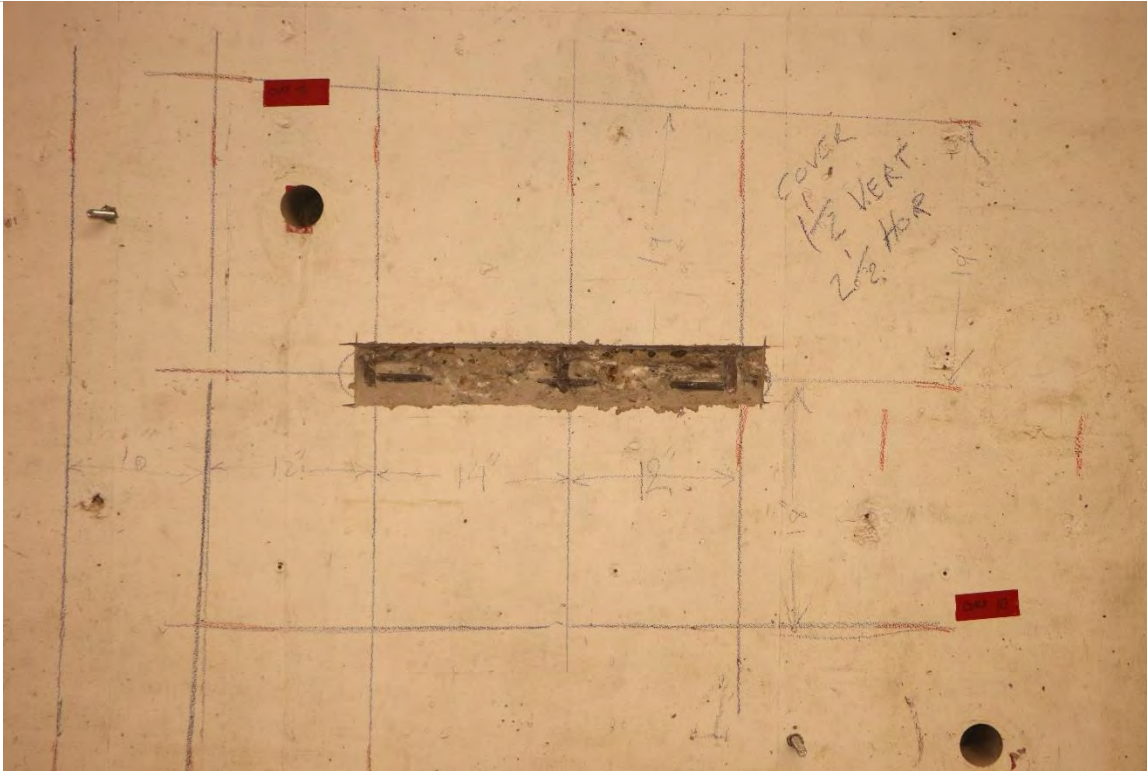
Photo 2.10—Destructive wall location (DT3), South wall, 1962 Construction - Basement (BA2-404)
