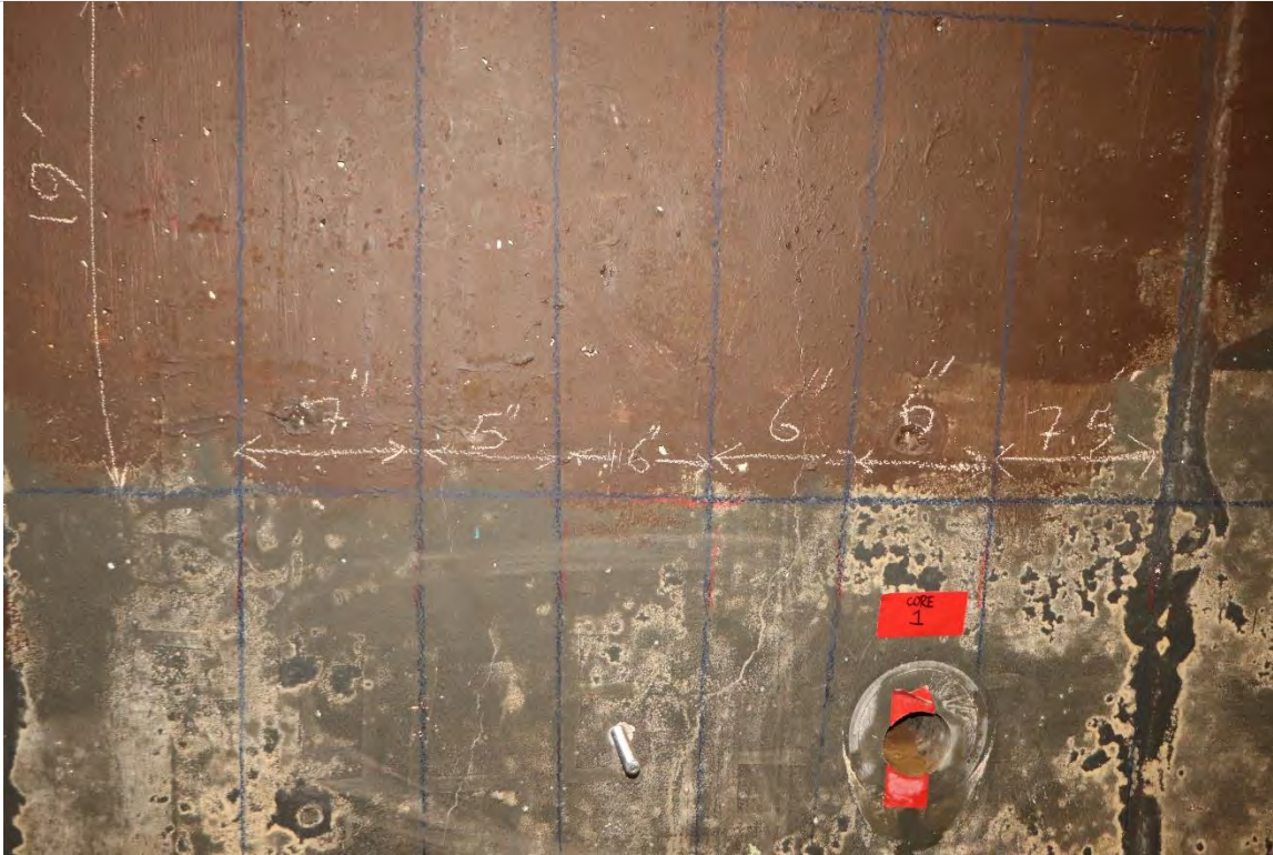
Photo 2.5- Concrete coring, West Wall, 1962 Construction - Basement (BA2-33)
