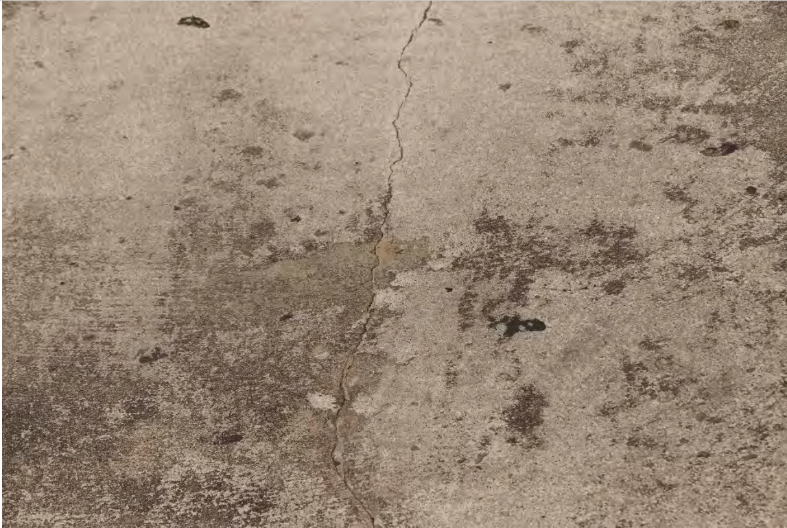
Photo 1.5- Cracks on concrete floor slab, Village level (BA1-80)
