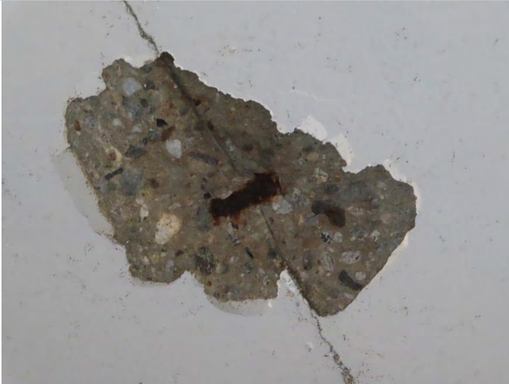
Photo 1.28- Soffit slab deterioration and spalls with exposed reinforcement, Pier level (SH1-249)
