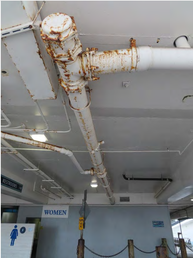
Photo 1.34- Corroded drainpipe, Pier level (MM1-33)
