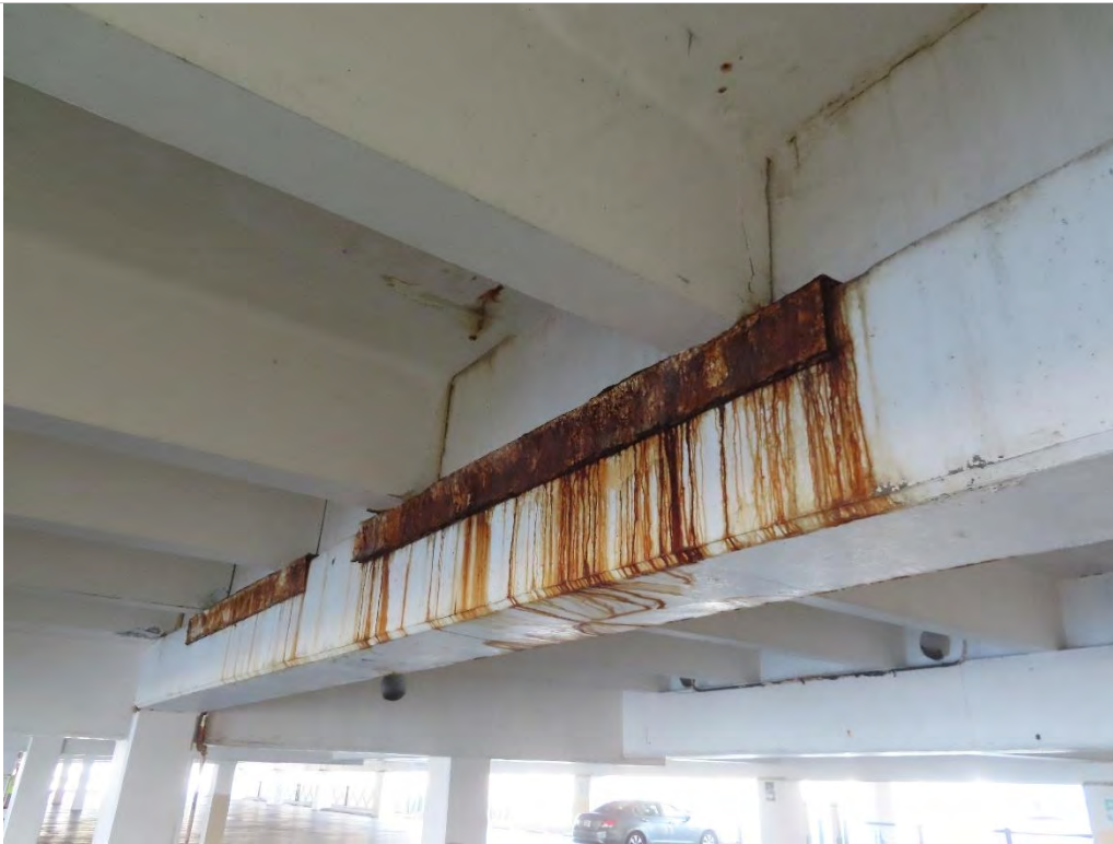
Photo 1.17- Exposed rebar on wall, Basement Level (SH3-308)
