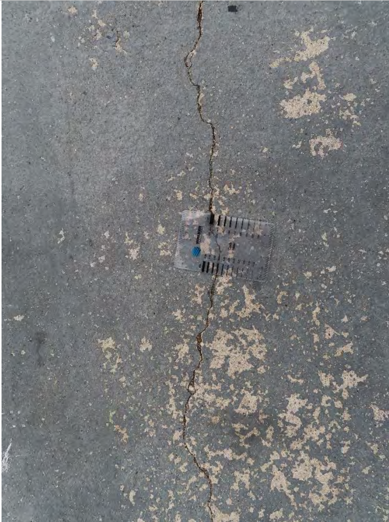
Photo 1.4- Cracks on concrete floor slab, Village level (SH1-165)
