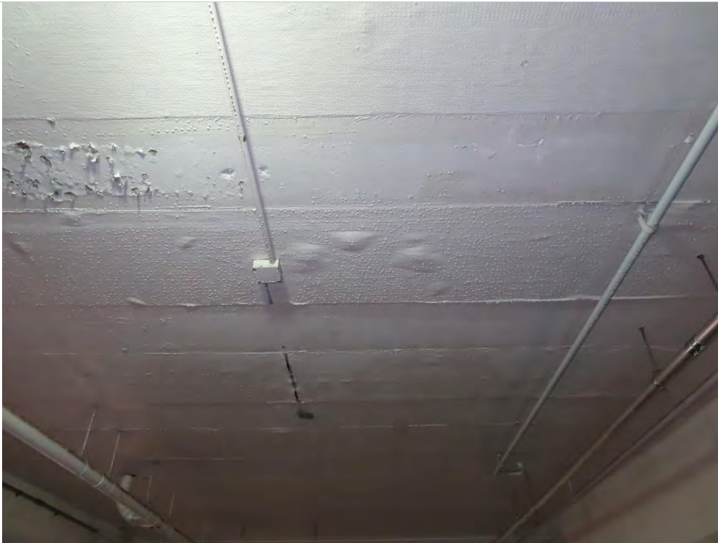
Photo 1.15- Deteriorated fiber reinforcing wrap, Village level (SH1-88)
