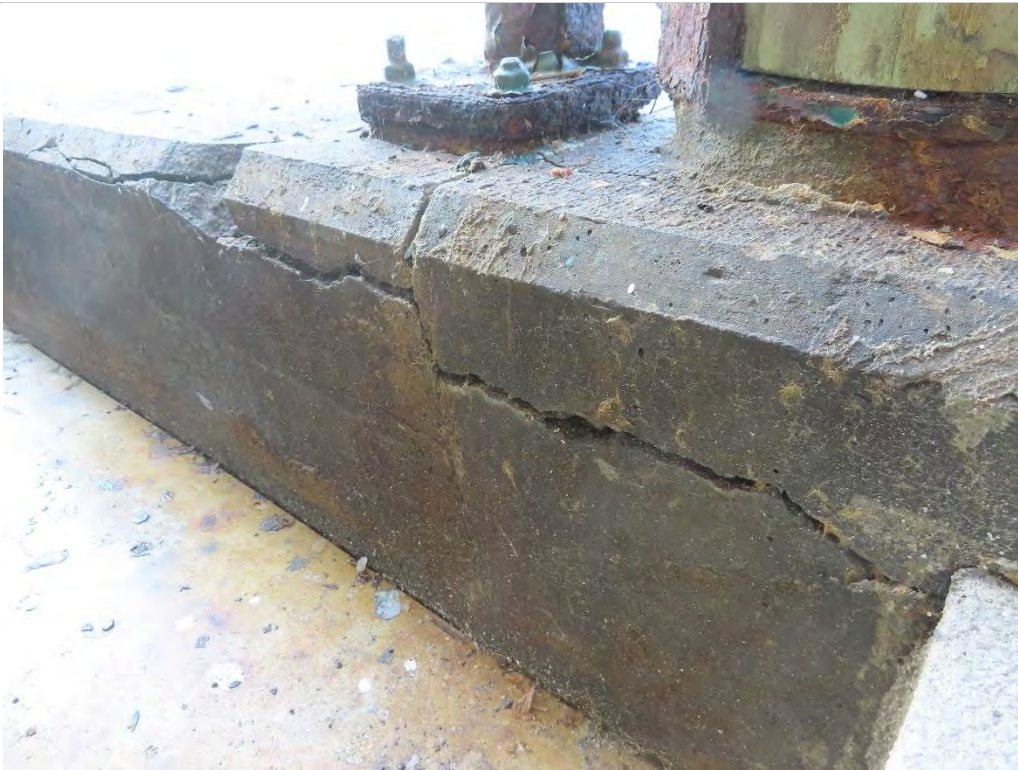
Photo 1.12- Concrete curb spall, Pier Level (SH3-35)
