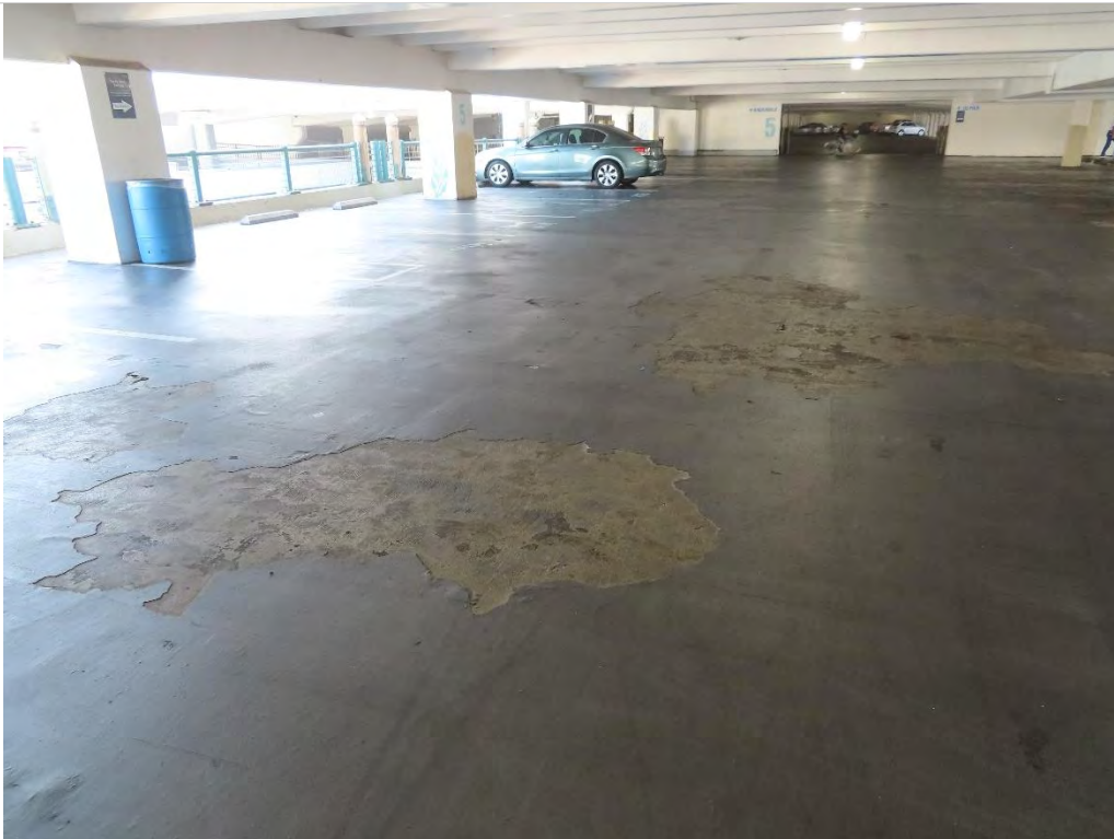
Photo 1.15- Compromised traffic coating, Pier Level (SH3-211)
