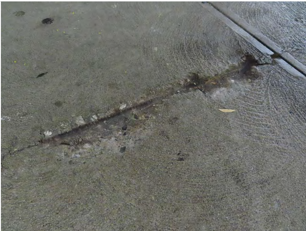
Photo 1.20- Exposed rebar on floor, Pier level (SH2-17)
