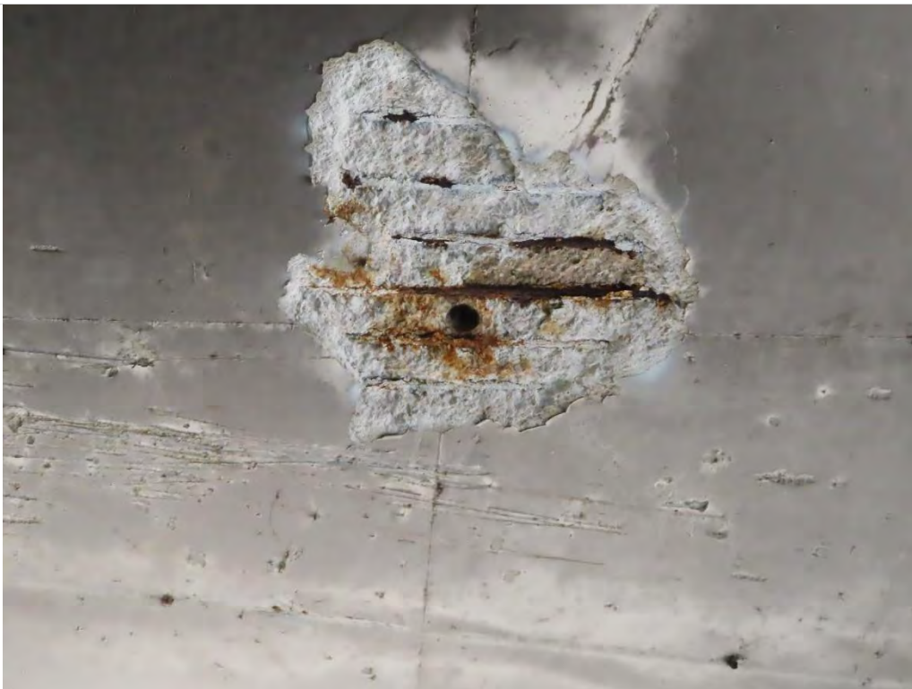
Photo 1.8- Soffit slab deterioration and spalls with exposed reinforcement, Village level (SH1-8)
