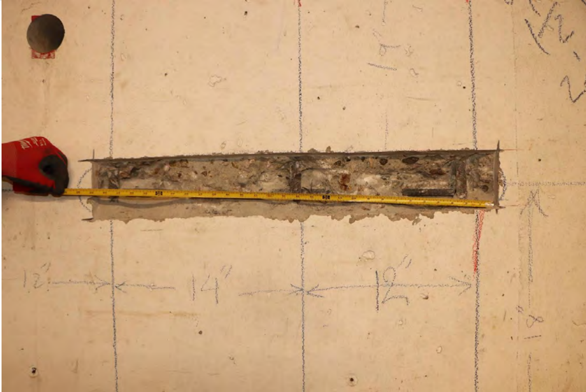
Photo 2.14— Vertical rebar placement at destructive location (DT3), South wall, 1962 Construction - Basement (BA2-409)
