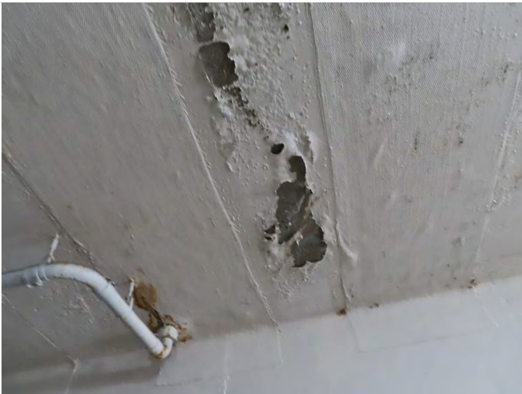
Photo 1.16- Deteriorated fiber reinforcing wrap, Village level (SH1-96)
