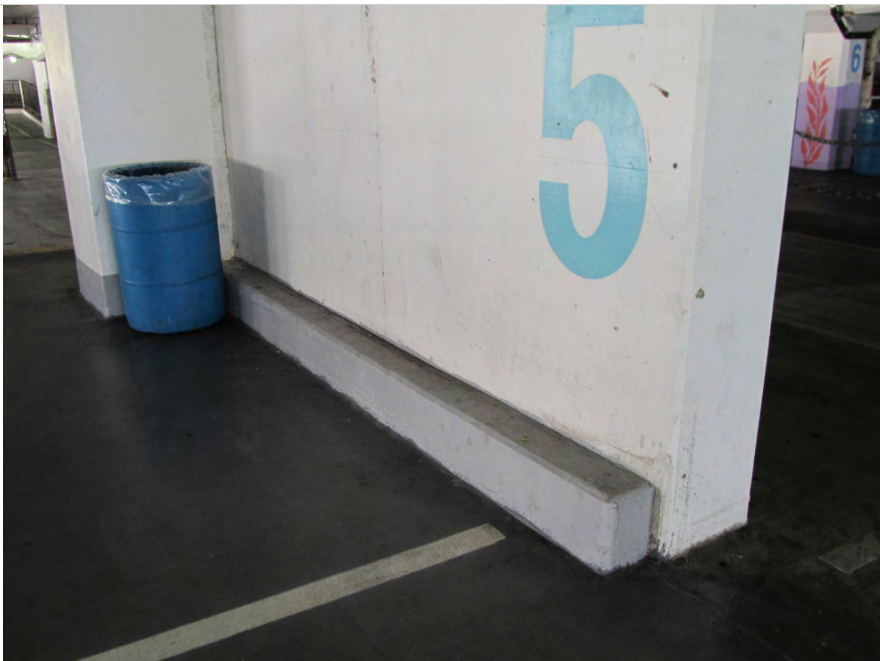
Photo 3.8- 10-inch-thick shear wall at line 11 and Y at the Pier Level
