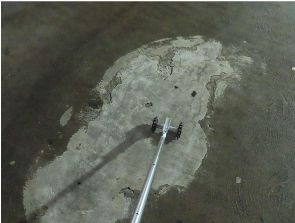
Photo 1.18- Concrete delamination, Pier level (SH2-21)
