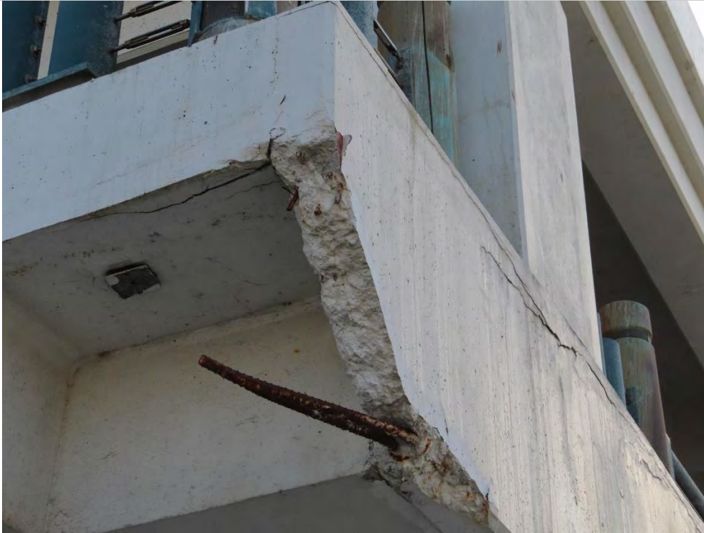
Photo 1.25- Concrete cantilever spandrel beam exposed rebar, Exterior – East elevation (SH2-372)
