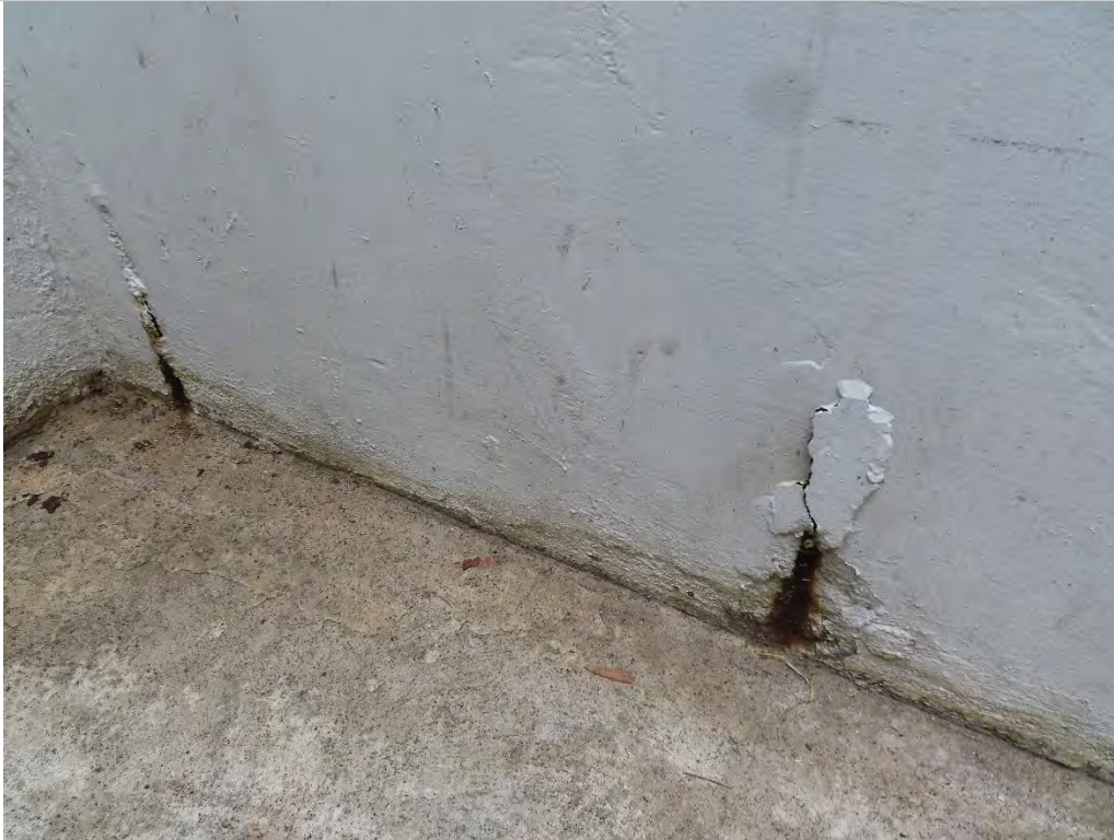
Photo 2.11- Exposed rebar on wall, Basin level (SH2-166)
