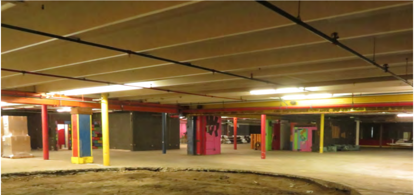
Photo 3.11—6-inch round steel columns at line X.7 and Y.3 at the Basement Level
