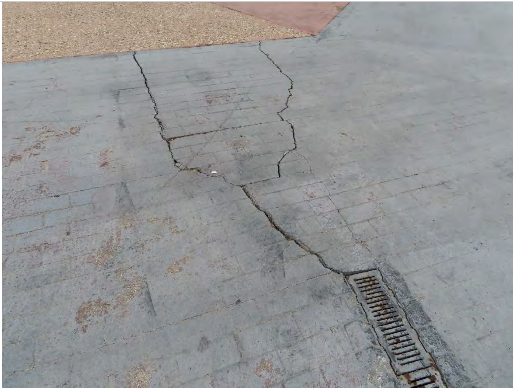
Photo 1.11- Typical spalled and cracked pavers, Village level (SH1-190)
