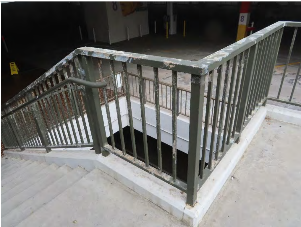
Photo 1.42- Corroded stair railing, (SH2-104)
