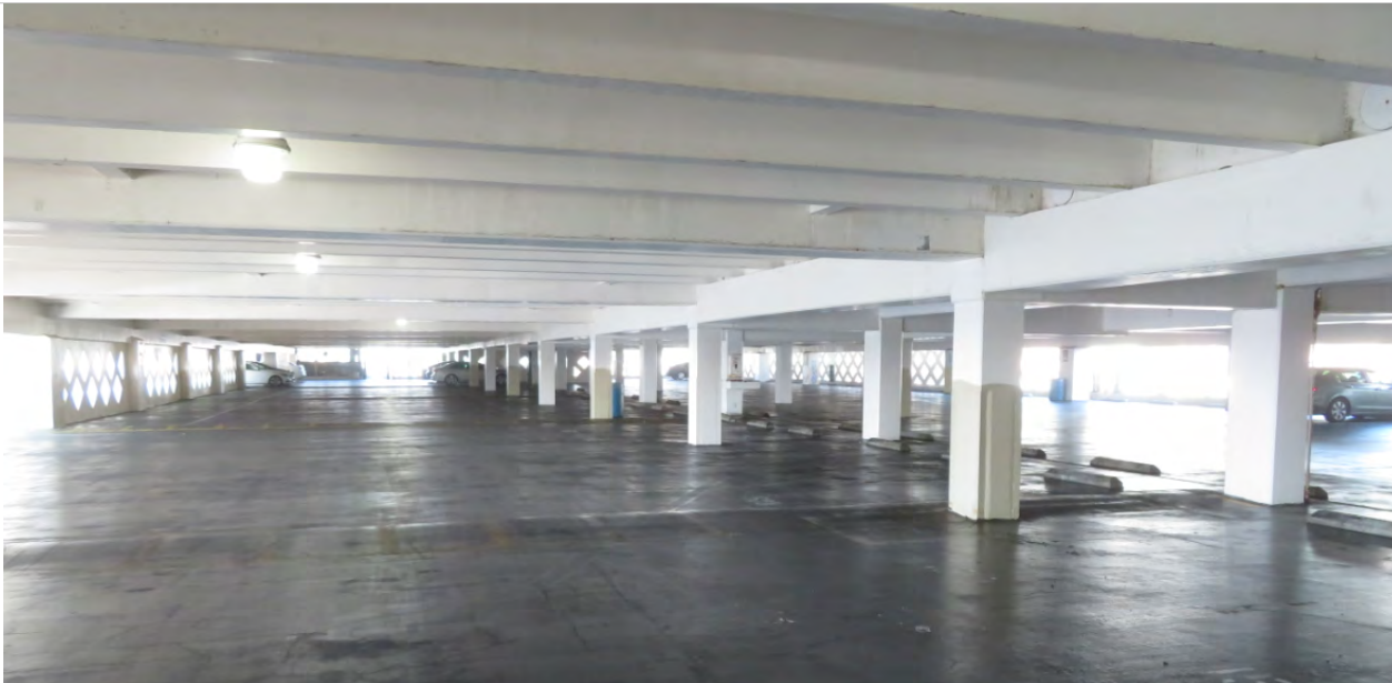
Photo 3.10—CIP Columns at Line X.7 and Y.3 at the Pier Level
