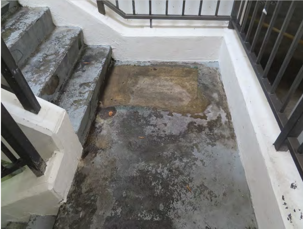
Photo 1.39- Typical stair coating worn off, (SH2-88)
