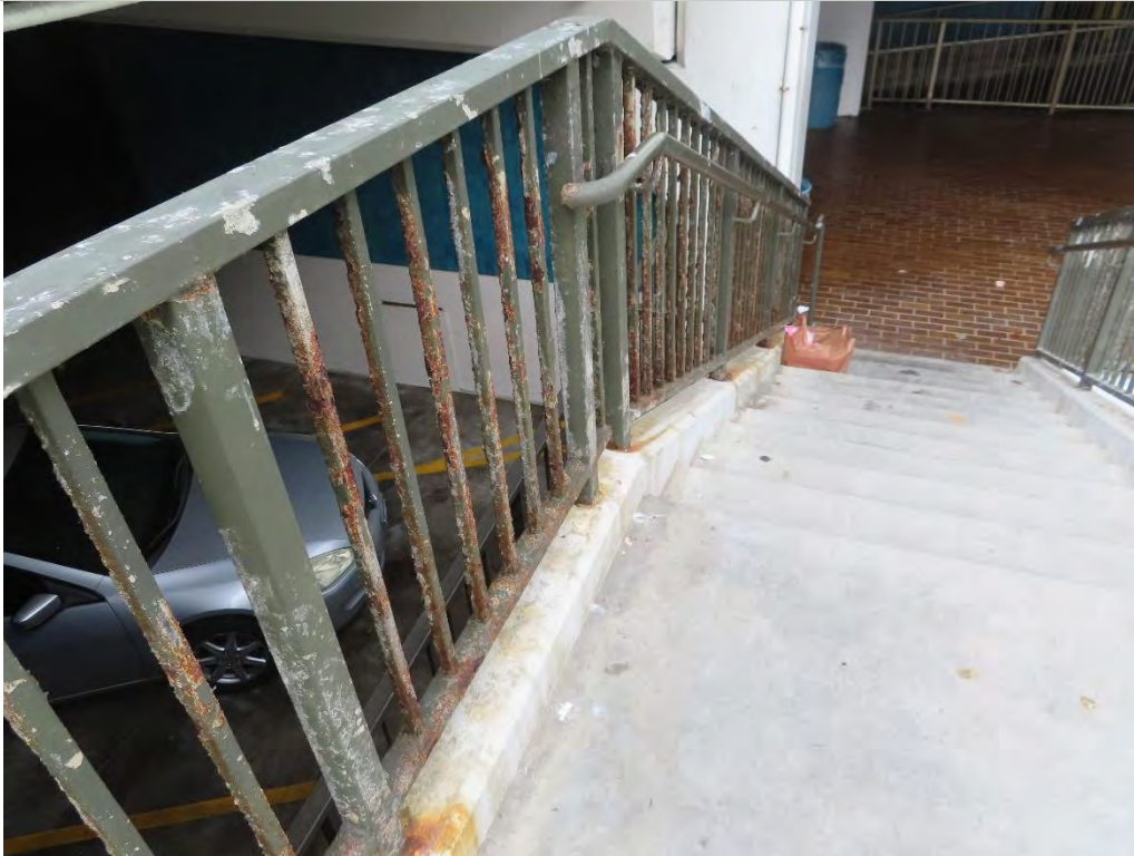
Photo 1.41- Corroded stair railing, (SH2-103)
