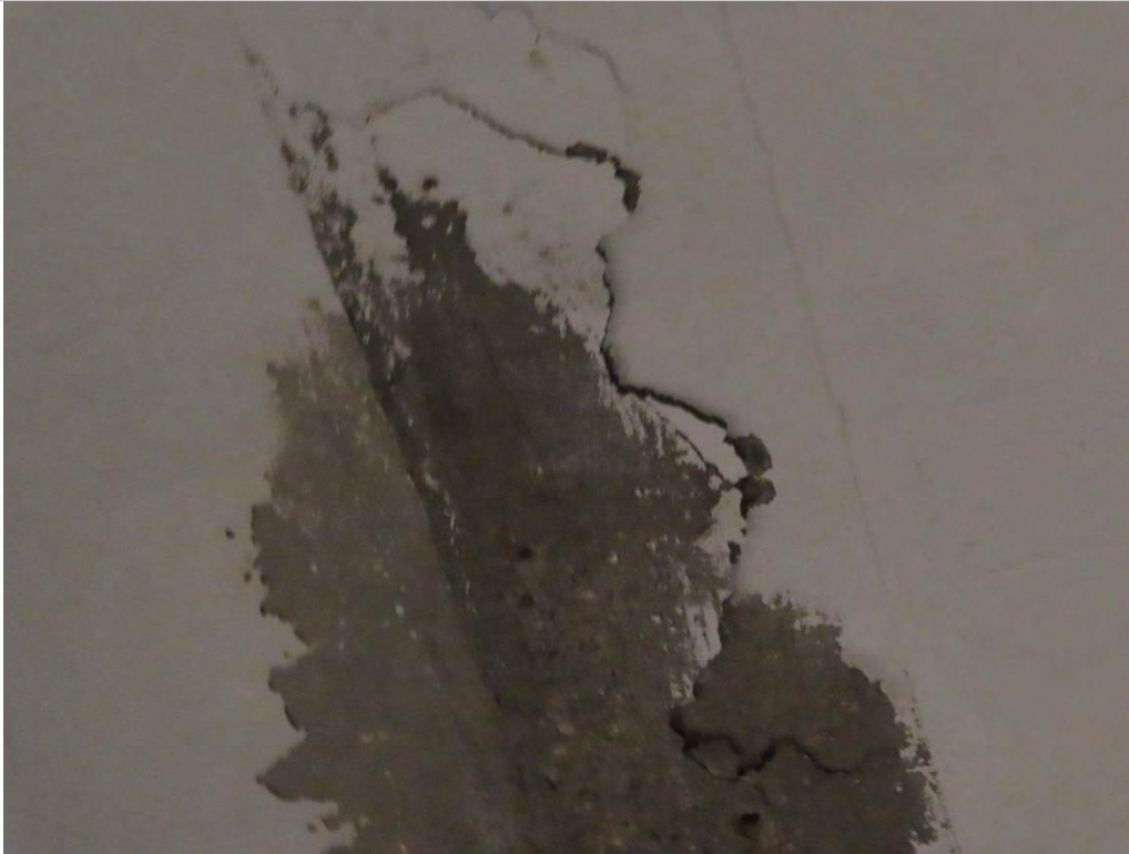
Photo 1.9- Concrete beam spalls with exposed reinforcement, Pier Level (SH3-31)
