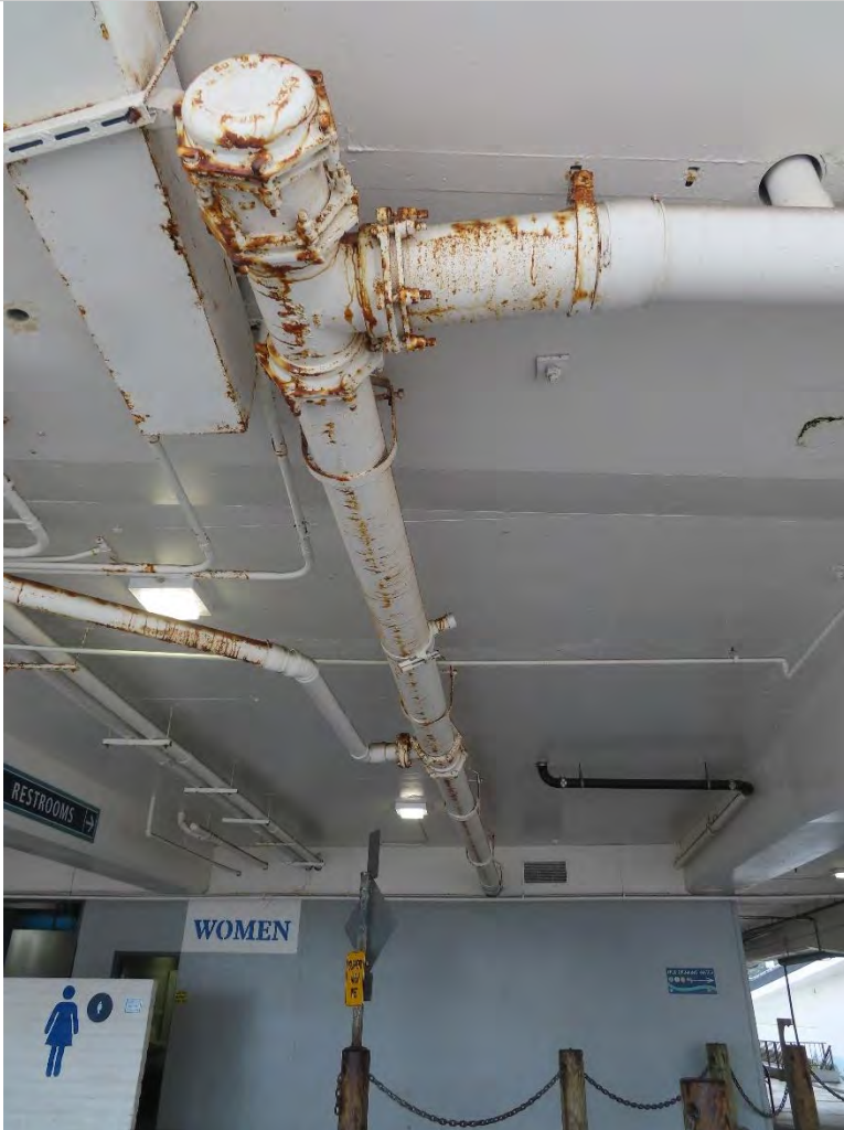
Photo 1.34- Corroded drainpipe, Pier level (MM1-33)
