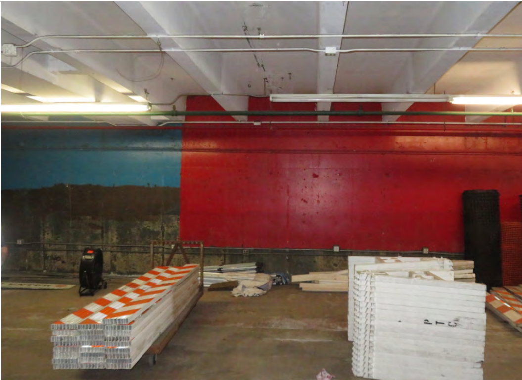
Photo 3.12- 8-inch-thick CIP Retaining Wall at line X and X.1 at Basement Level
