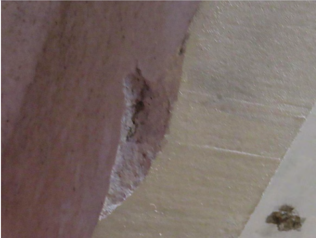
Photo 1.21- Concrete wall crack, Basement Level (SH3-256)
