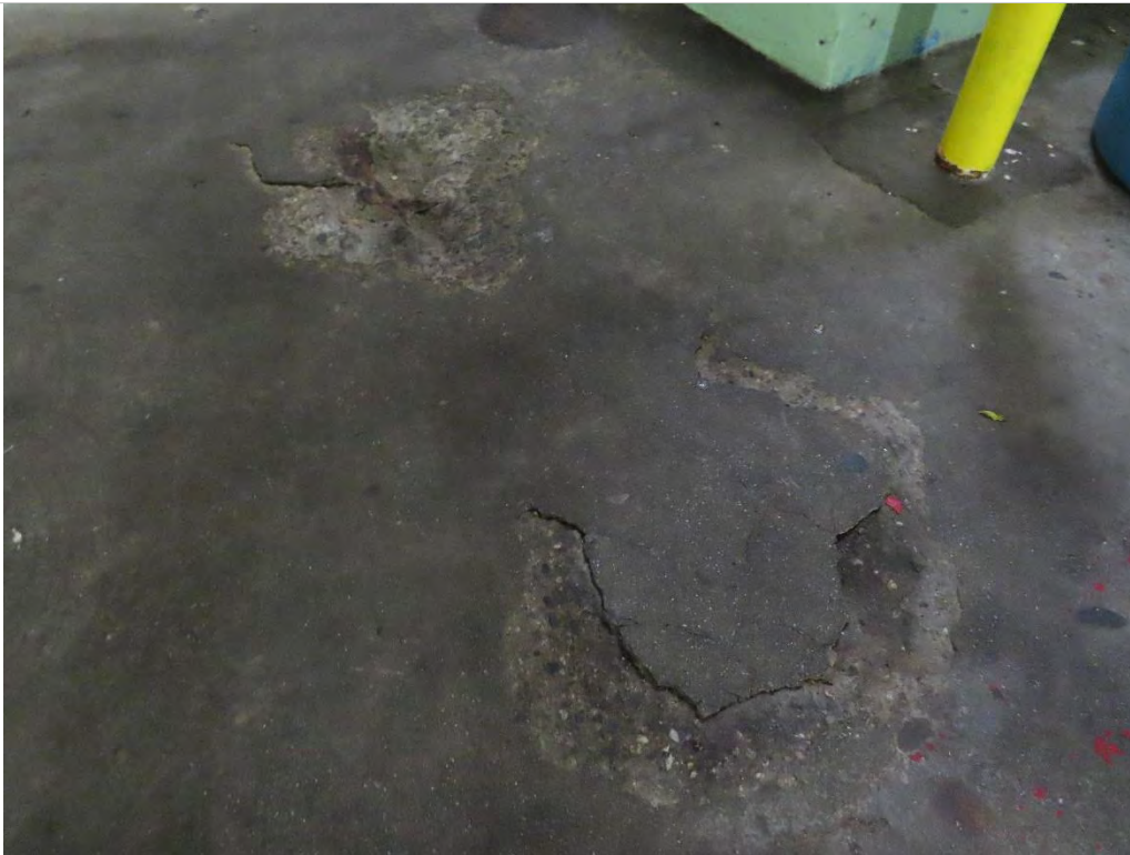
Photo 1.37- Deteriorated slab on grade, Basin level (SH2-48)
