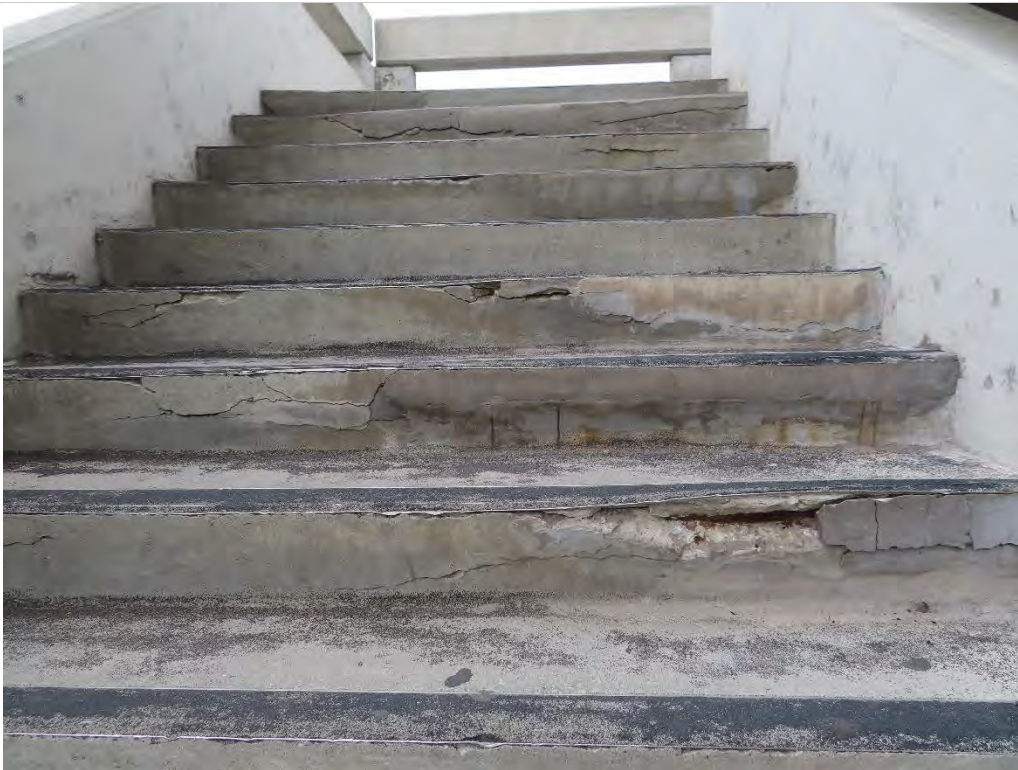
Photo 2.13- Damaged concrete stair treads and risers, (SH2-206)
