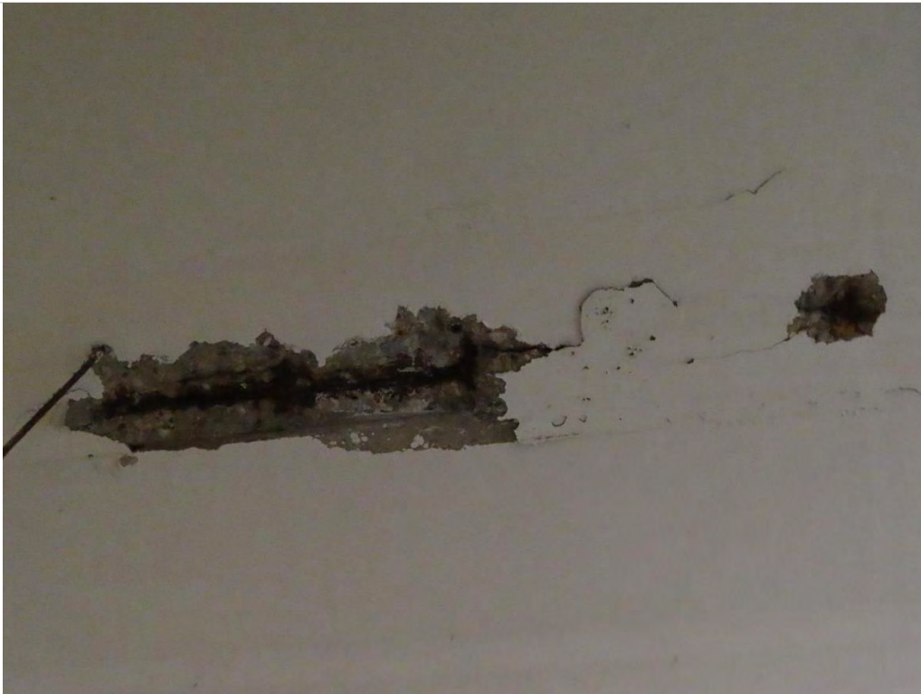
Photo 1.7- Soffit slab deterioration and spall with exposed reinforcement, Pier Level (SH3-312)
