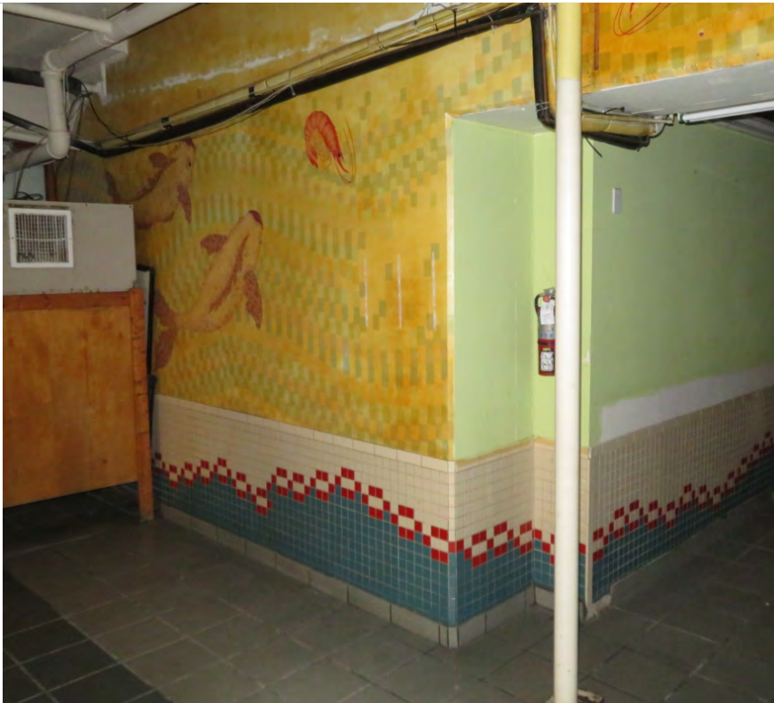
Photo 3.4- 24-inch-thick shear wall at line 3 and Y at Basement Level
