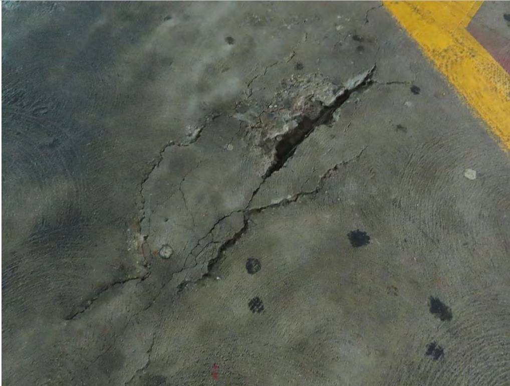
Photo 1.22- Isolated slab edge spall, Pier level (MM1-129)
