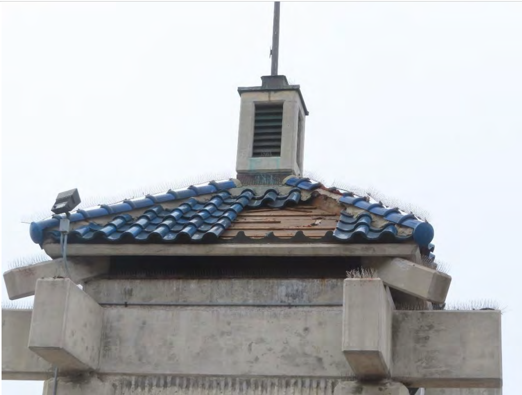
Photo 2.3- Missing roof tiles on the stair tower, Plaza level (SH2-130)
