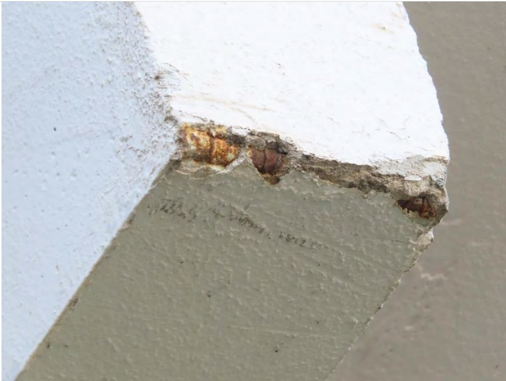
Photo 1.25- Concrete cantilever spandrel beam exposed rebar, Exterior – East elevation (SH2-372)
