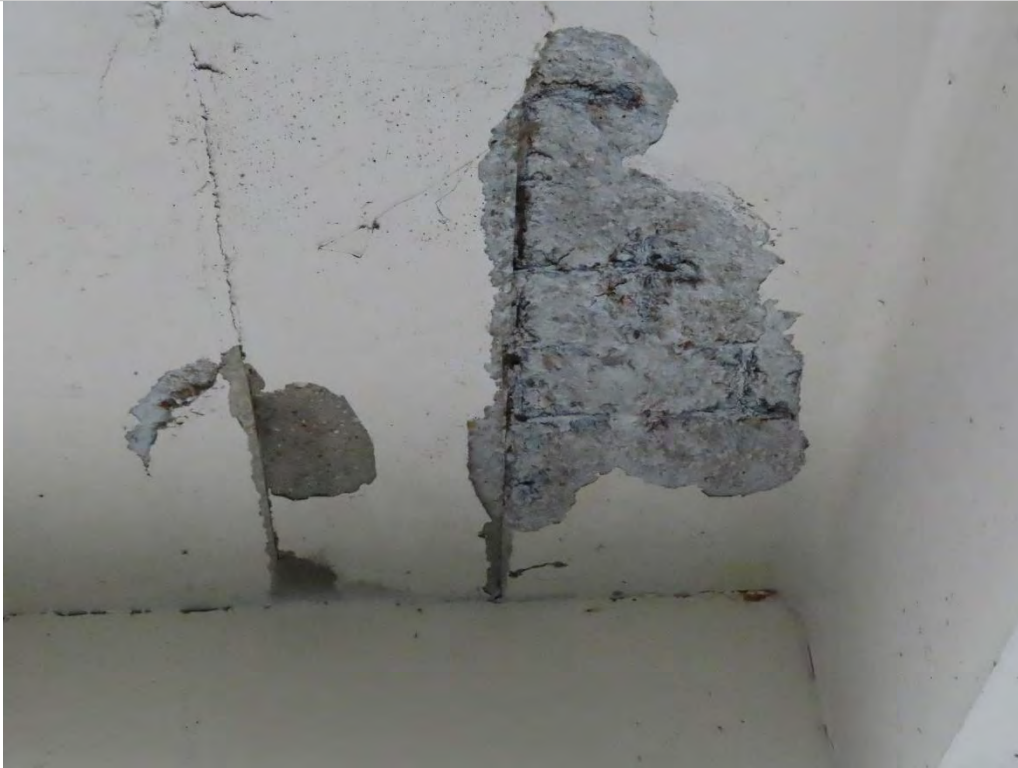
Photo 1.5- Concrete floor delamination, Pier Level (SH3-229)
