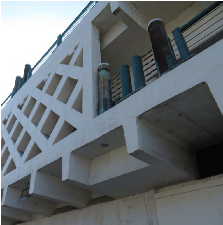
Photo 3.16- CIP Columns at shear wall ends at line Z at the Pier and Basement Level
