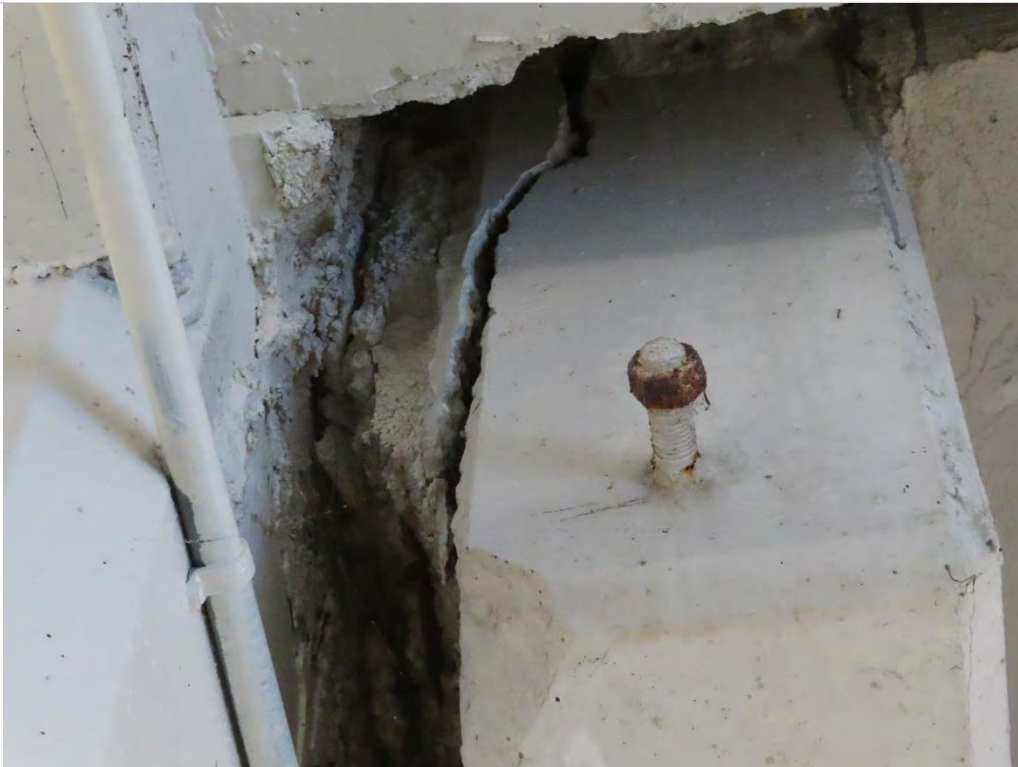
Photo 1.11- Concrete beam spall, Pier Level (SH3-197)
