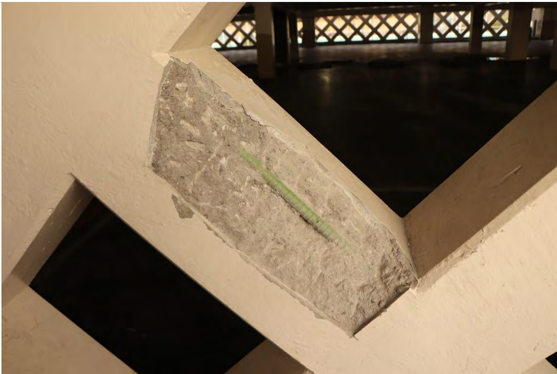
Photo 2.13- Opening of diagonal members on waffle wall, Only # 6 longitudinal bar was found, No confinement bar was present, 1992 Retrofit Wall on Gridline 3— Pier Level (BA2-178)
