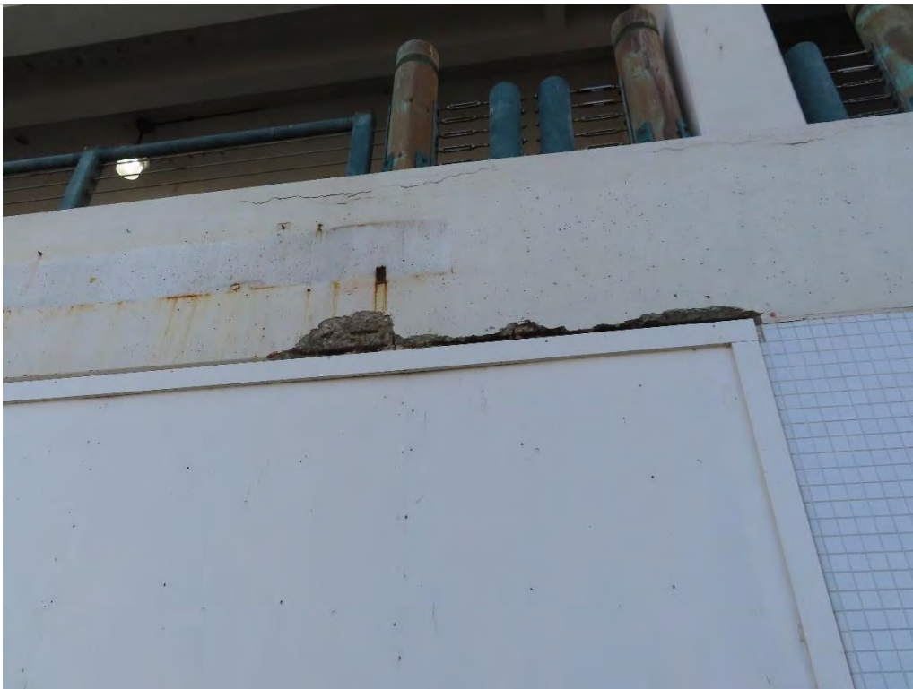
Photo 1.23- Concrete spandrel beam spall with exposed rebar, Exterior - North elevation (SH2-356)
