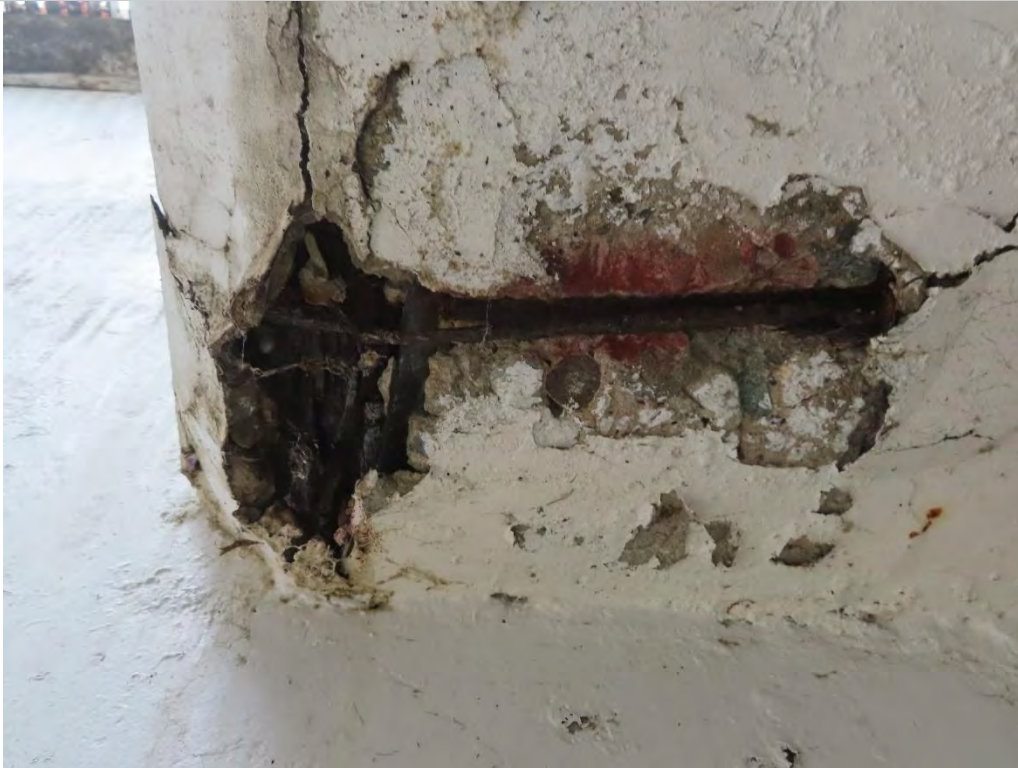
Photo 2.15- Damaged beam P/T rebar, Basin level (SH2-174)
