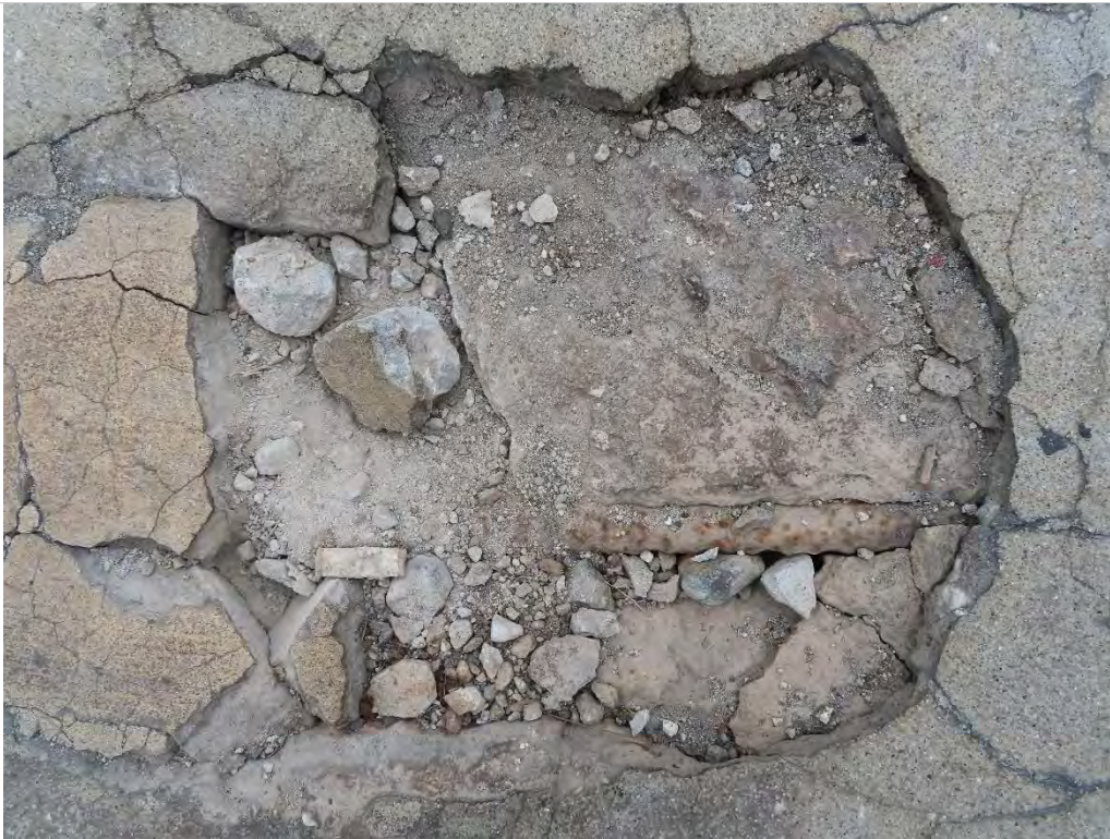
Photo 1.7- Exposed rebar on floor, Village level (SH1-180)
