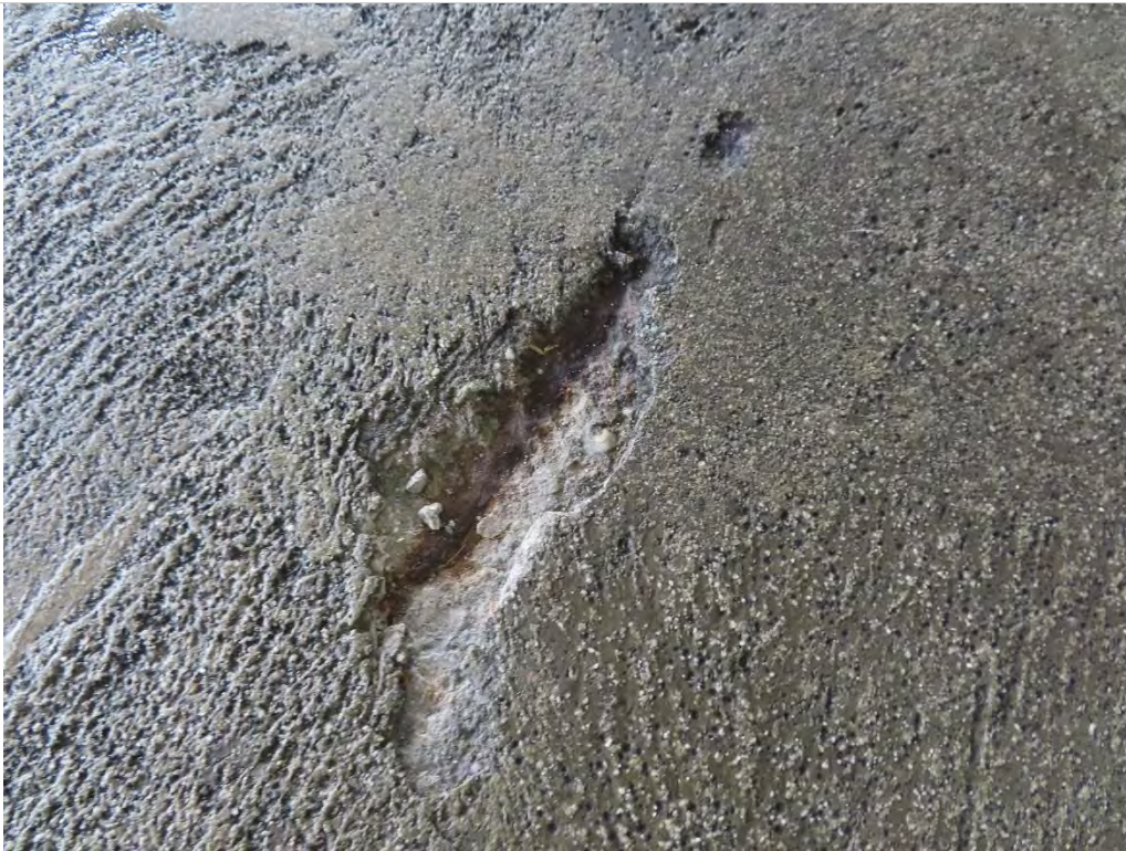
Photo 2.5- Exposed rebar on floor, Pier level (SH2-155)
