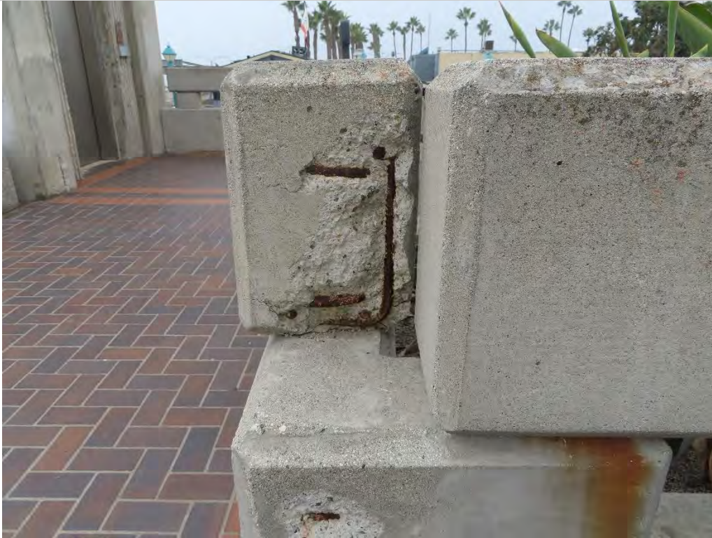
Photo 2.1- Spalled precast concrete spandrel with exposed rebar, Plaza level (SH2-265)
