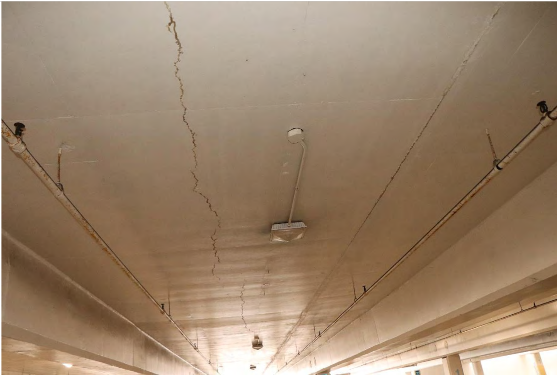
Photo 2.10- Concrete spalling underside the slabs, Pier level (SH2-185)
