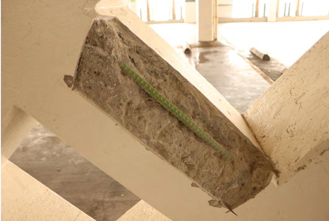
Photo 2.13- Opening of diagonal members on waffle wall, Only # 6 longitudinal bar was found, No confinement bar was present, 1992 Retrofit Wall on Gridline 3— Pier Level (BA2-178)
