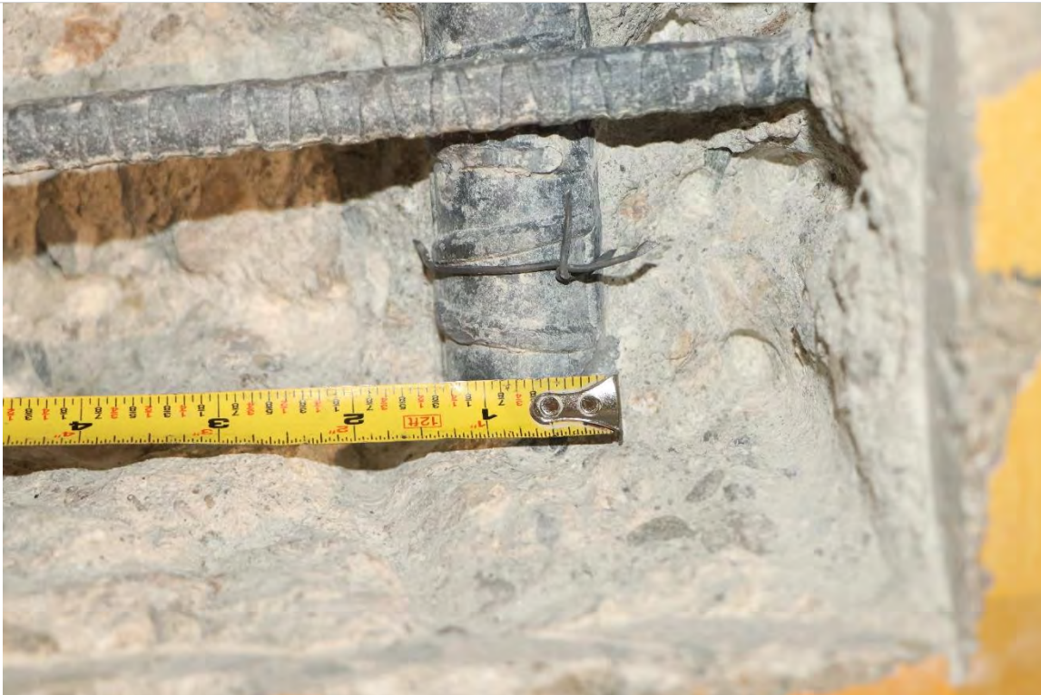
Photo 2.16— Vertical #10 bar found at wall jamb, destructive opening location DT4, Kitchen wall on gridline 3, 1962 Construction - Basement (BA2-580)
