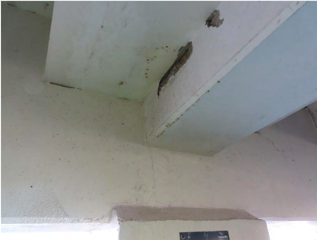
Photo 1.9- Concrete beam spalls with exposed reinforcement, Pier Level (SH3-31)
