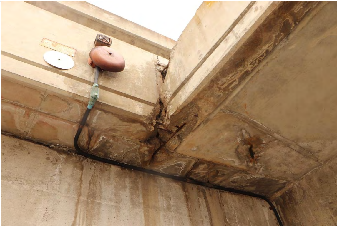
Photo 2.6- Soffit slab deterioration and spalls with exposed reinforcement, Pier level (BA1-326)
