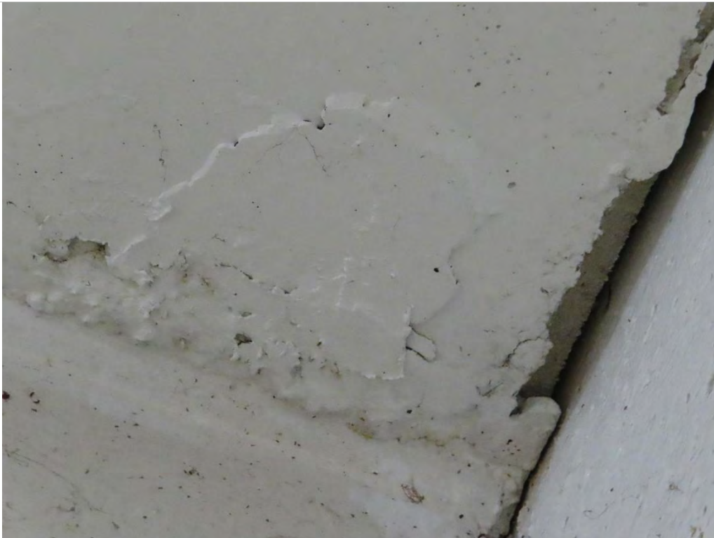
Photo 2.10- Concrete spalling underside the slabs, Pier level (SH2-185)
