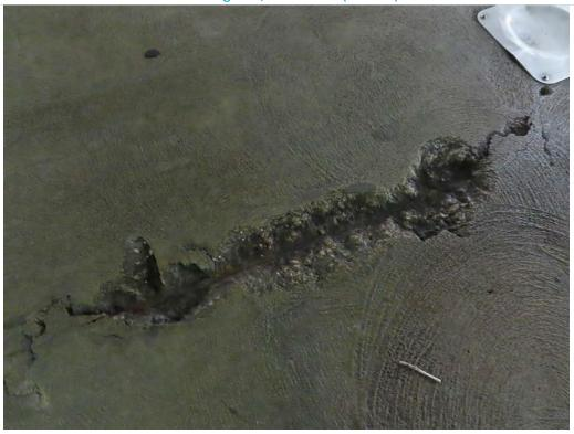
Photo 1.37- Deteriorated slab on grade, Basin level (SH2-48)
