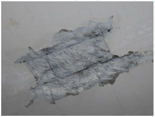
Photo 1.27- Soffit slab deterioration and spalls with exposed reinforcement, Pier level (SH2-58)
