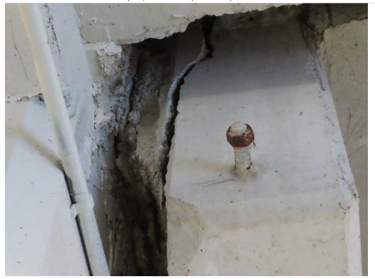
Photo 1.12- Concrete curb spall, Pier Level (SH3-35)
