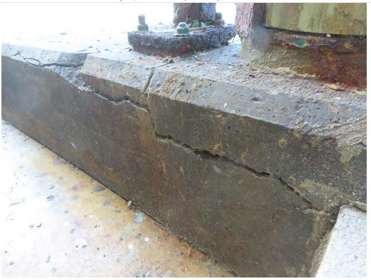
Photo 1.13- Concrete curb spall, Pier Level (SH3-189)
