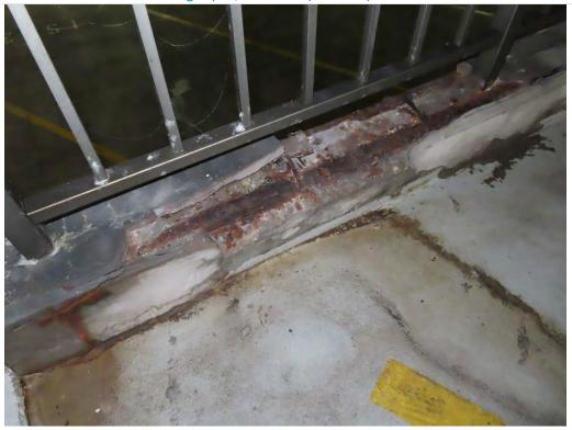
Photo 1.24- Exposed rebar on wall, Pier level (SH1-117)
