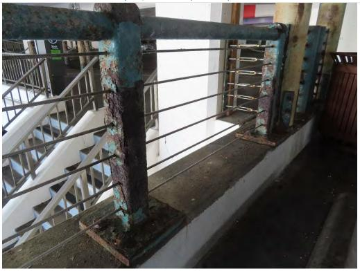
Photo 1.15- Compromised traffic coating, Pier Level (SH3-211)
