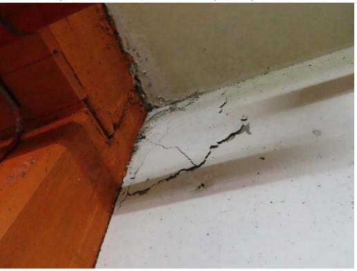
Photo 1.19- Concrete beam spall with exposed rebar, Basement level (SH3-303)
