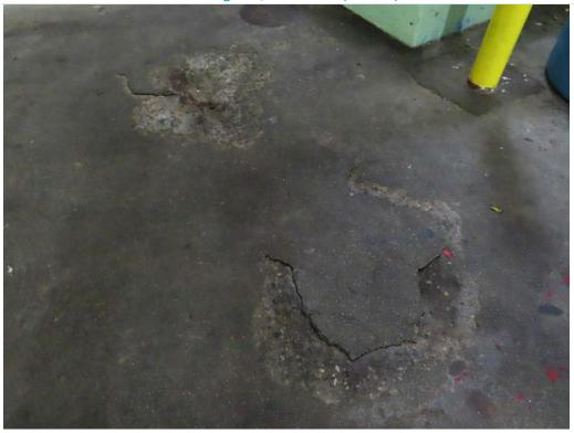
Photo 1.38- Isolated concrete column spalls, Basin level (SH1-241)
