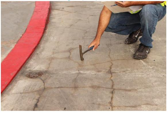
Photo 1.2- Concrete delamination, Village level (SH1-167)
