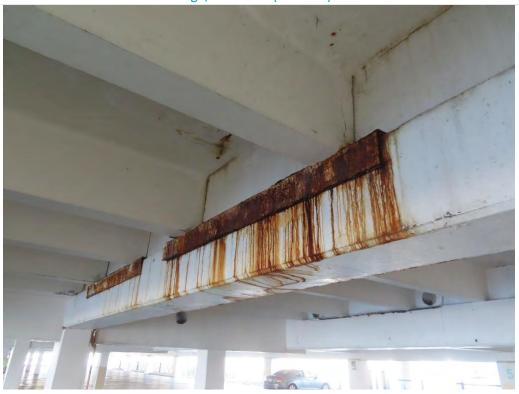
Photo 1.17- Exposed rebar on wall, Basement Level (SH3-308)
