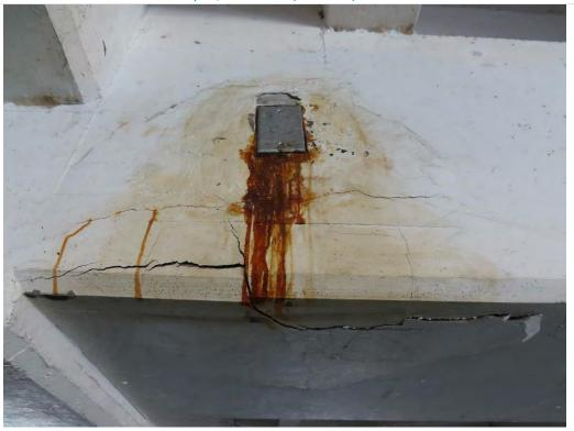
Photo 1.11- Concrete beam spall, Pier Level (SH3-197)
