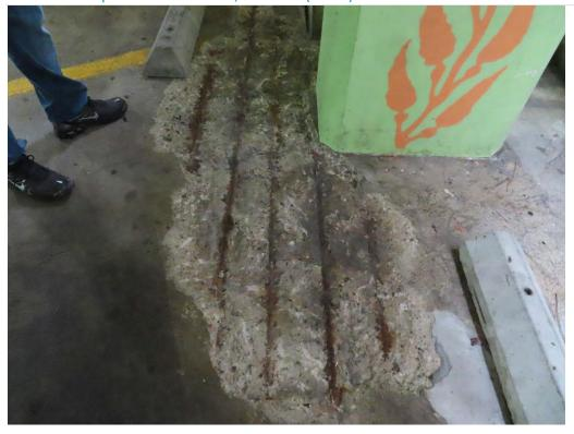
Photo 1.20- Exposed rebar on floor, Pier level (SH2-17)
