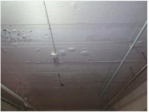
Photo 1.16- Deteriorated fiber reinforcing wrap, Village level (SH1-96)
