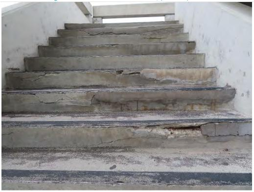
Photo 2.14- Damaged concrete stair treads and risers, (SH2-209)
