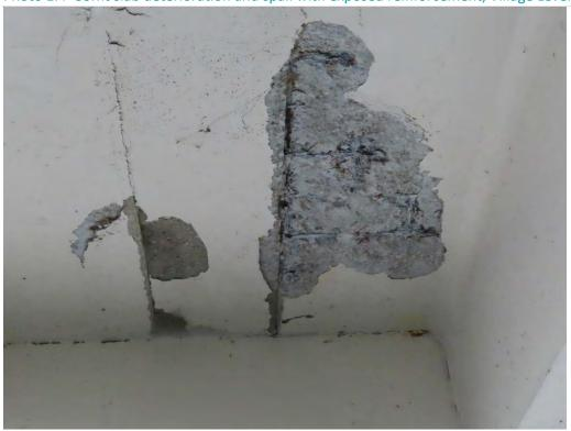
Photo 1.5- Concrete floor delamination, Pier Level (SH3-229)
