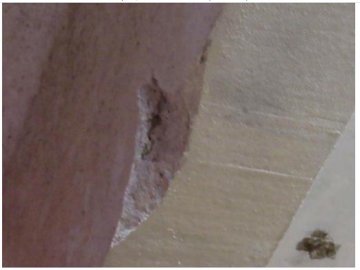
Photo 1.21- Concrete wall crack, Basement Level (SH3-256)
