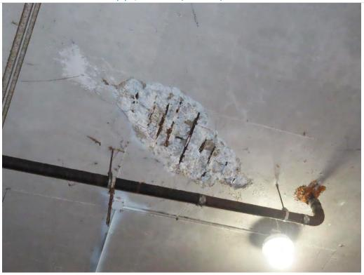
Photo 1.36- Deteriorated slab on grade, Basin level (SH2-44)
