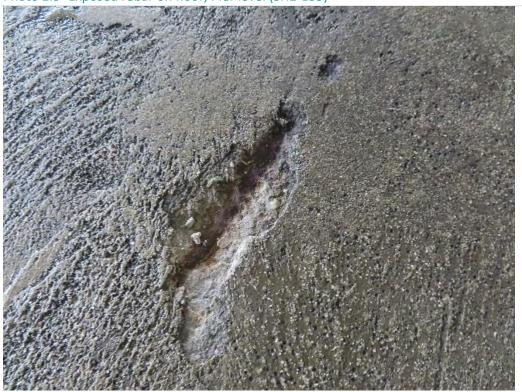
Photo 2.6- Soffit slab deterioration and spalls with exposed reinforcement, Pier level (BA1-326)
