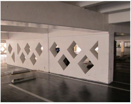
Photo 3.6- 12-inch-thick waffle shear wall along line X at Pier Level
